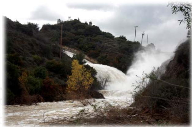
Santiago Creek Dam Spillway December 2010
