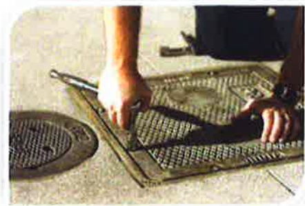
Grease Interceptor is Opened for Inspection
