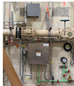
Wall mounted electric tankless water heater.
