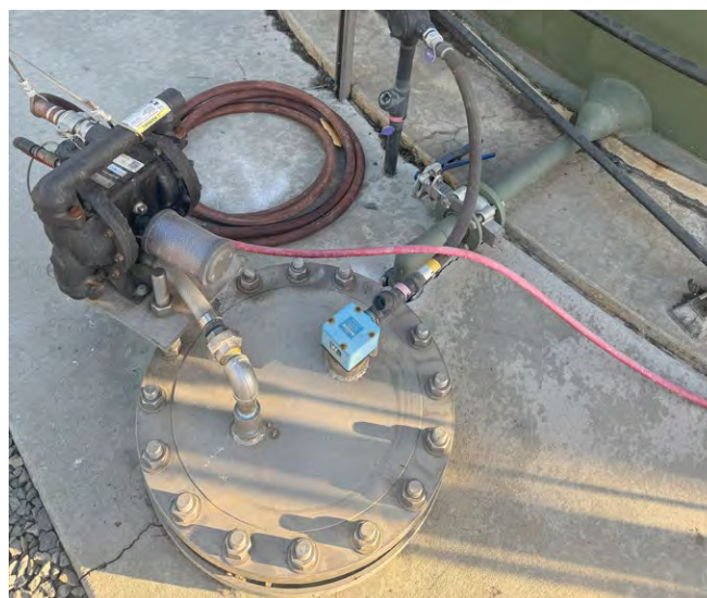
Existing Condensate Trap at Gas Holder with Temporary Pumping Setup.
