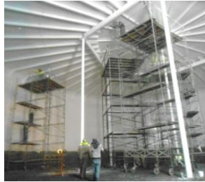
Interior Coating Assessment
