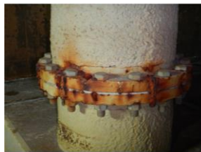
At-grade Test Station
