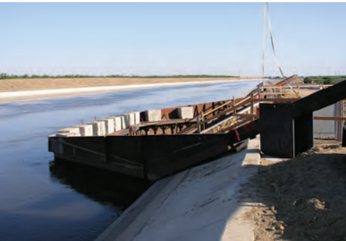
Semitropic Water Storage District Stored Water Recovery Unit
