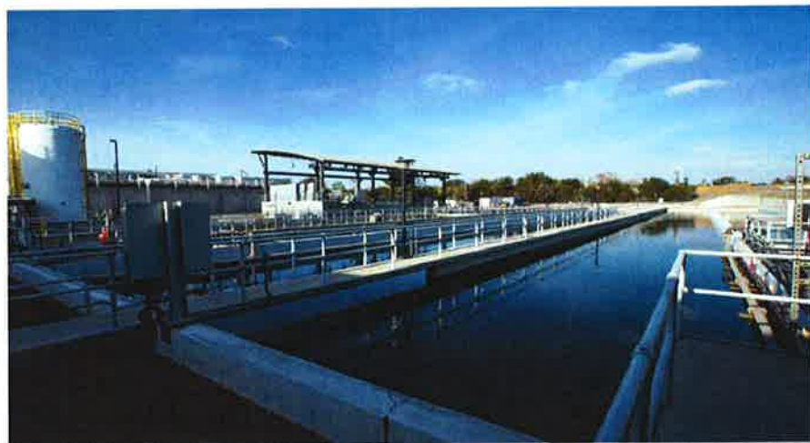
Michelson Water Recycling Plant
