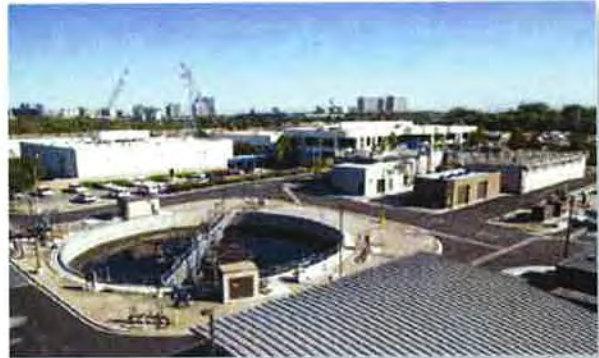
Michelson Water Recycling Plant
