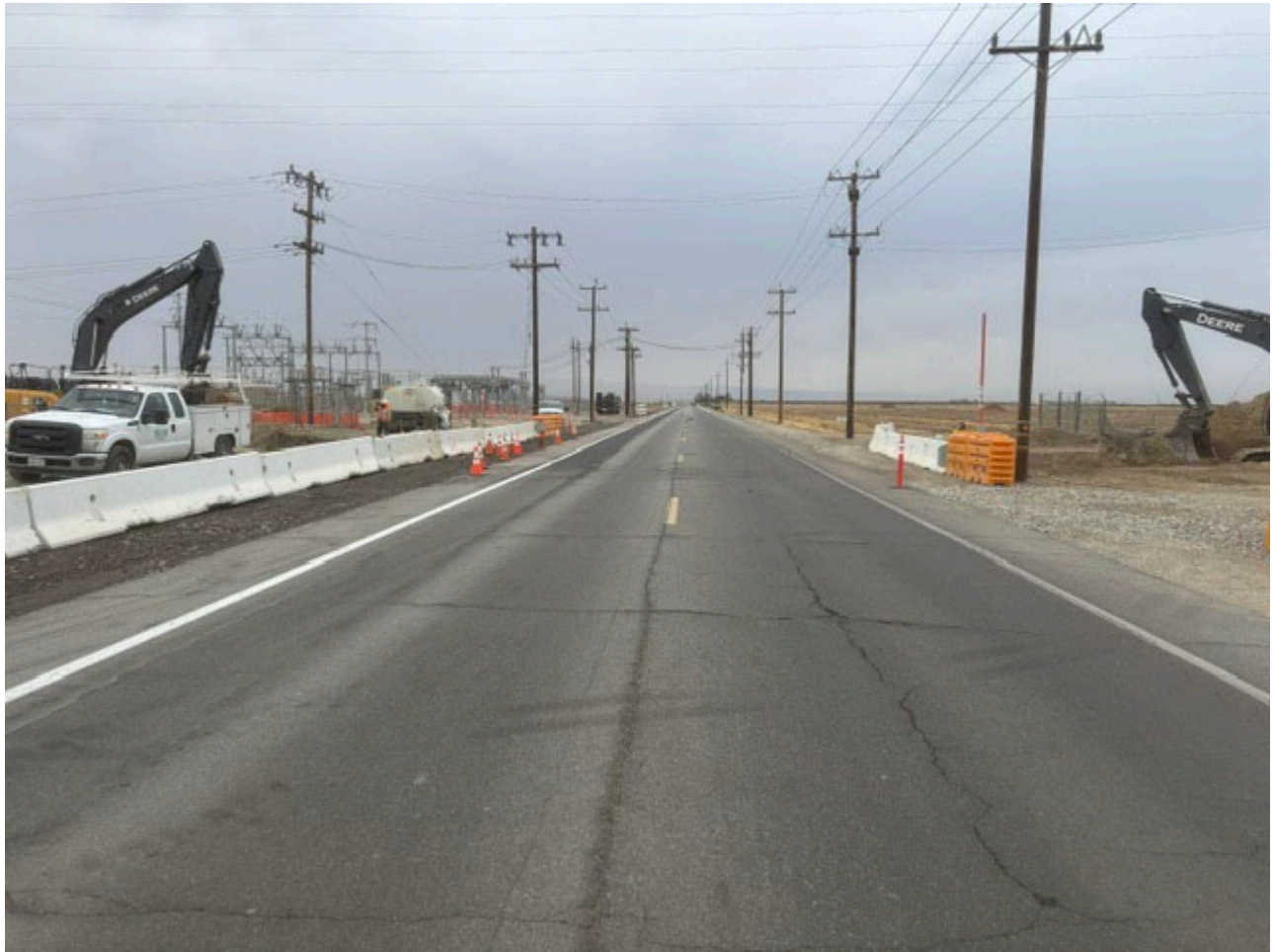
Installation of K-Rail and Crash Barriers
