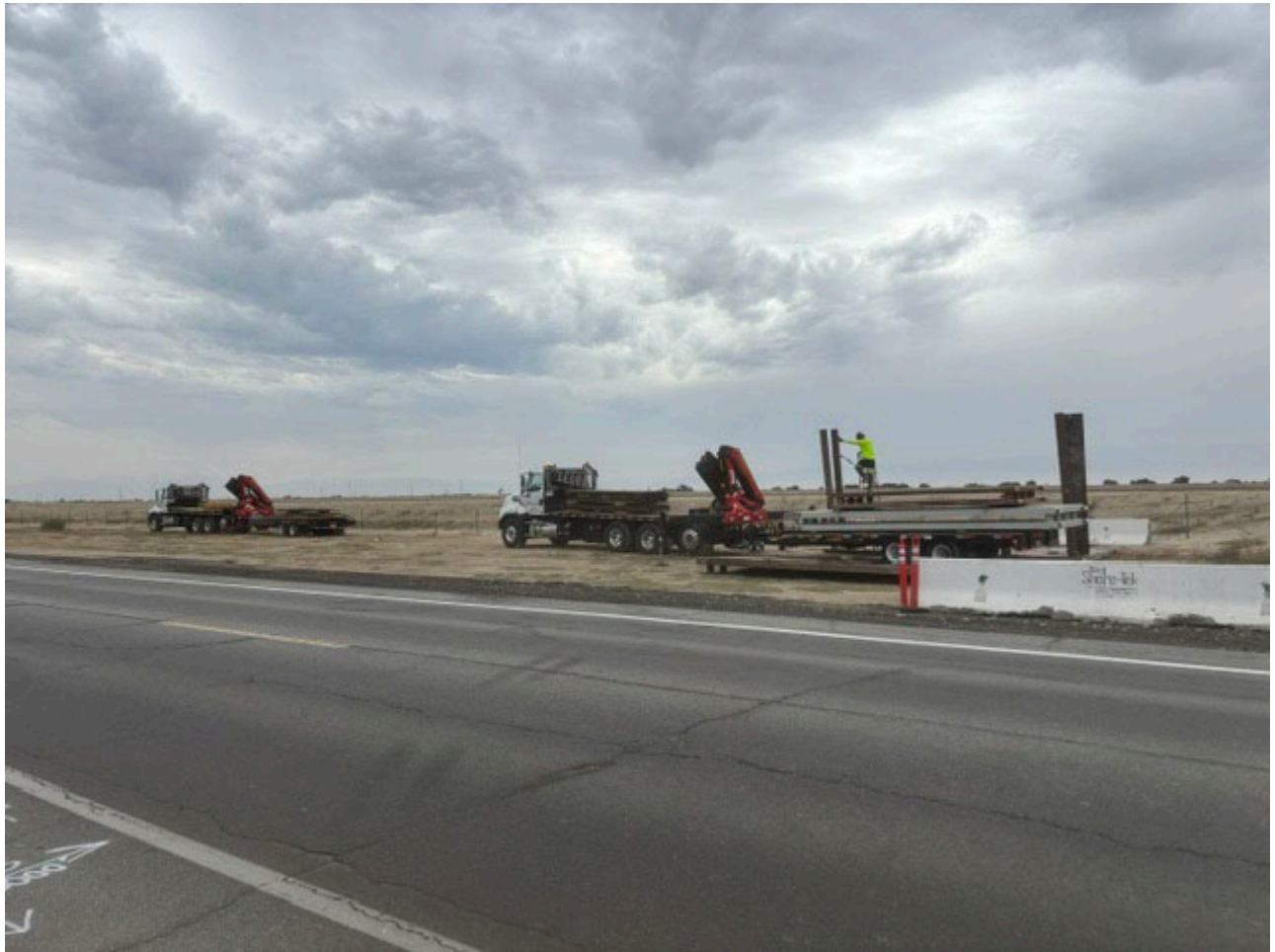
Delivery of Shoring Materials
