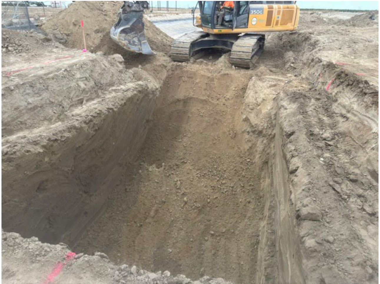
Excavation on North Side of Stockdale Hwy for Cased Crossing
