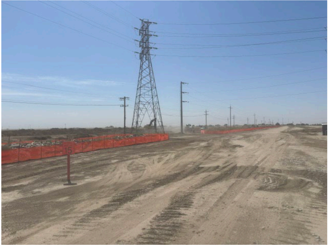
Bio Fencing Installed around Broken Concrete Stockpile
