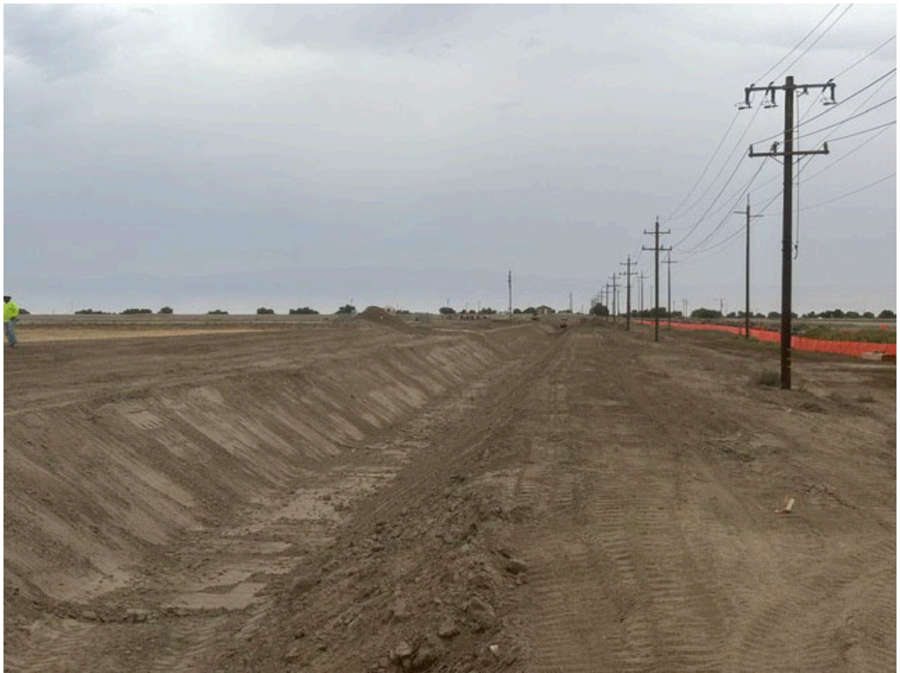
Channel Fine Grading
