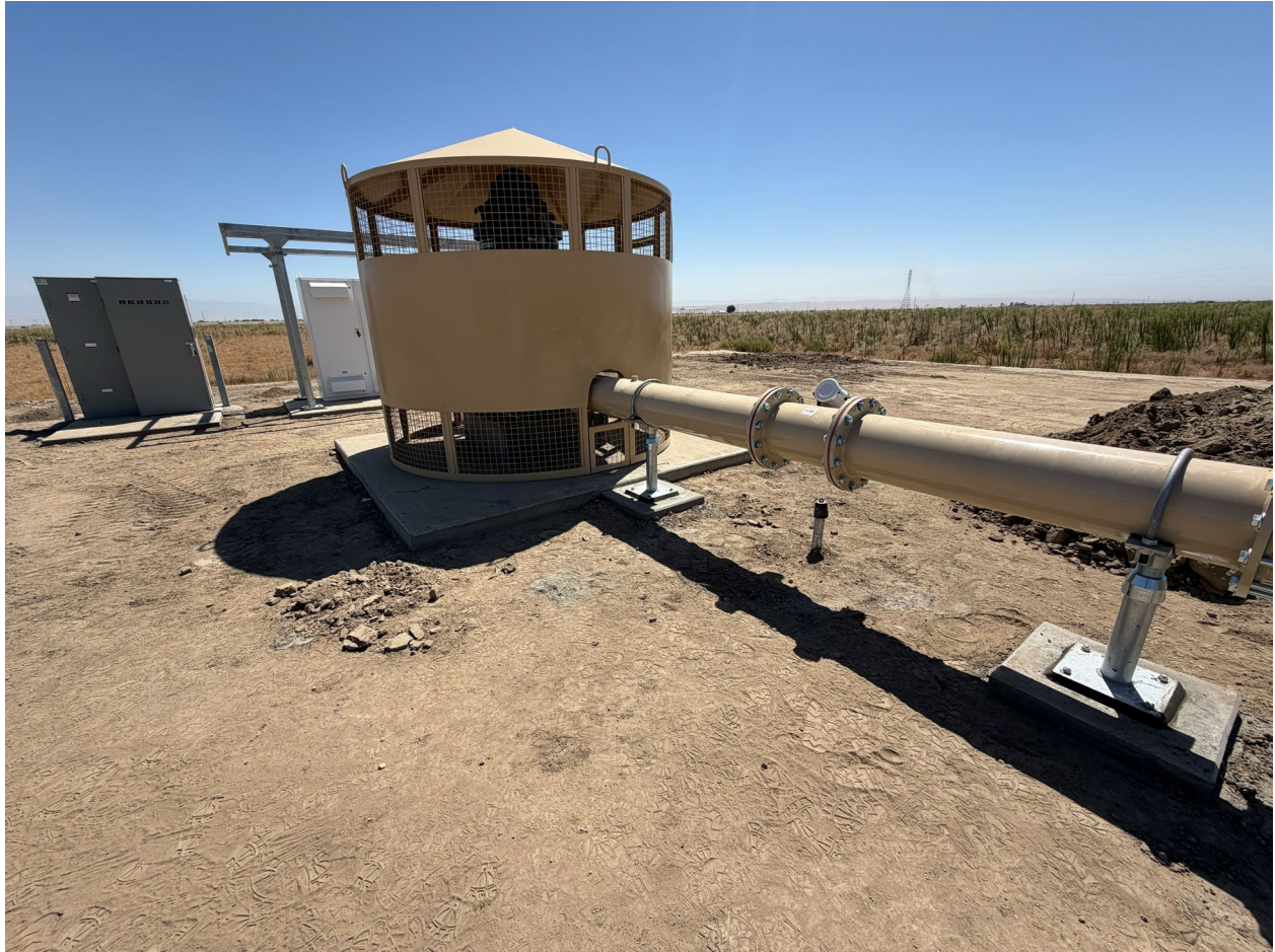
SN-1: Discharge Piping Installation
