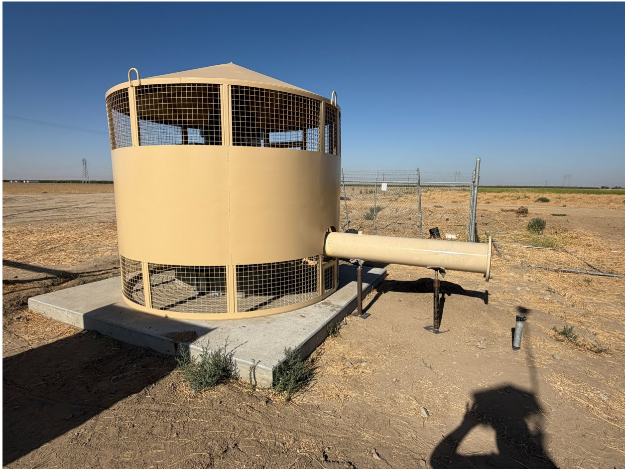
Existing Ag Well: Pump, Motor, Enclosure, and Piping Installation
