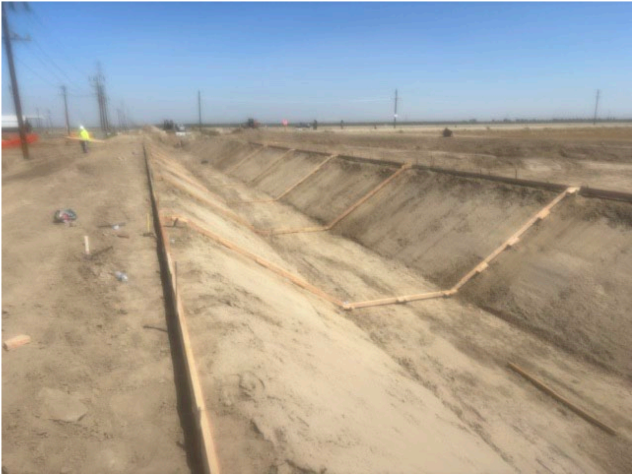
Formwork for Concrete Lining
