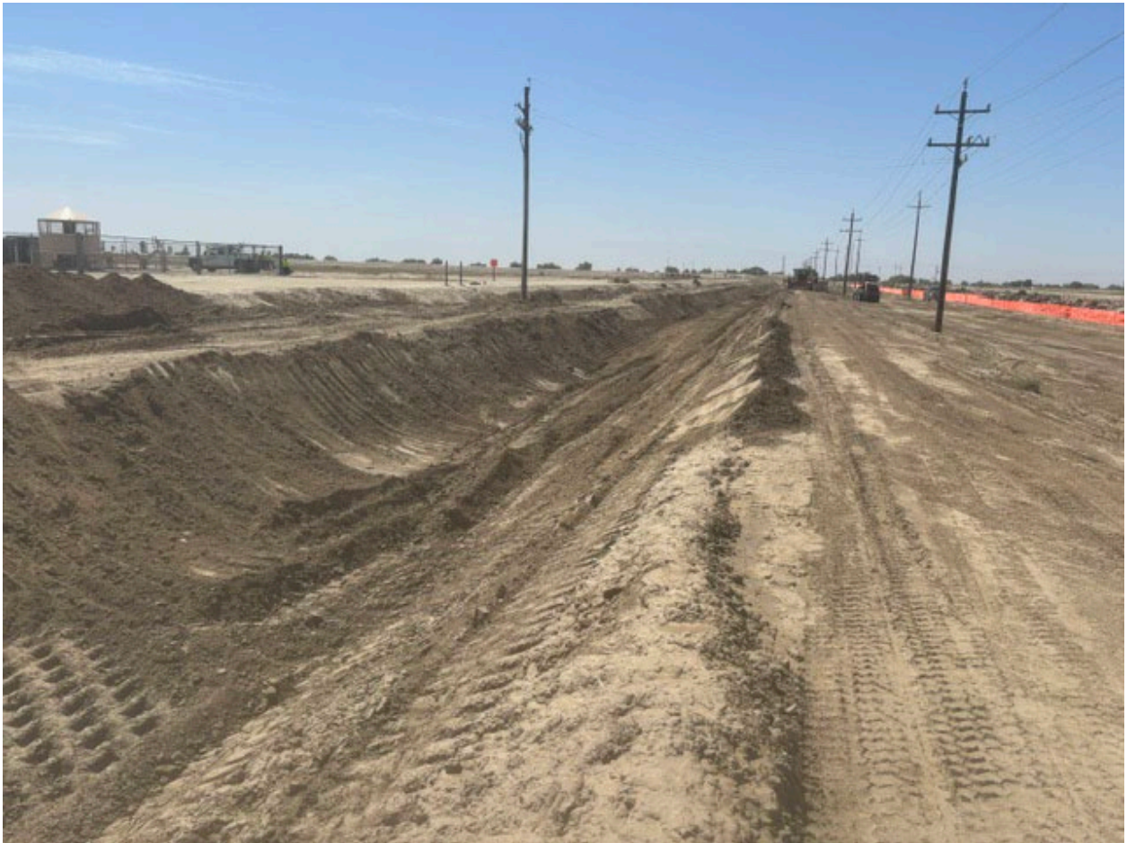
Concrete Liner Removal
