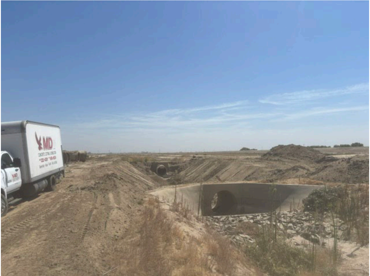
Removal of Existing 72" RCP Siphon at Pioneer Canal
