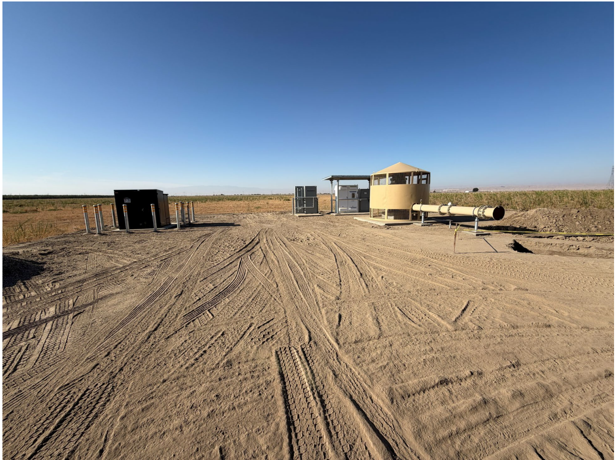
SN-1: Site with PG&E Transformer and Service Installed
