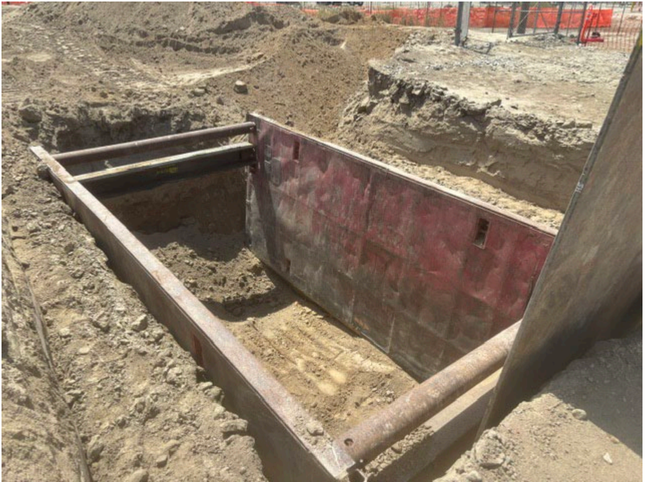
Shoring on South Side of Stockdale Hwy
