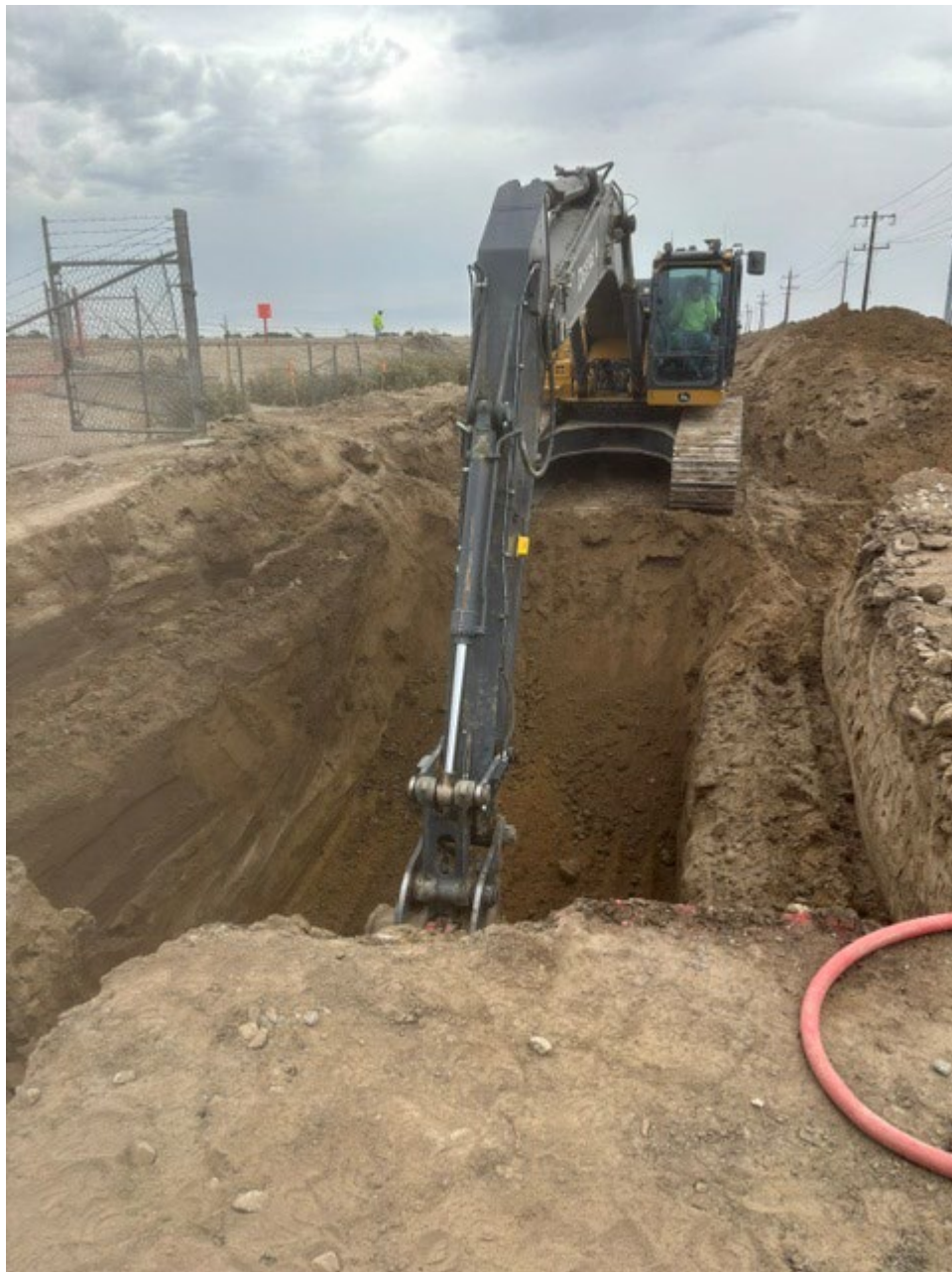
Excavation on South Side of Stockdale Hwy for Cased Crossing
