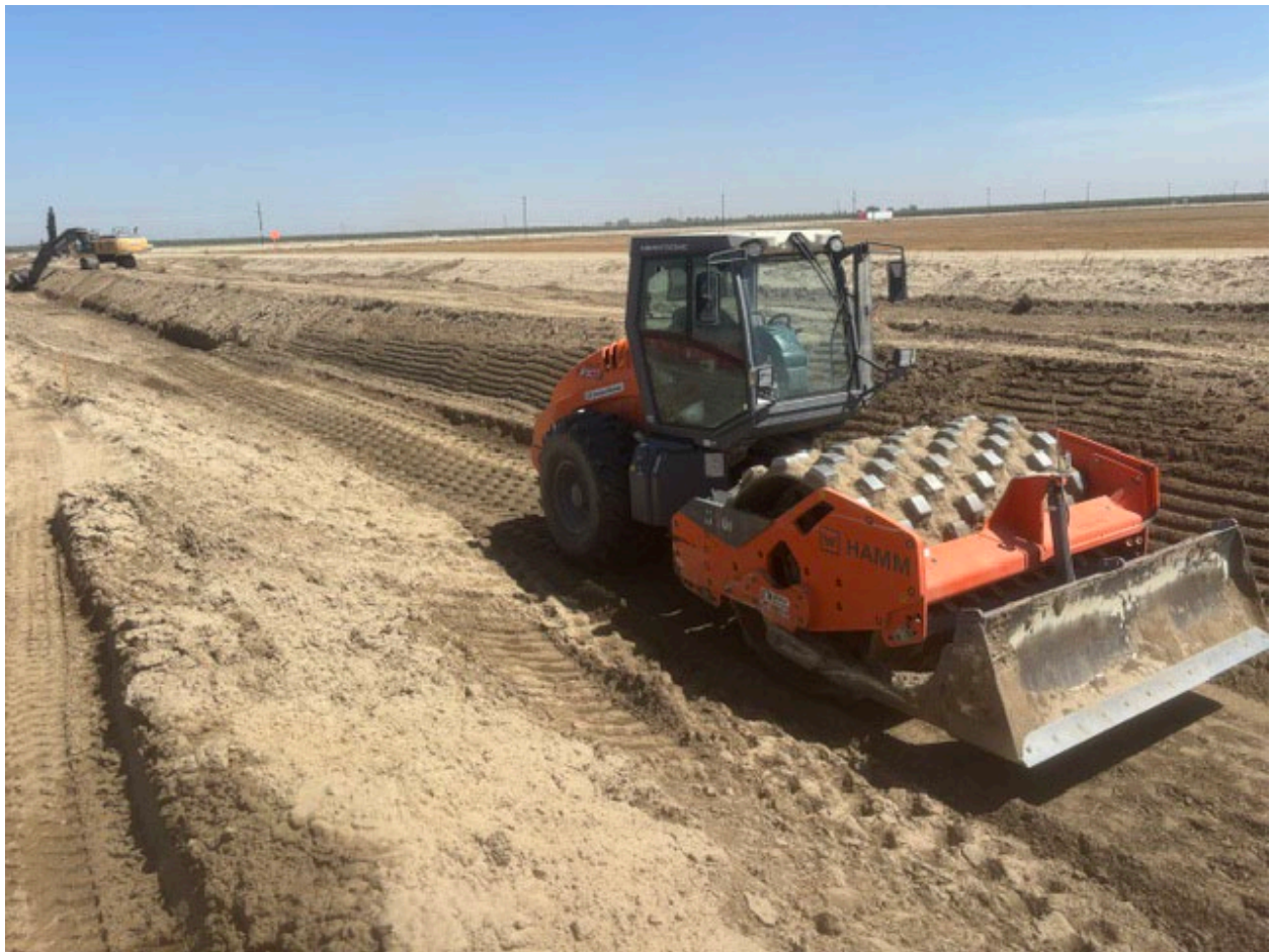
Channel Earthwork and Compaction
