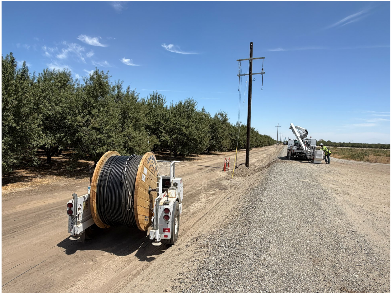
SN-1: PG&E Service Installation
