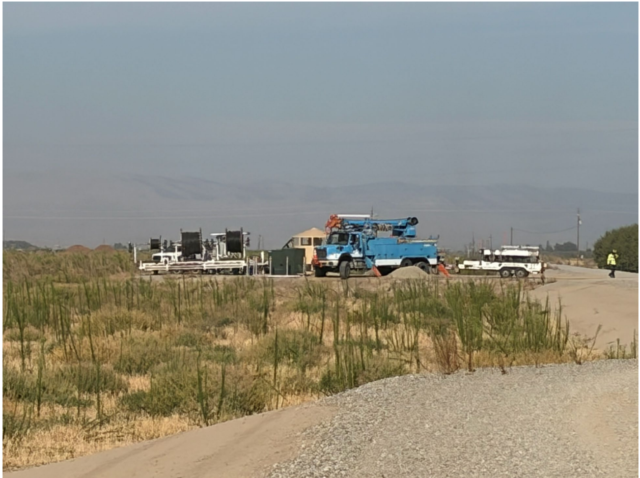
SN-1: PG&E Service Installation
