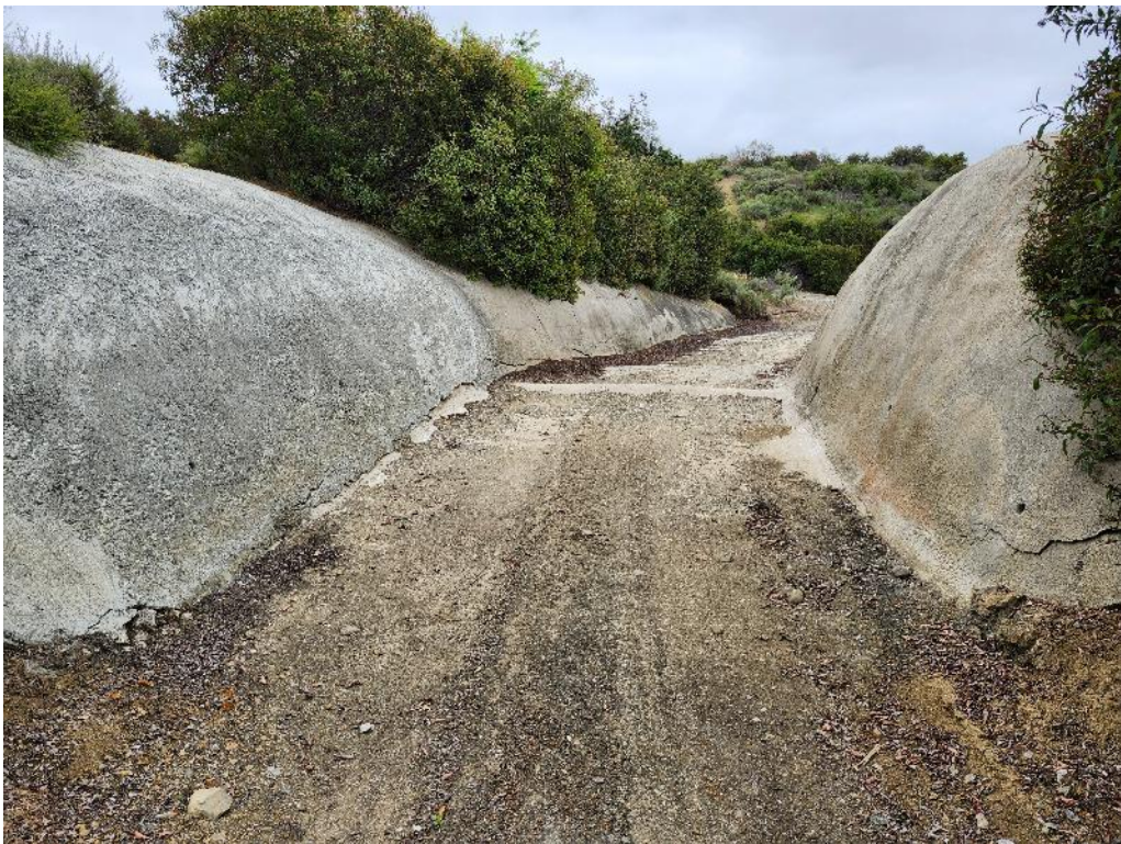
Photo 4. Downstream channel of the spillway.
