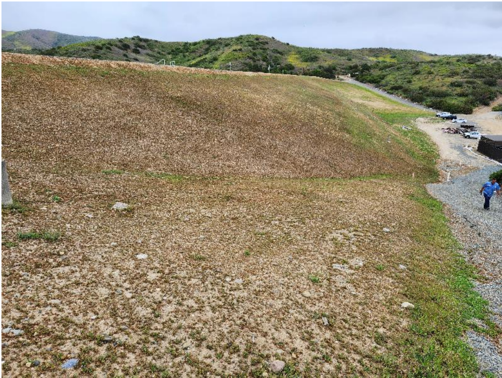
Photo 2. Downstream slope of the dam.
