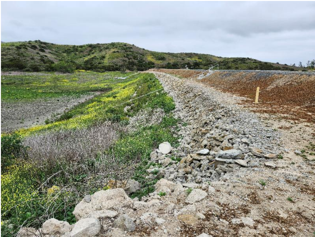
Photo 1. Upstream slope of the dam.
