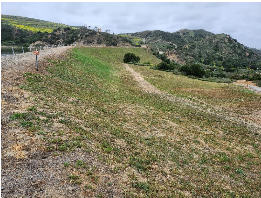
Photo 2. Downstream slope of the dam.
