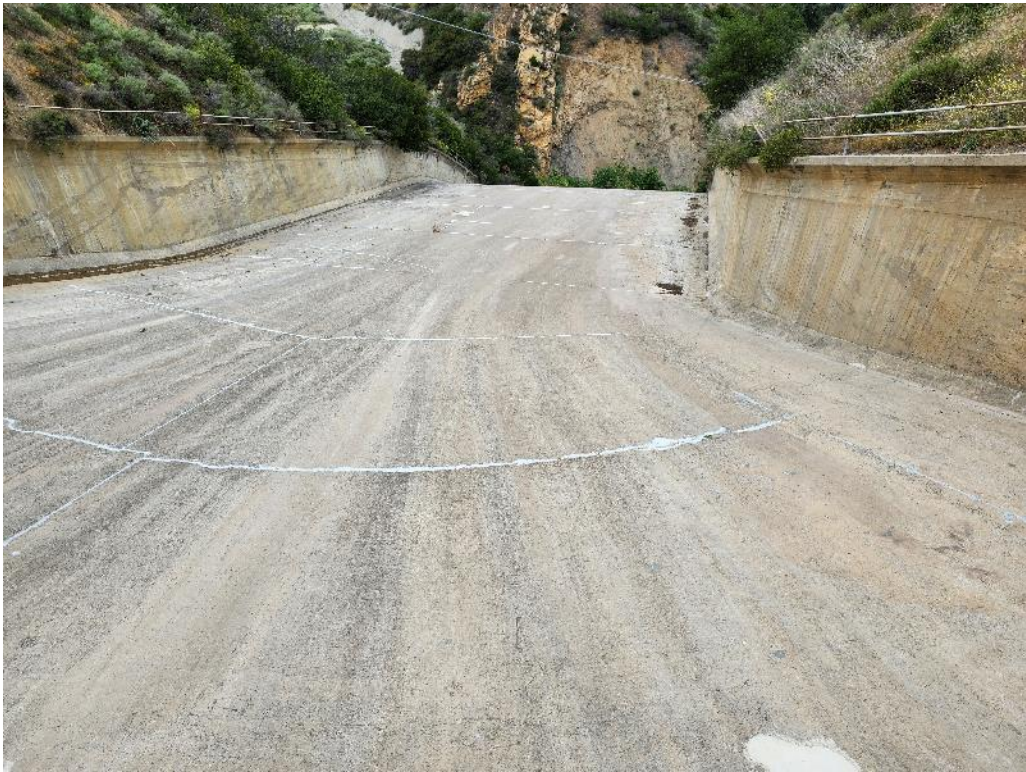
Photo 5. Spillway downstream chute.
