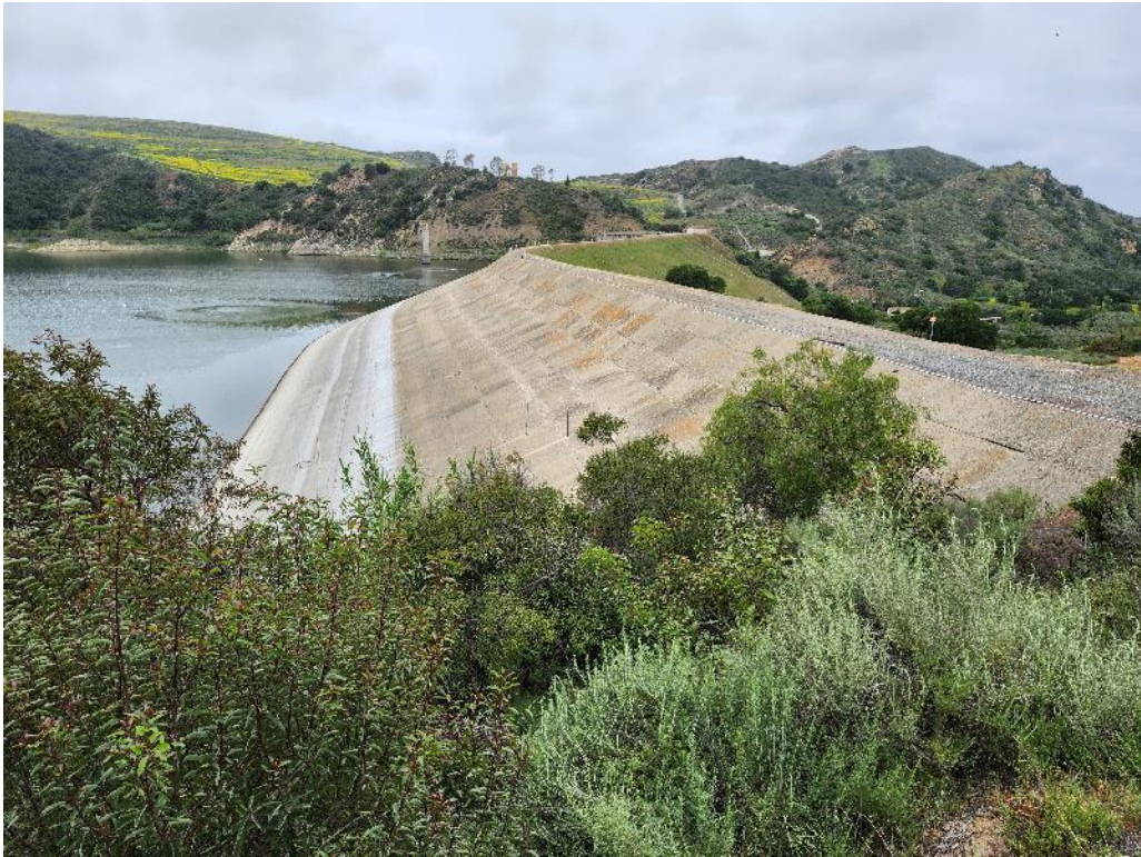
Photo 1. Upstream slope of the dam.
