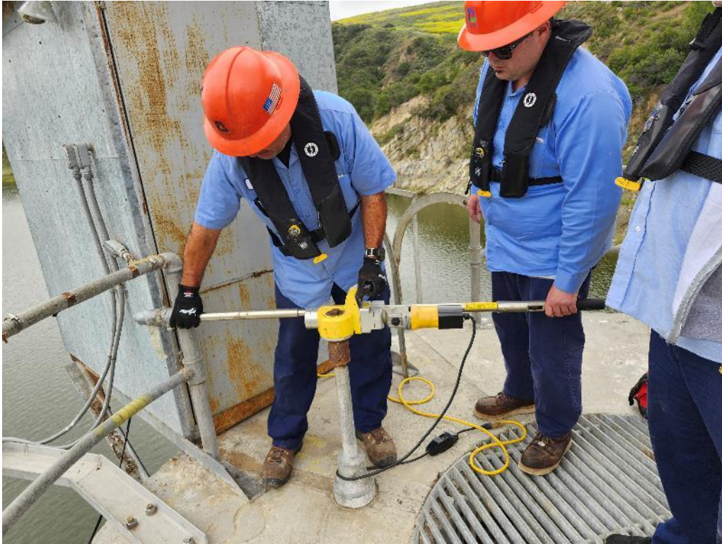
Photo 7. Cycling the upstream slide gates.
