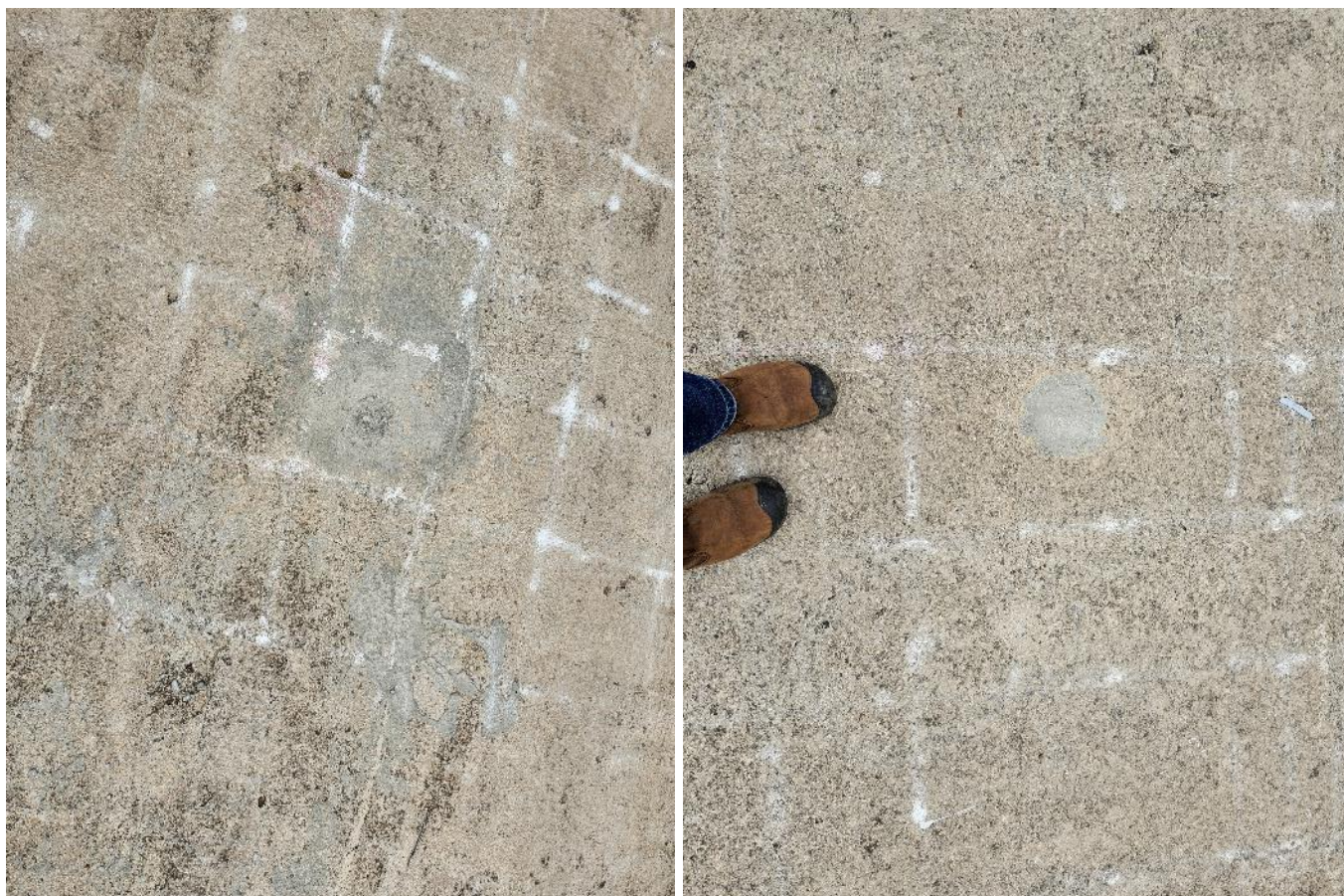
Photo 6. Examples of corings in the spillway satisfactorily backfilled.
