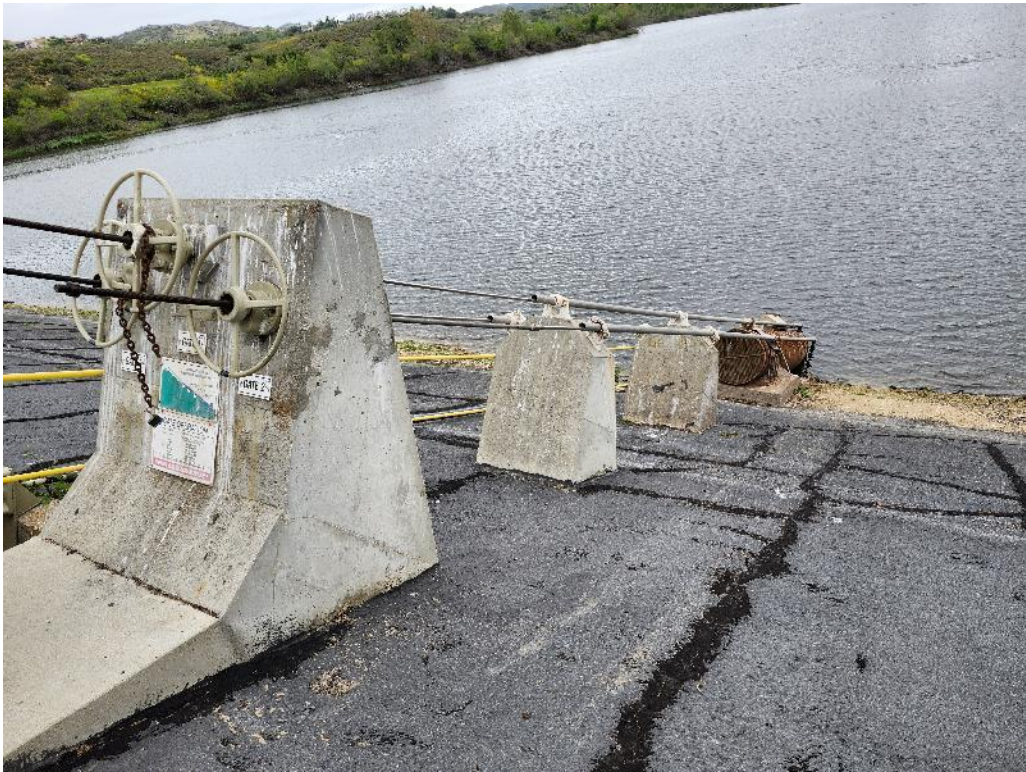
Photo 6. Slide Gate #2 bent stem has been repaired.
