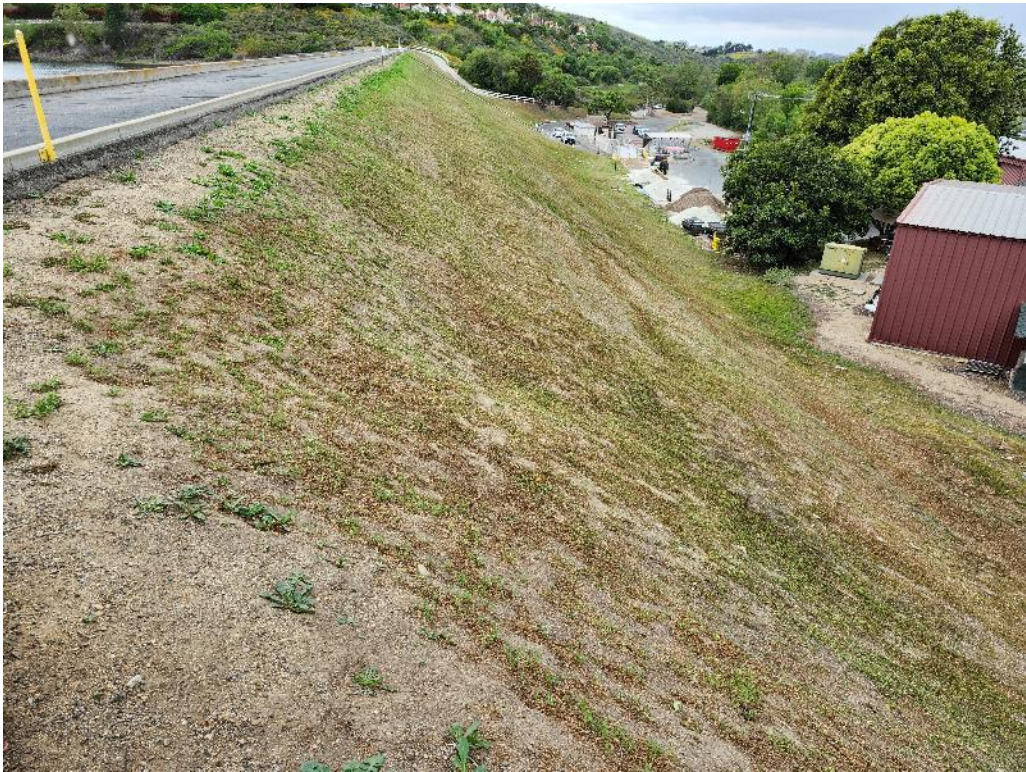
Photo 2. Downstream slope of the dam.
