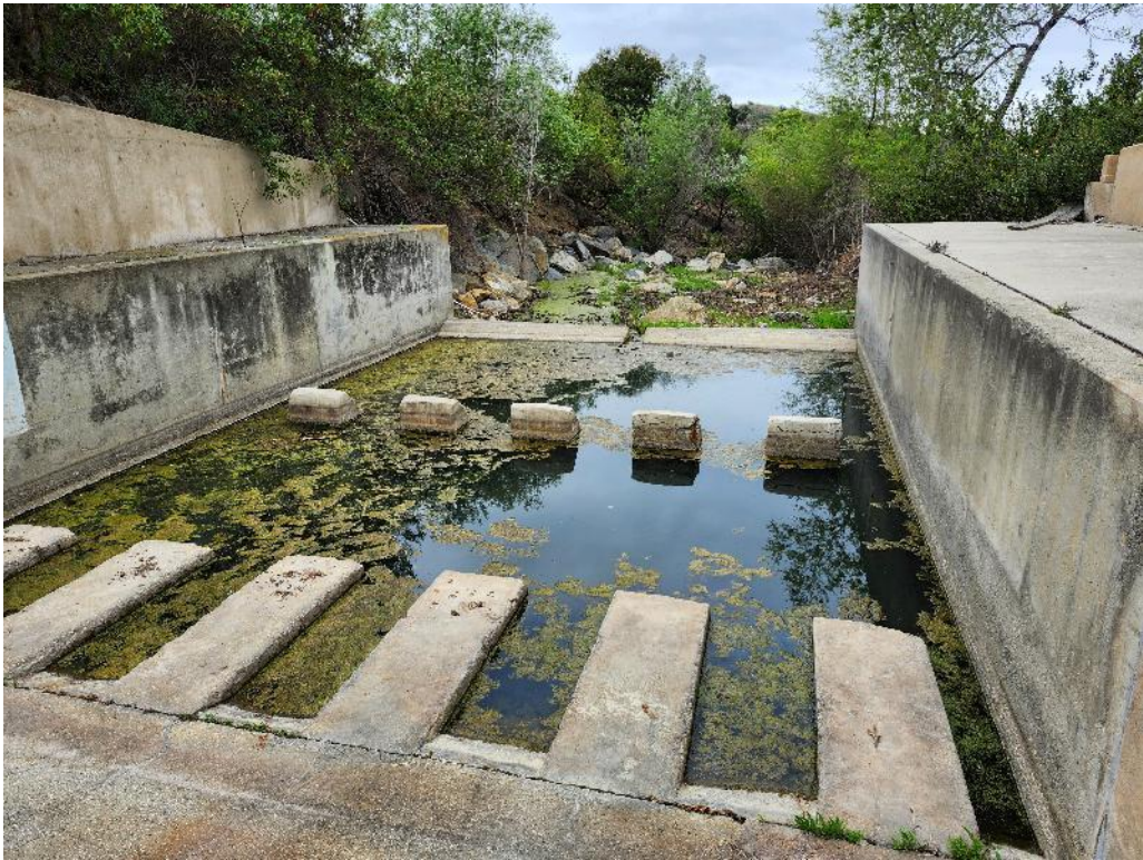
Photo 5. Downstream stilling basin of the spillway.
