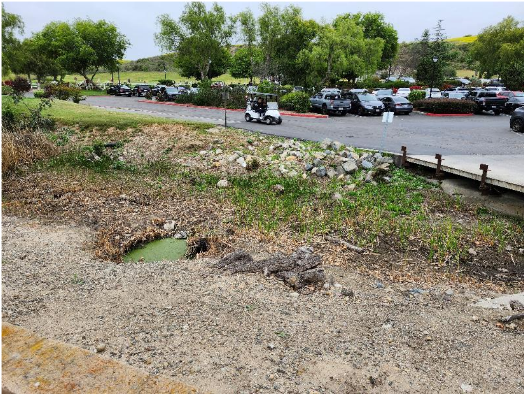
Photo 7. The downstream exit and channel of the low-level outlet.
