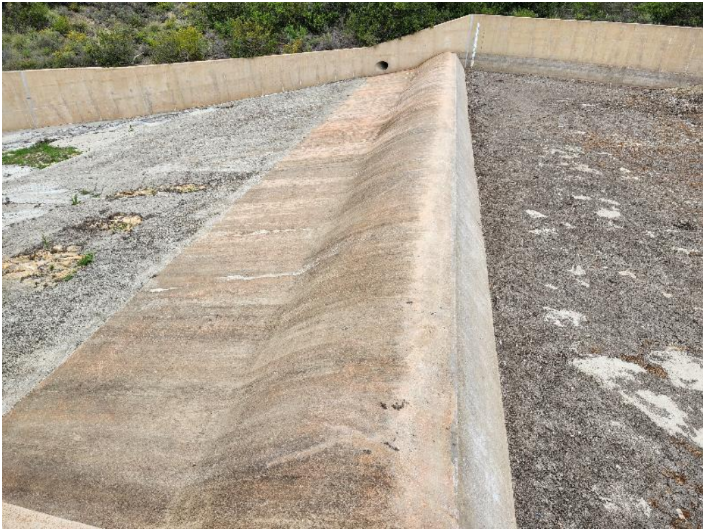
Photo 3. Spillway ogee weir.
