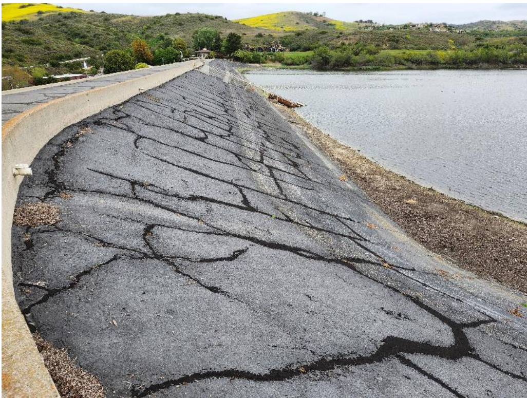
Photo 1. Upstream slope of the dam.
