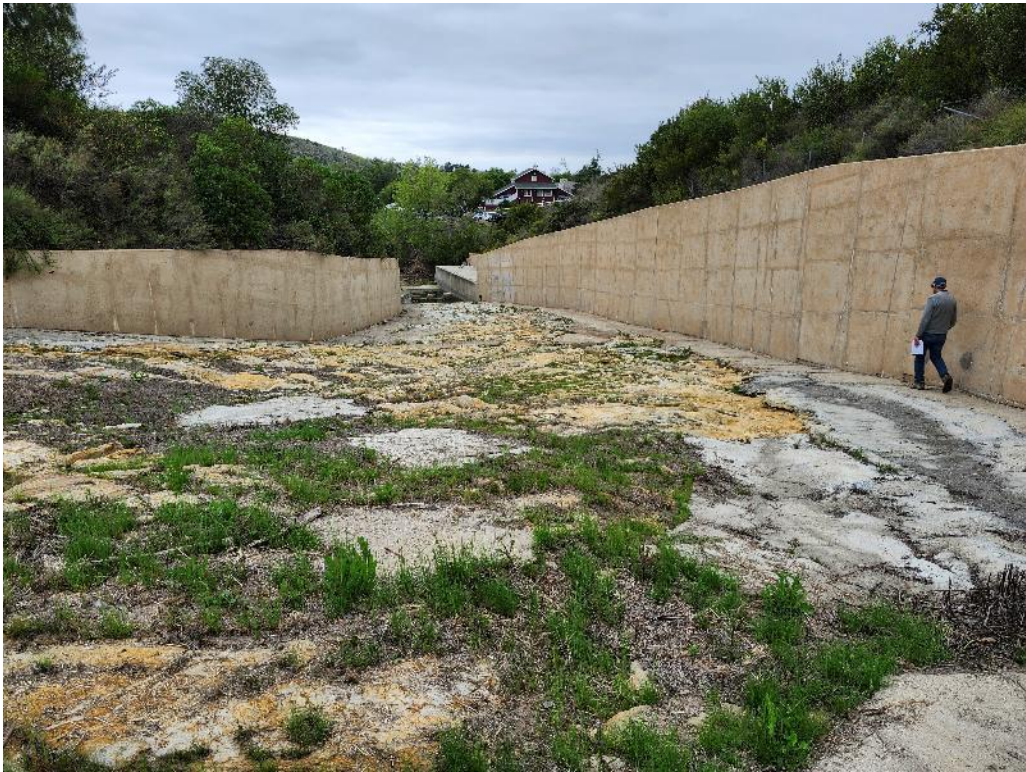
Photo 4. Downstream channel of the spillway.
