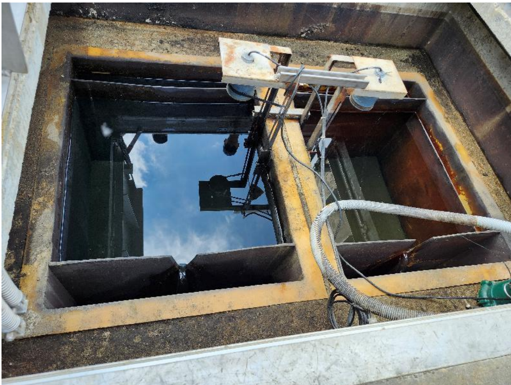
Photo 5. Toe Drain and Floor Drain vault drained by new seepage return line.
