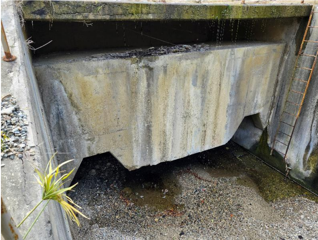
Photo 4. Downstream terminal structure for the spillway.
