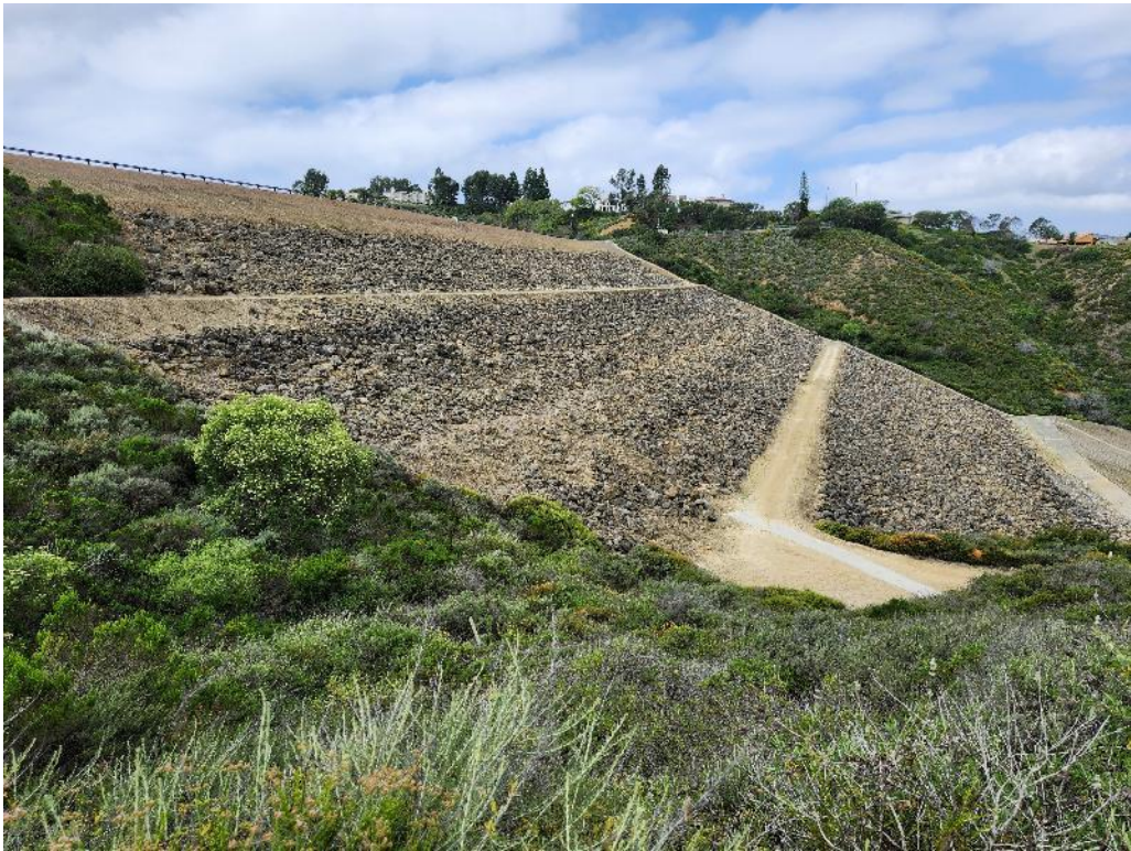
Photo 2. Downstream slope of the dam.
