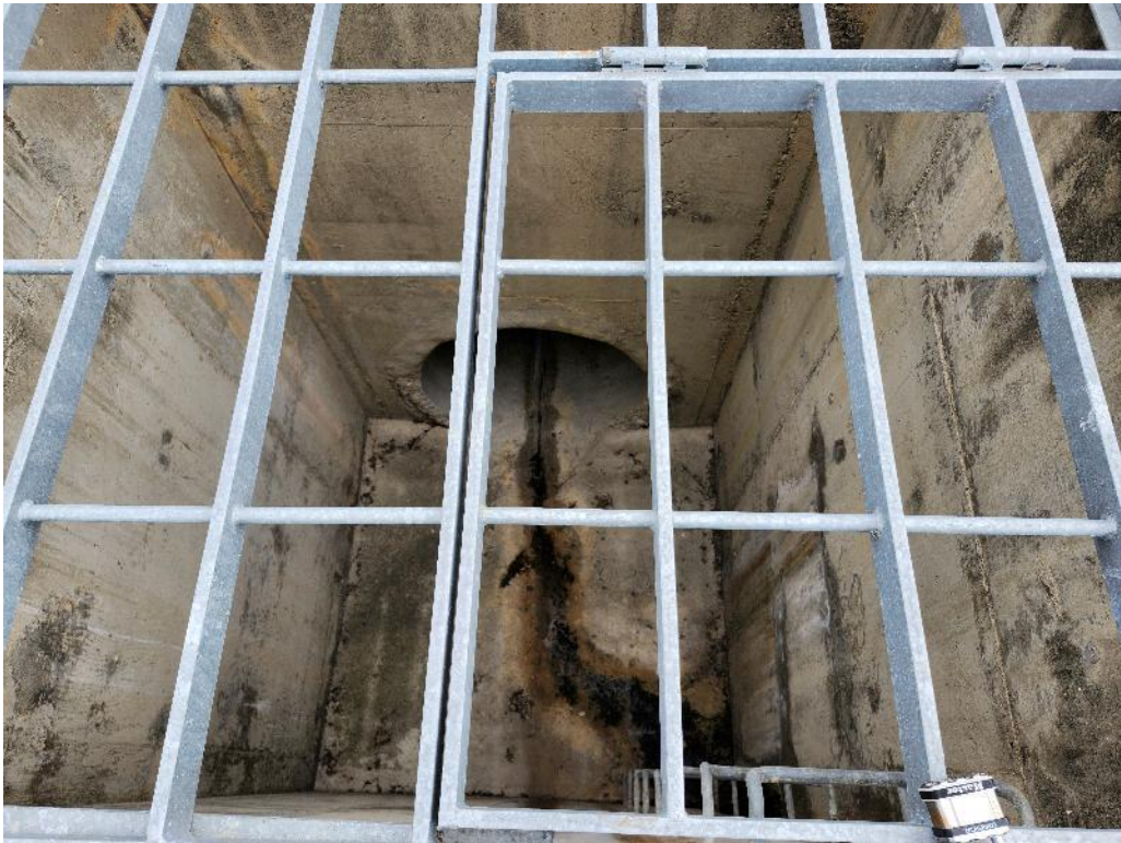
Photo 3. Interior of spillway drop inlet.
