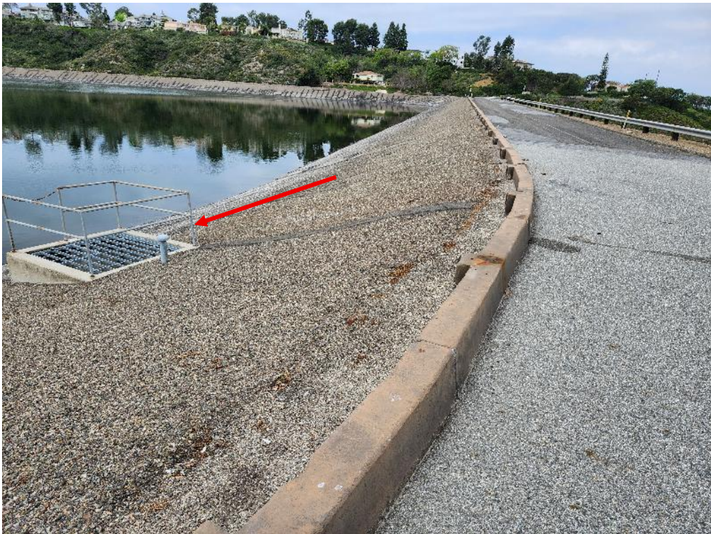
Photo 1. Upstream slope of the dam. Red arrow indicates the right spillway drop inlet.
