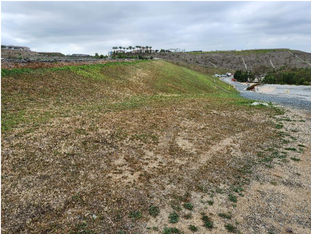
Photo 2. Downstream slope of the dam.
