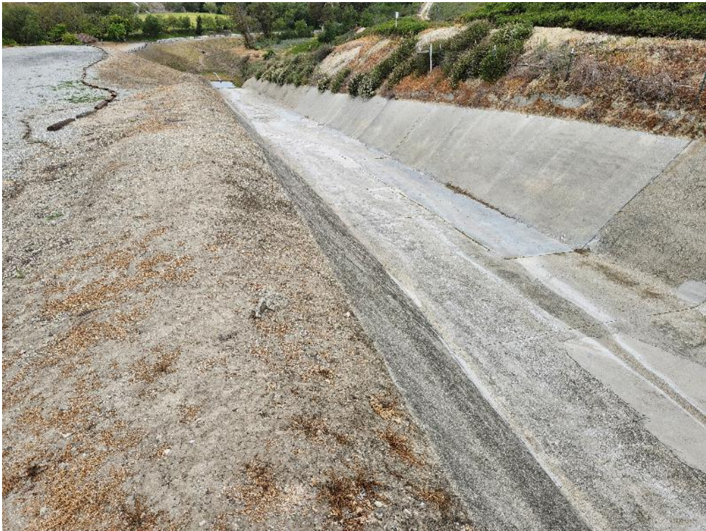
Photo 4. Downstream channel of the spillway.
