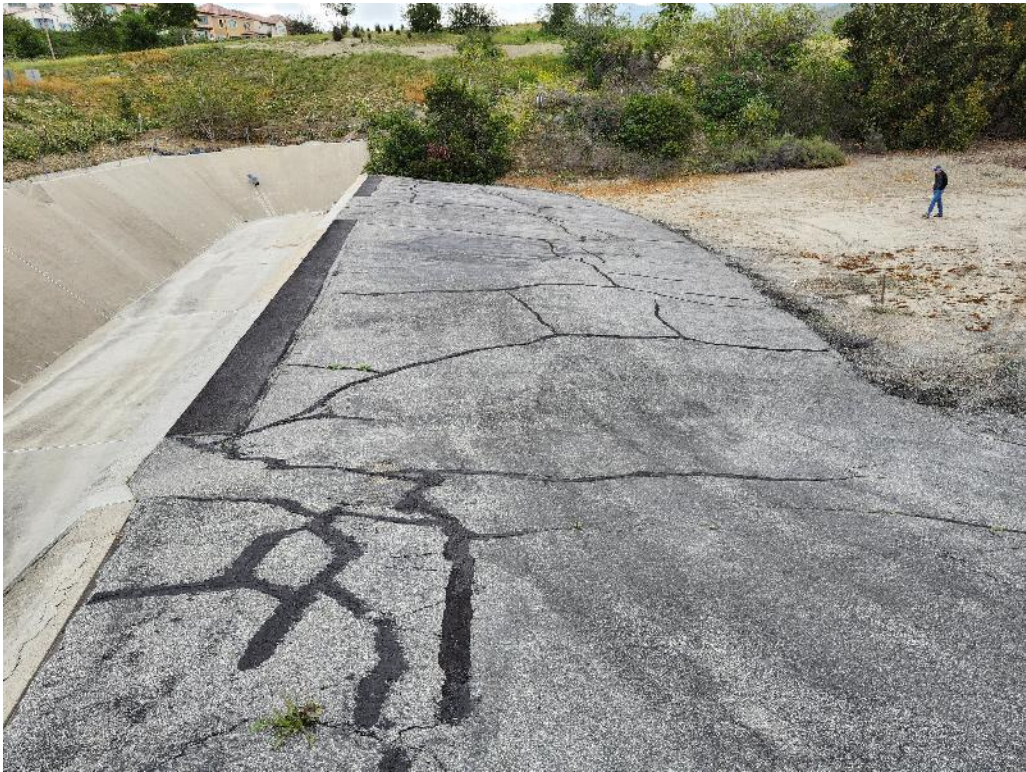
Photo 3. Spillway approach and side channel control section.
