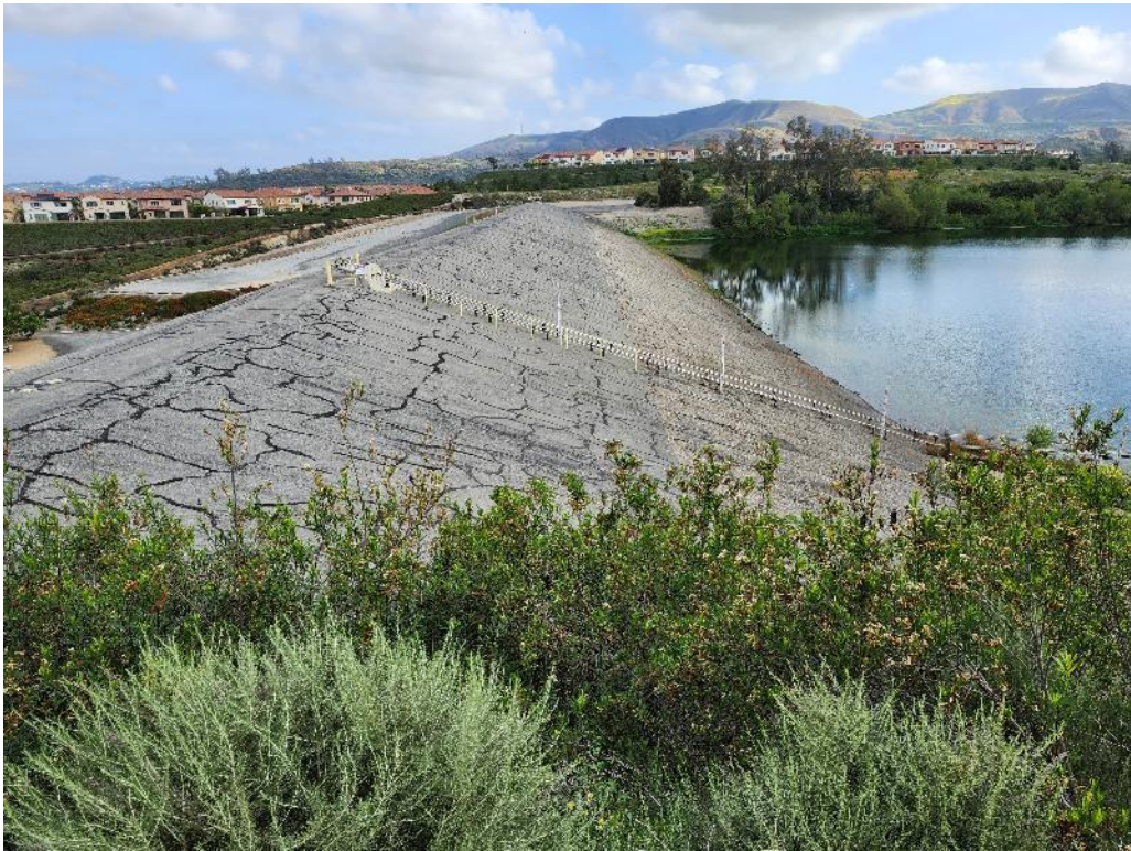
Photo 1. Upstream slope of the dam.
