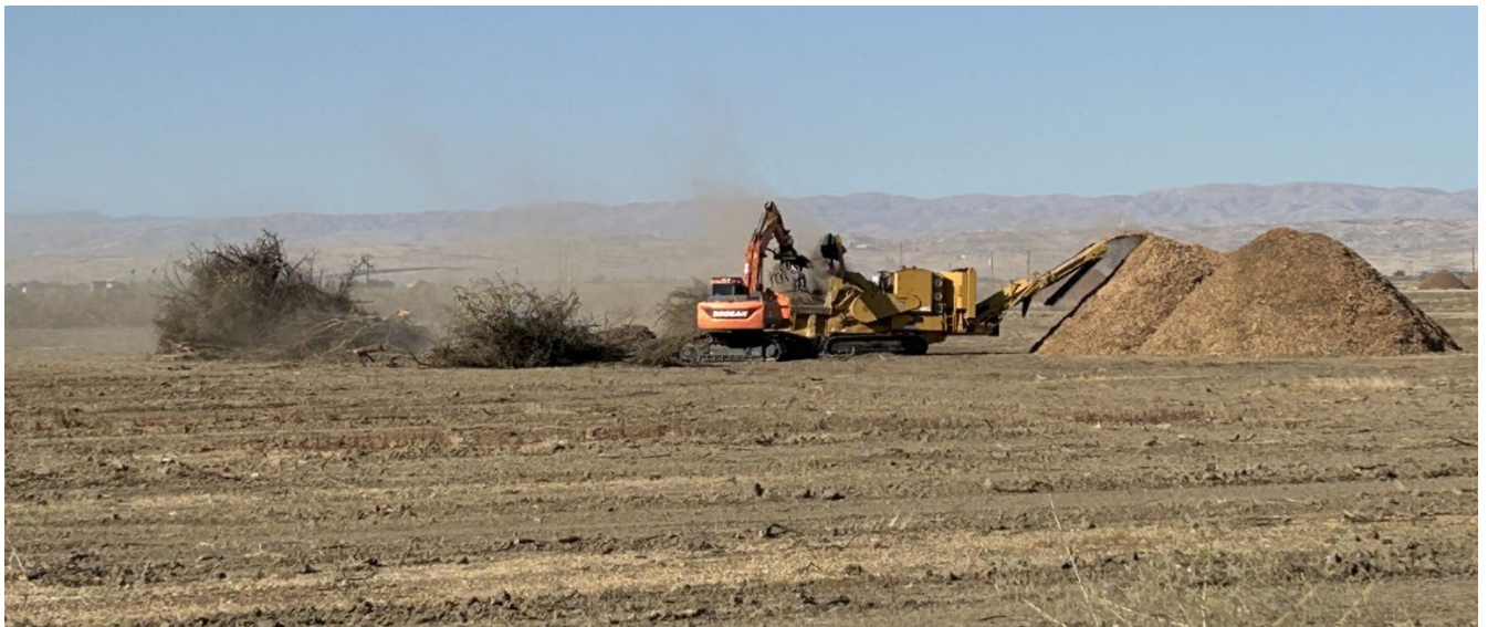
Looking south at grinding operations.
