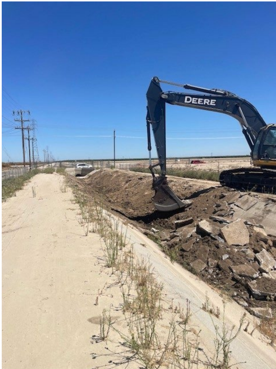
Lining Demolition
