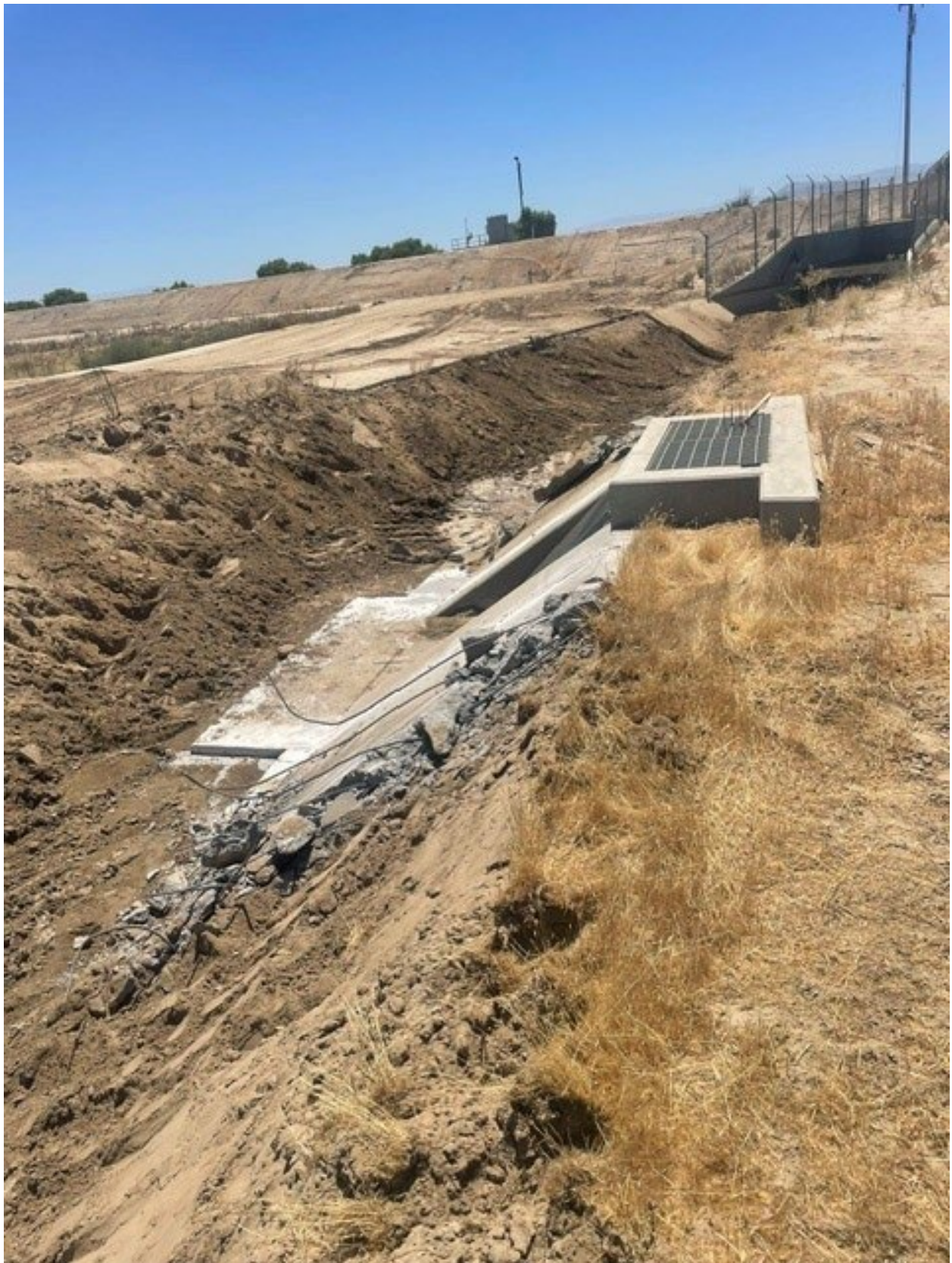
Lining Removal around CVC Intertie Inlet
