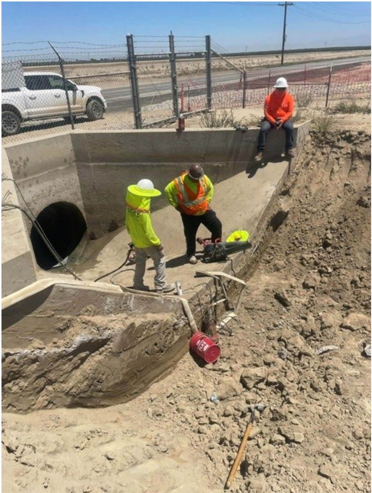
Stockdale Hwy Crossing – Headwall Demolition
