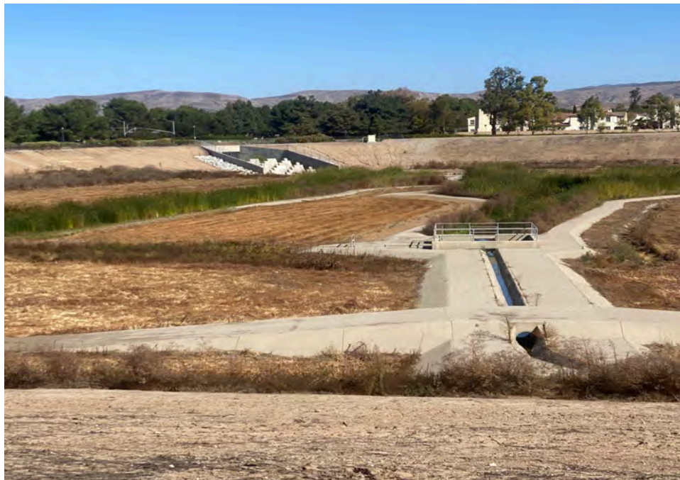
Figure 9. Overview of Trabuco as of November 2024.
