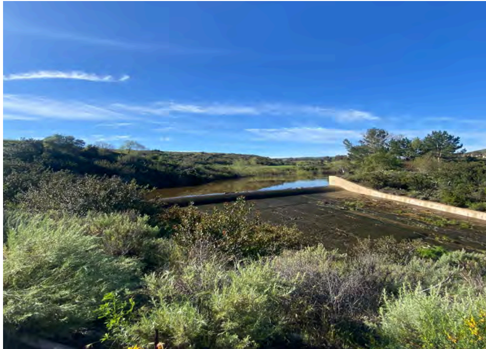
Figure 37. Overview of Ridge Valley C in November, 2024.
