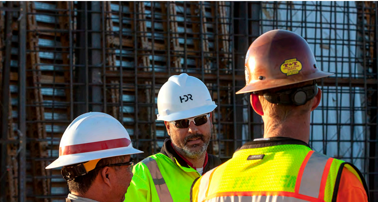
Chris Acosta collaborates with the Kleinfelder inspection team during nighttime concrete placements at the Lake Isabella Dam Safety Modification Project, demonstrating the integrated HDR–Kleinfelder partnership and shared field leadership needed for complex dam construction projects
