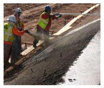
The application of shotcrete is highly specialized and requires a certified nozzleman in order to ensure against rebound which results from a portion of the mortar bouncing away from the surface to which it is applied. It is recommended that the shotcrete lining have a smooth trowel surface in order to improve the hydraulic characteristics.
