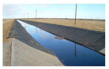
greater than 20% material finer than a 75 micron sieve so that there are fine sands and silts that provide good cohesion. The canal and levee material shall be compacted to a minimum 90% relative compaction and graded to provide a smooth and uniform surface for the installation of the HDPE lining.
