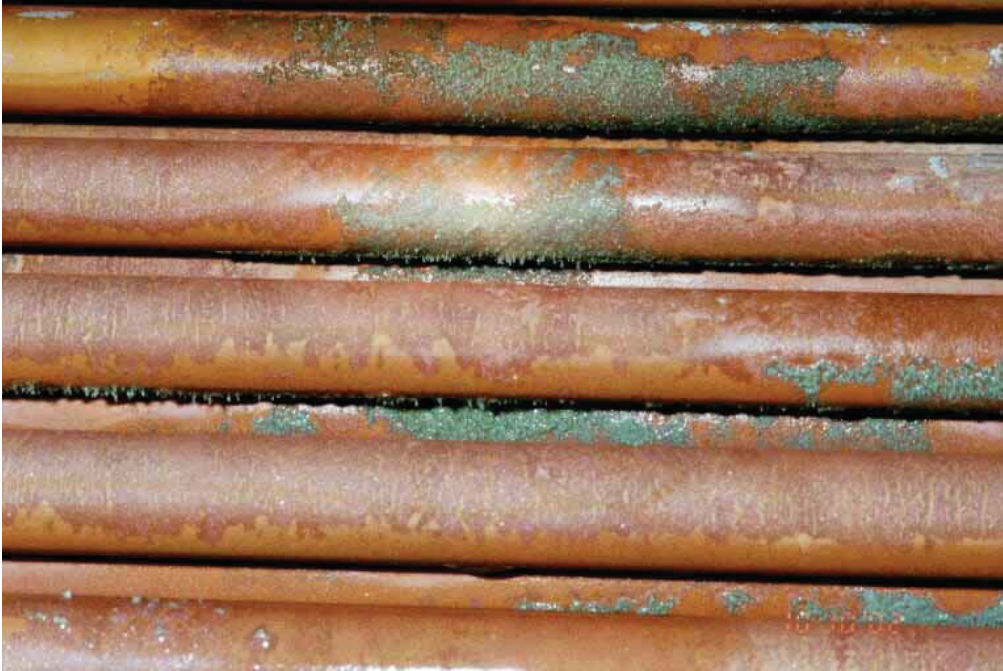
Figure 63: Irvine pipes side-view close-up, October 2002
