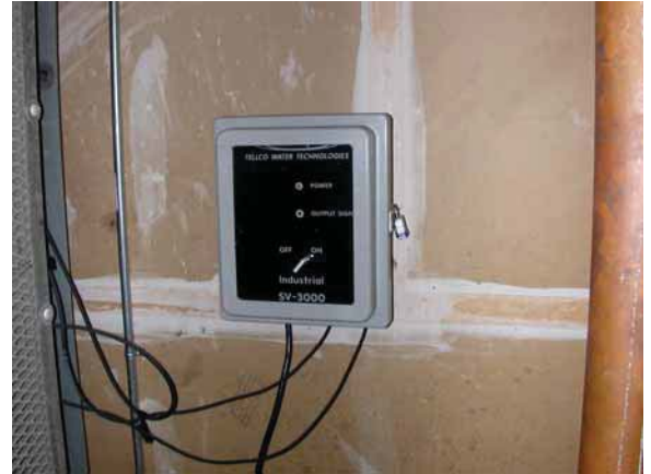
Figure 50: Scale Viper Control Box
