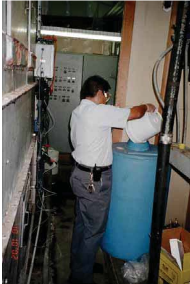
Figure 55: Chemical storage tank at Irvine
