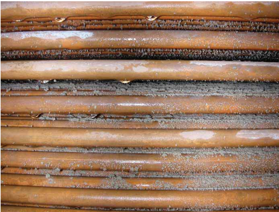
Figure 84: Scale at USC in December
