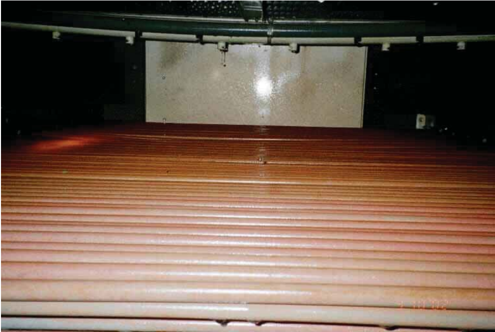
Figure 72: Santa Monica cooling tubes from top, Oct. 2002
