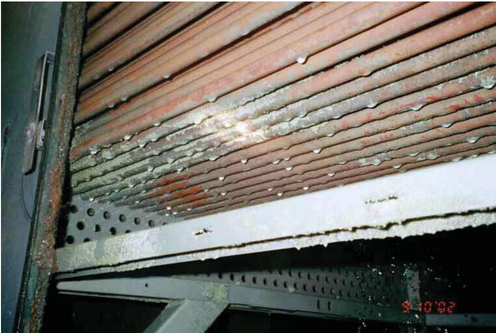
Figure 73: Santa Monica cooling tubes from bottom, Oct. 2002
