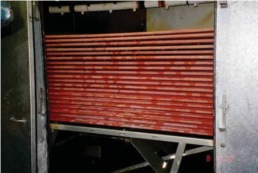
Figure 51: Beverly cooling tubes pre retrofit, September 8, 2002
