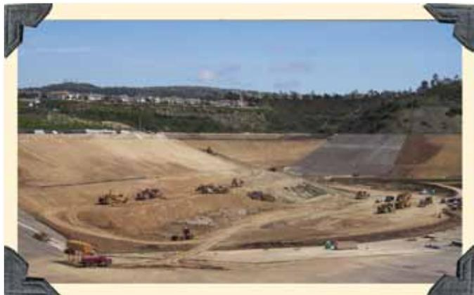
IRWD converted the San Joaquin Reservoir from drinking water storage to a one billion gallon recycled water storage facility in 2004. Here, crews regrade the reservoir to prepare for the installation of a new lining.
