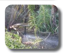
Leaking broken spray heads can quickly create a big usage spike on your water bill. Take time to regularly view each spray head while running your sprinkler system to catch little needed fixes before they become costly leaks.
