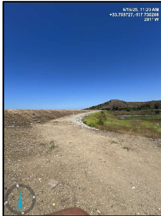
Photo 1) Upstream face looking towards right abutment showing bench and dry reservoir.
