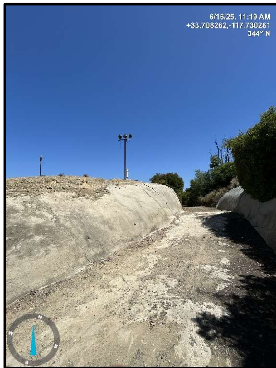
Photo 8) Spillway channel looking upstream.
