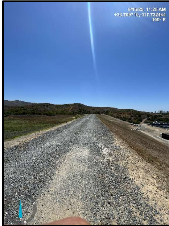
Photo 3) Crest, upstream face, and downstream face looking towards left abutment.
