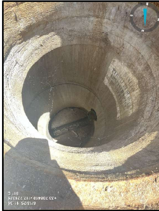
Photo 9) Drain outfall inside dry seepage vault.
