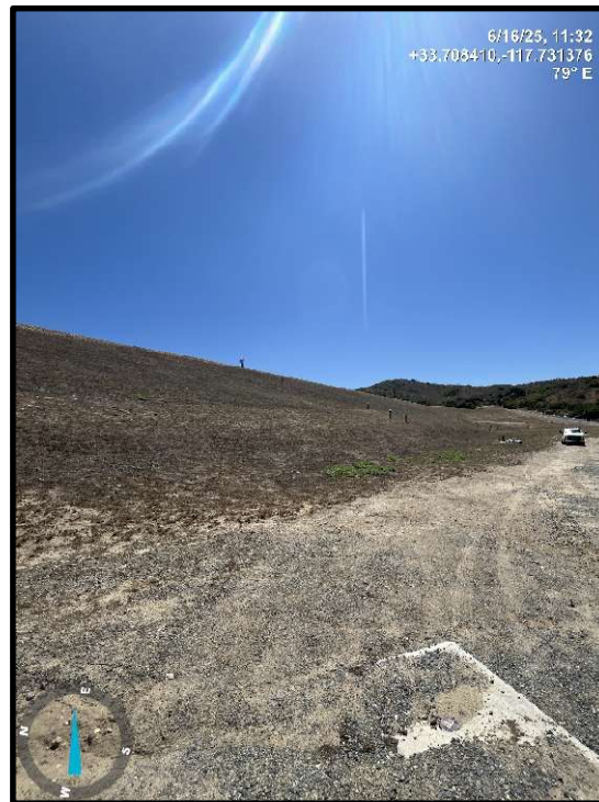
Photo 6) Downstream face from toe looking towards left abutment.
