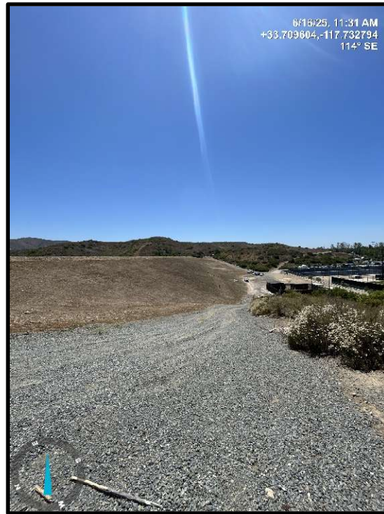
Photo 5) Downstream face looking towards left abutment.
