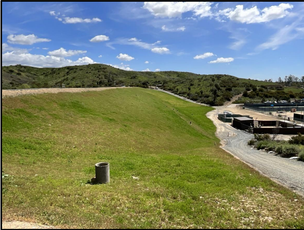
Photo 5) Downstream face looking towards left abutment.
