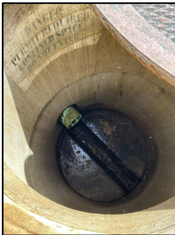
Photo 10) Drain outfall inside dry seepage vault.
