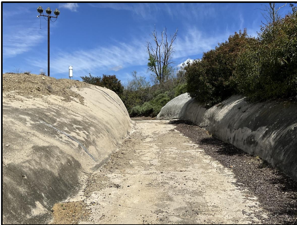
Photo 8) Spillway channel looking downstream.
