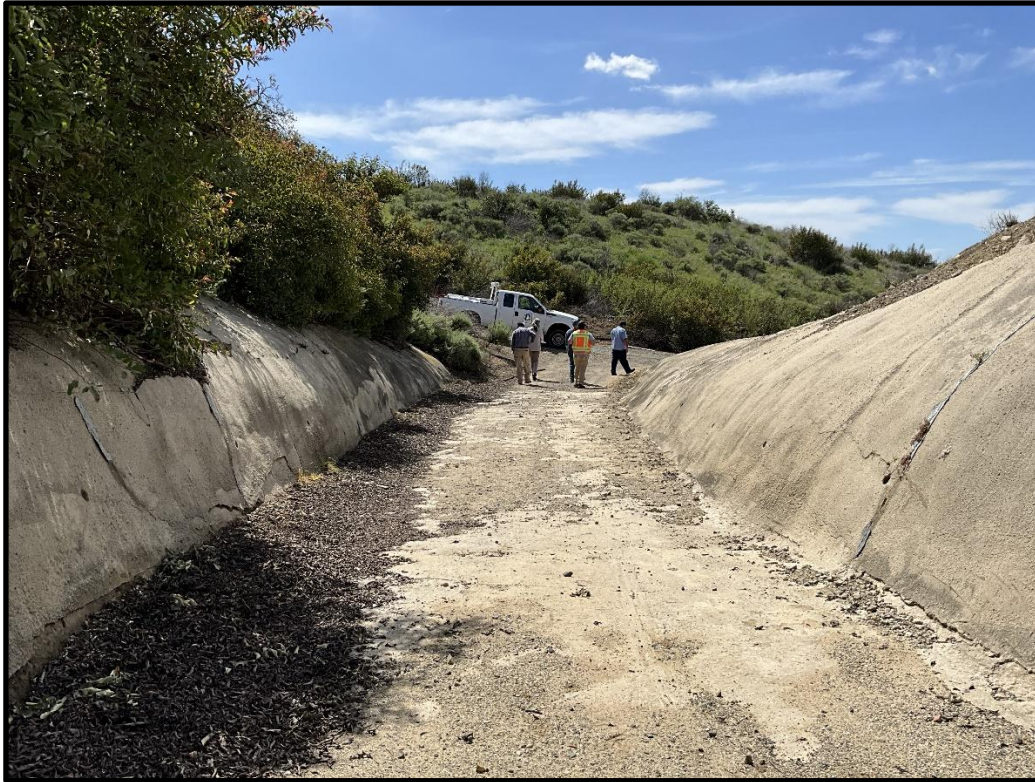
Photo 7) Spillway approach looking downstream.
