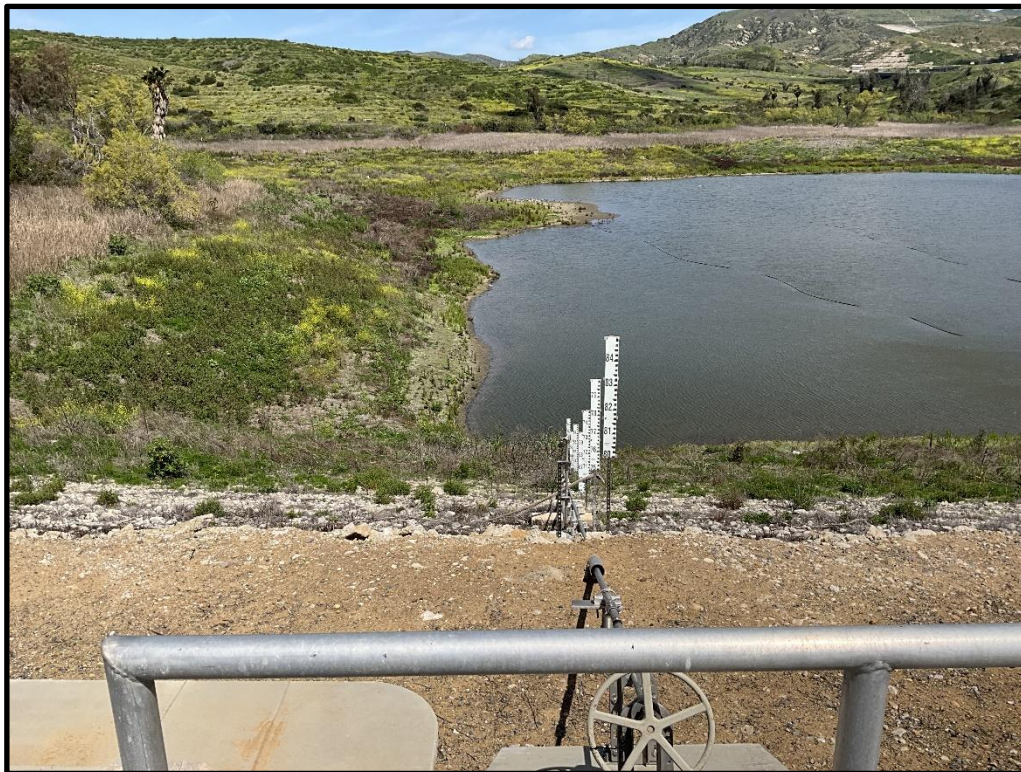
Photo 4) Syphon reservoir and reservoir staff gauge. Note low water level from recent rain.
