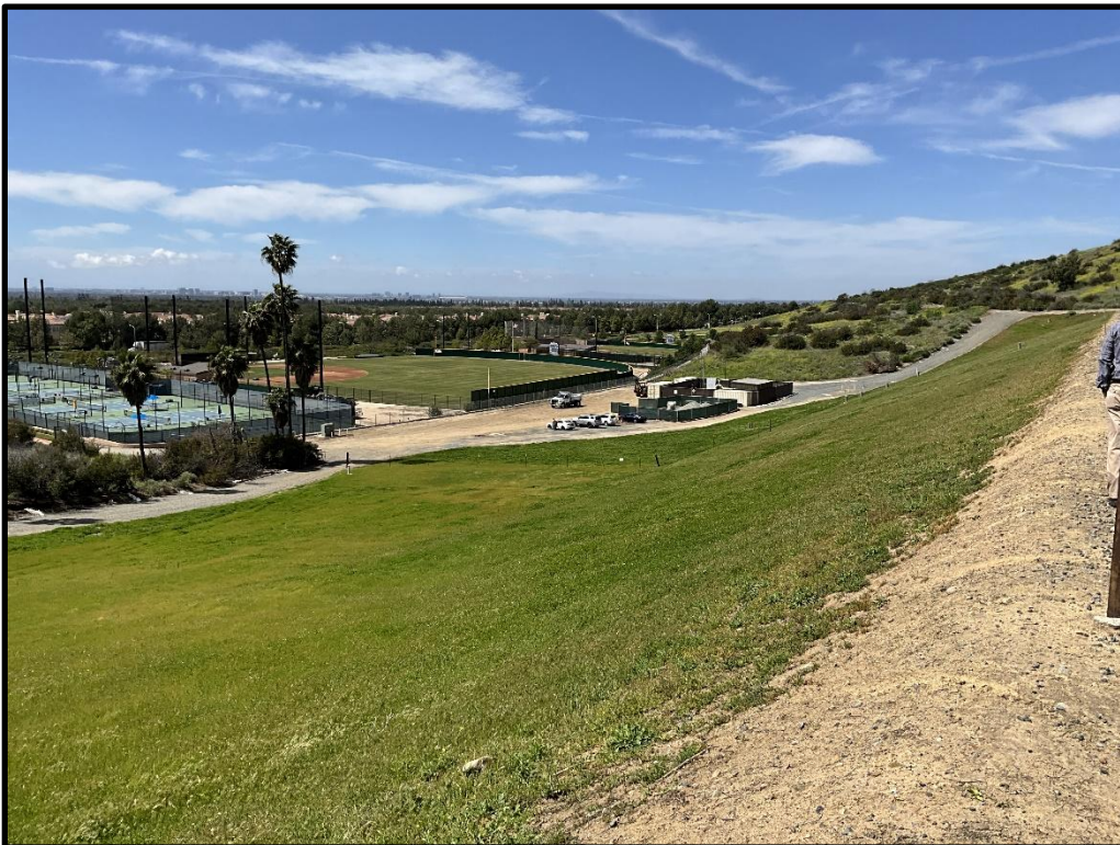
Photo 2) Downstream face looking towards right abutment.
