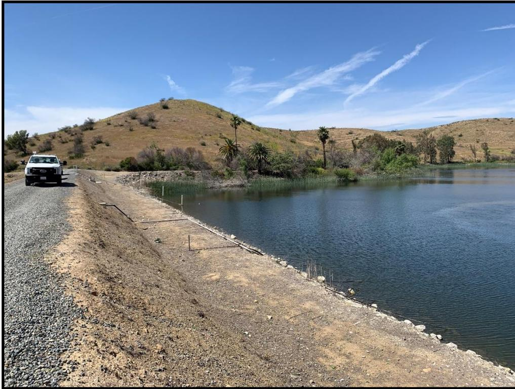
**Photo 1)** Crest and upstream face looking towards right abutment showing bench.
