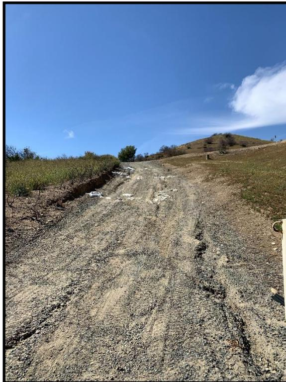
**Photo 12)** Erosion rills at right abutment access road.
