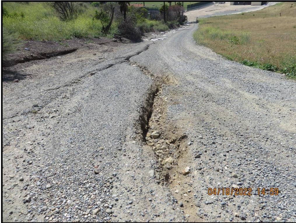
**Photo 11)** Erosion rills at left abutment access road.
