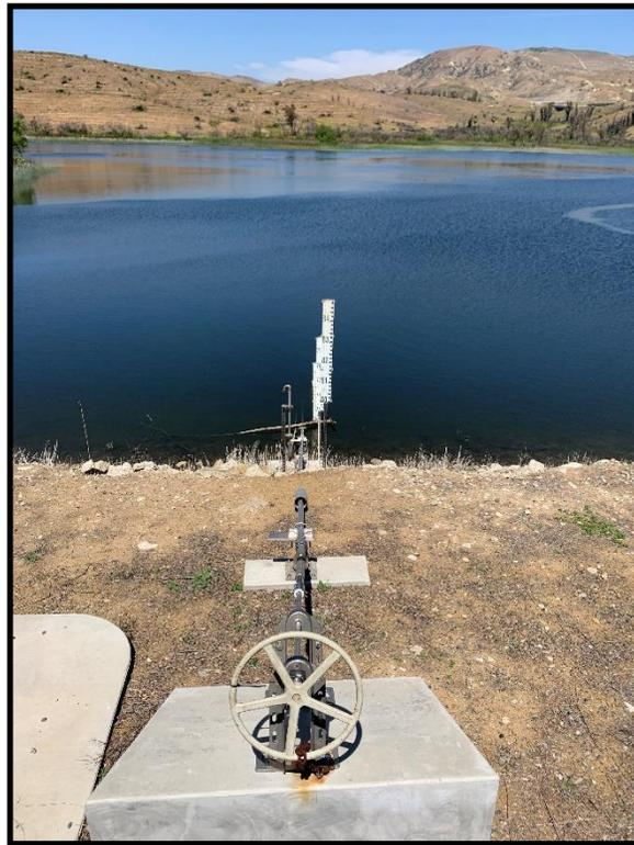
**Photo 9)** Outlet valve wheel and stem and reservoir staff gauge.
