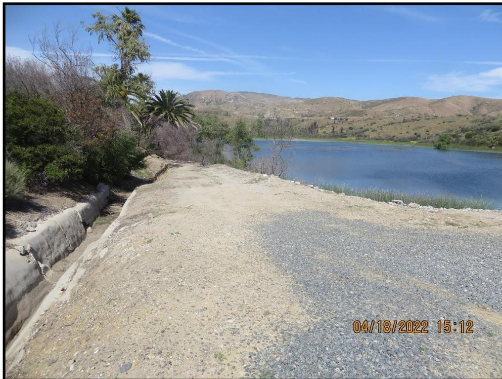
**Photo 4)** Old ditch and vegetation growing on right upstream groin riprap area.
