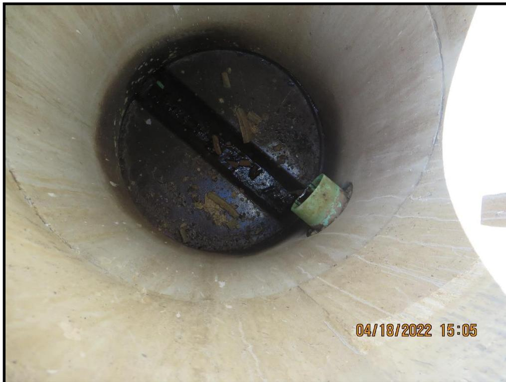
**Photo 10)** Drain outfall inside the seepage vault.
