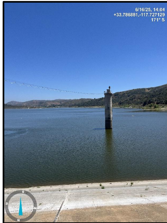
Photo 21) Concrete outlet tower.
