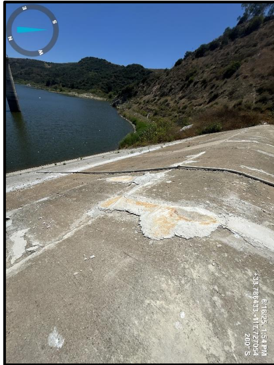
Photo 11) Concrete patch work on concrete panels.
