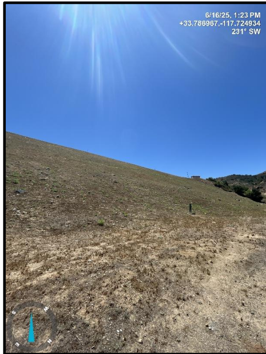
Photo 4) Downstream face looking towards left abutment.
