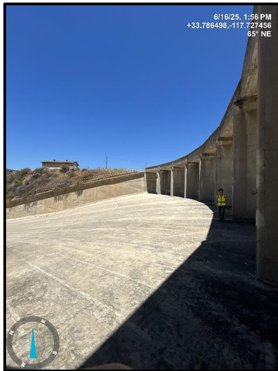
Photo 16) Spillway chute and bridge, looking east.
