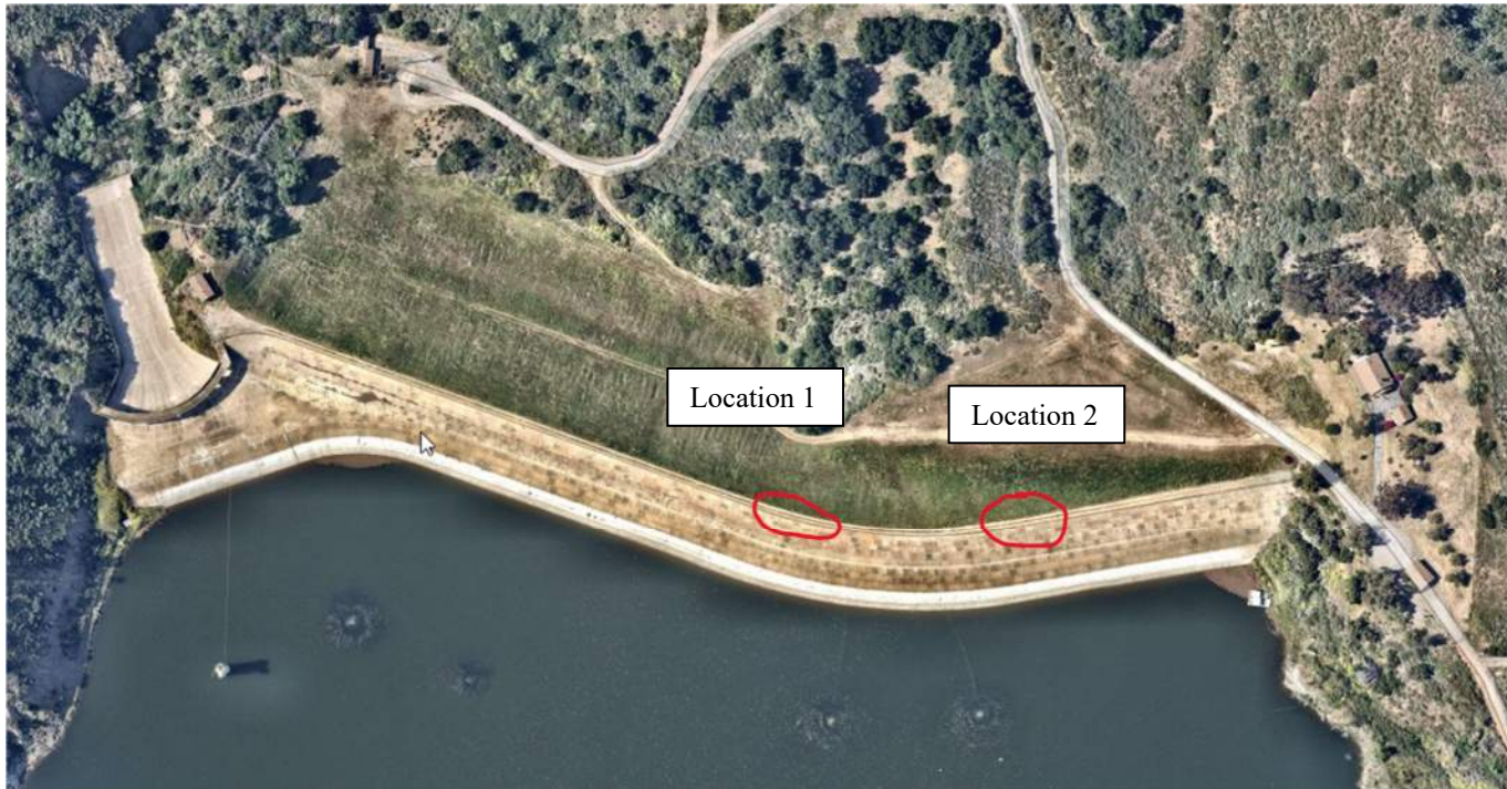
Figure 1: Aerial of Santiago Creek Dam with approximate dam crest crack locations.
