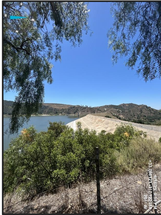
Photo 1) Dam crest, upstream face, and downstream face looking towards left abutment.
