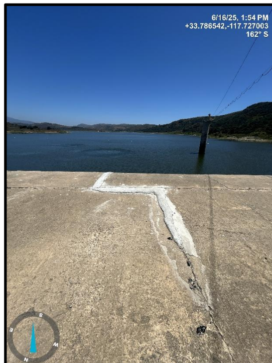
Photo 10) Concrete patch work on concrete panels. Note outlet tower in background
