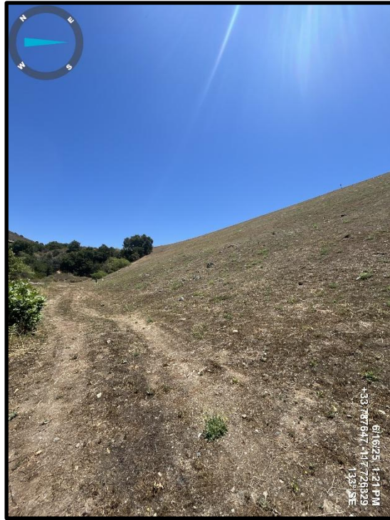
Photo 5) Downstream face bench looking towards right abutment.
