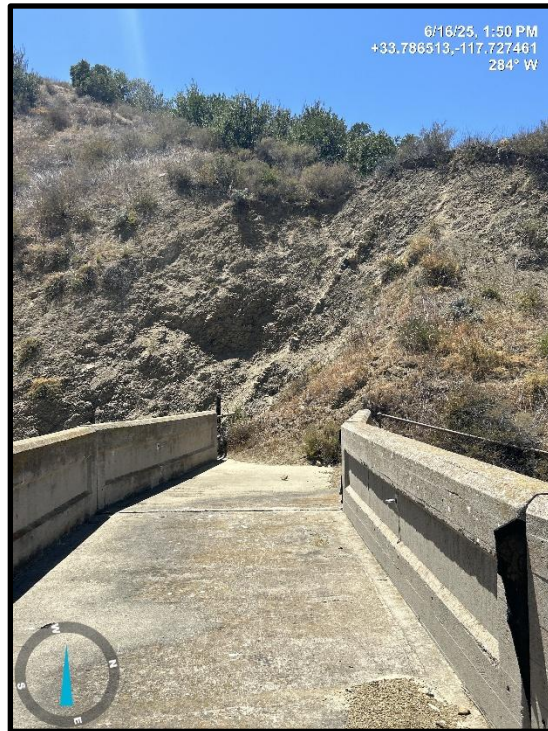
Photo 9) View of left abutment from spillway bridge. Note recently cleared sediment..
