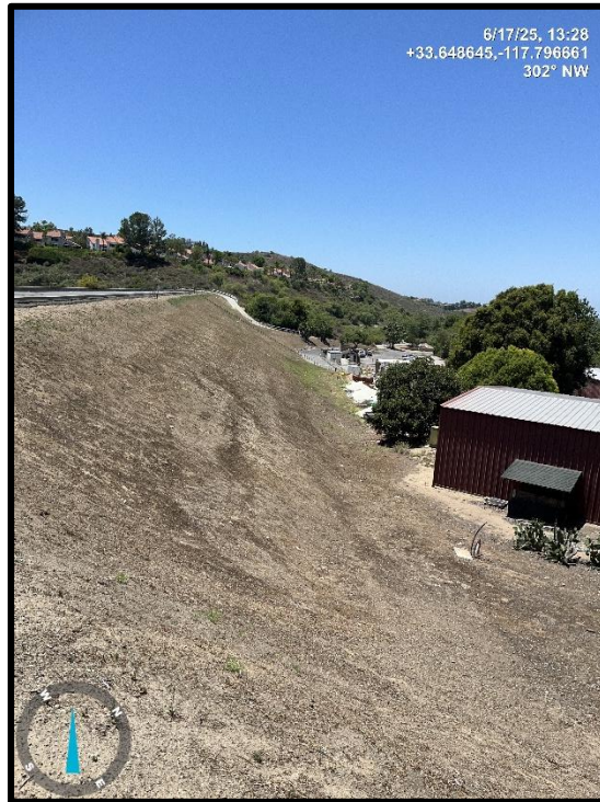
Photo 7) Downstream face of dam. Looking towards left abutment.
