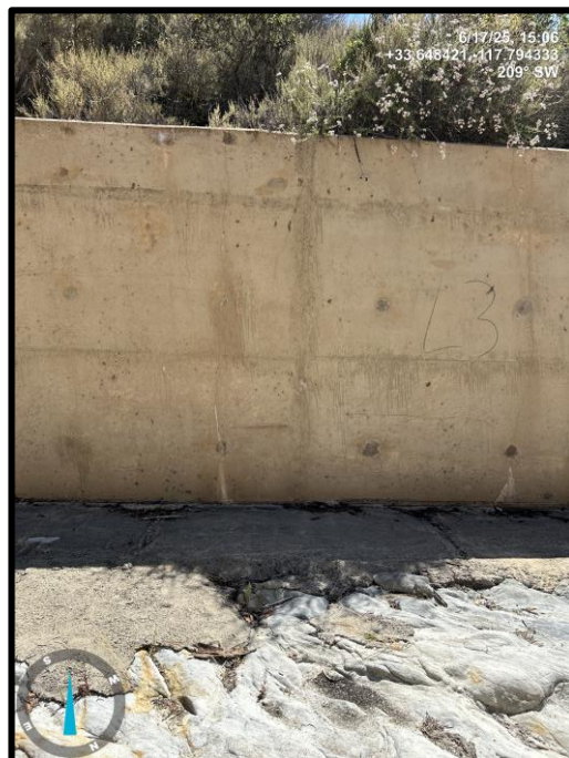
Photo 28) View of spillway wall panel L3.
