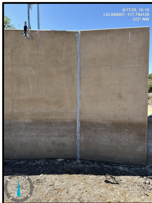
Photo 10) Recently repaired joint.
