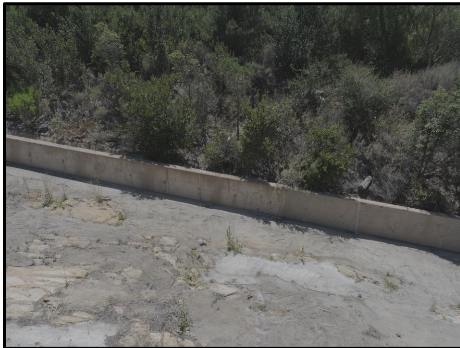
Photo 8) View of spillway wall panel L1.
