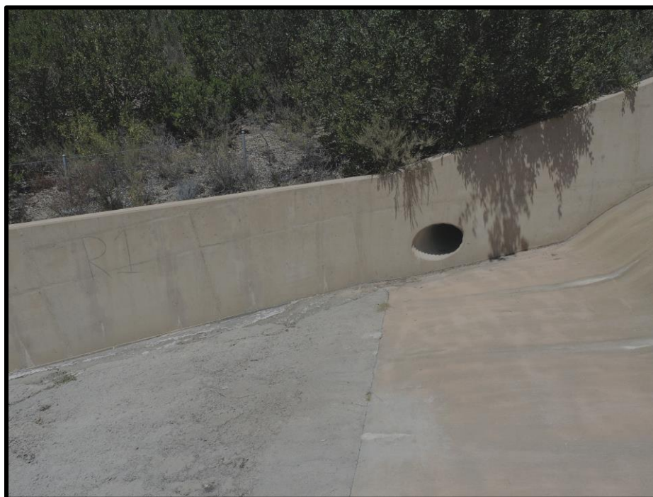
Photo 6) View of spillway wall panel R1.
