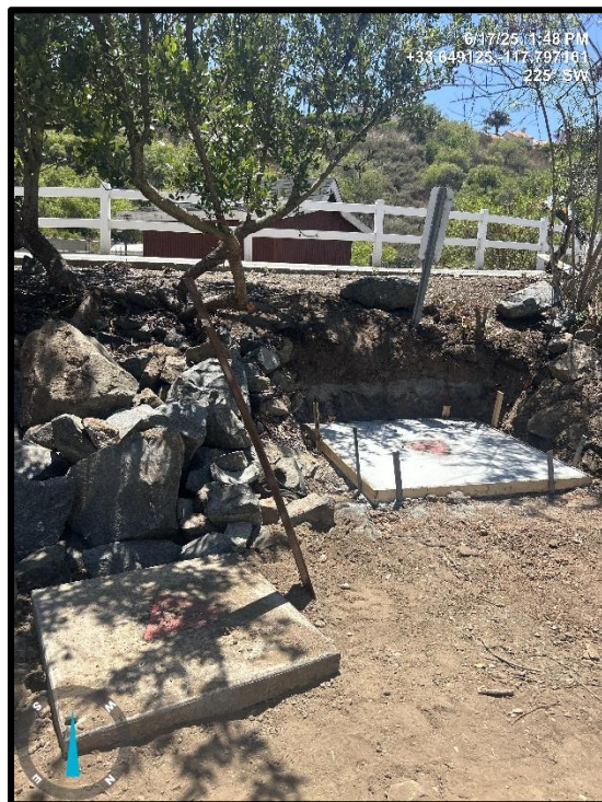
Photo 16) Close up of new concrete pads and access to emergency valves.
