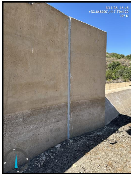
Photo 11) Recently repaired joint.
