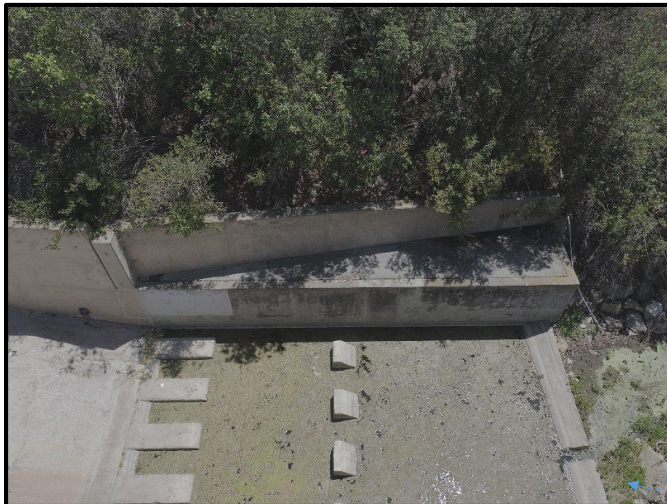
Photo 12) Close up view of spillway stilling basin. Note brush/tule growth downstream.
