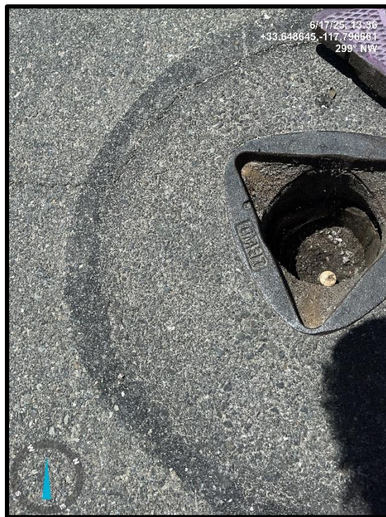
Photo 18) Close up view of Piezometer P-4.
