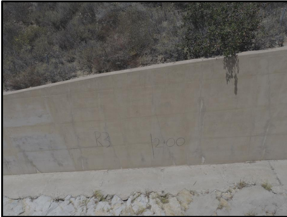
Photo 31) View of spillway wall panel R3.
