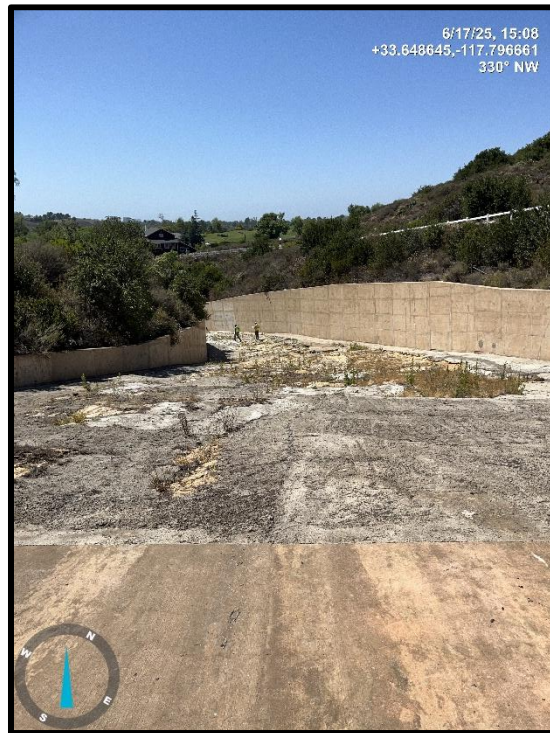
Photo 10) Spillway channel looking downstream. Note vegetation.
