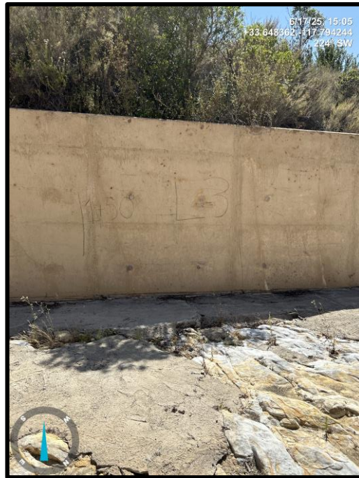
Photo 27) View of spillway wall panel L3.
