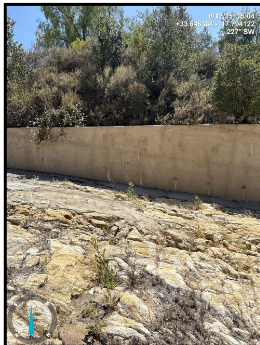
Photo 22) View of spillway wall panel L2.
