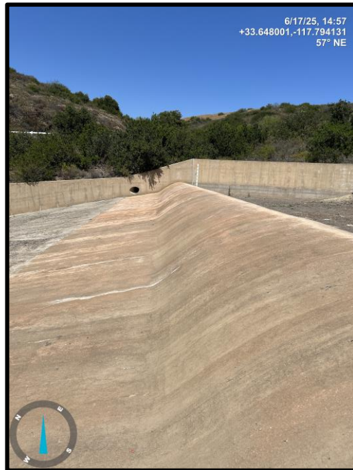
Photo 7) View of spillway ogee weir looking northeast.
