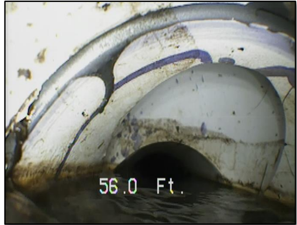
Photo 16 – STA 00+56: Change in the pipe diameter.
