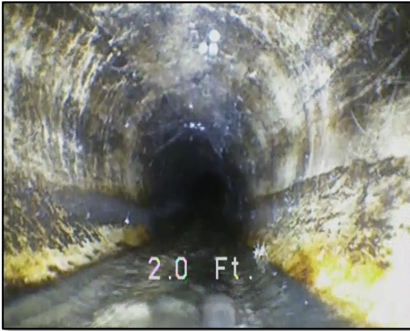
Photo 11 – STA 00+02: Pipe is in good condition with 100% staining on pipe walls.
