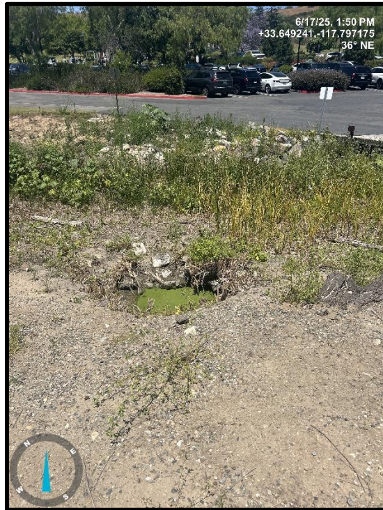
Photo 15) Sand Canyon creek. Note minor vegetation growth and outlet outfall.
