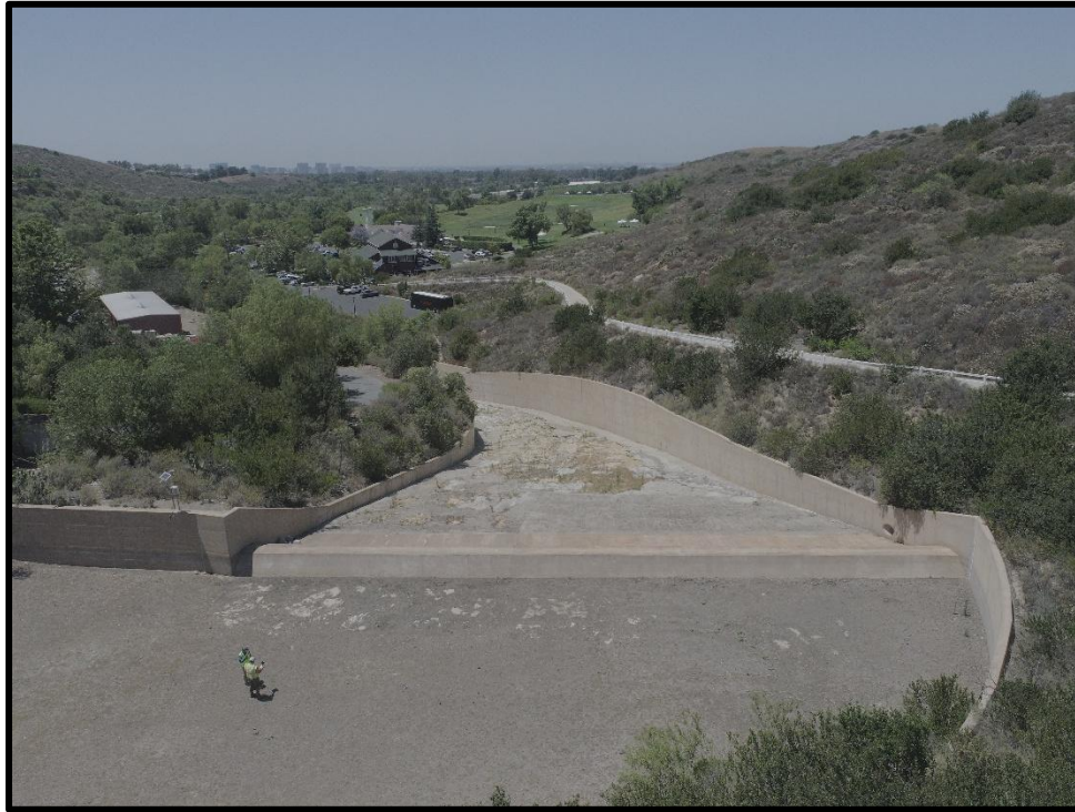
Photo 9) Spillway control ogee section and approach.
