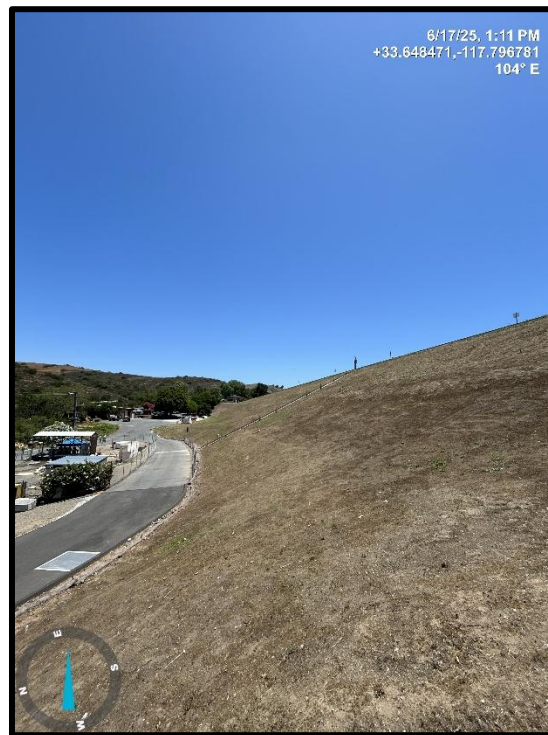
Photo 6) Downstream face of dam. Looking towards right abutment.
