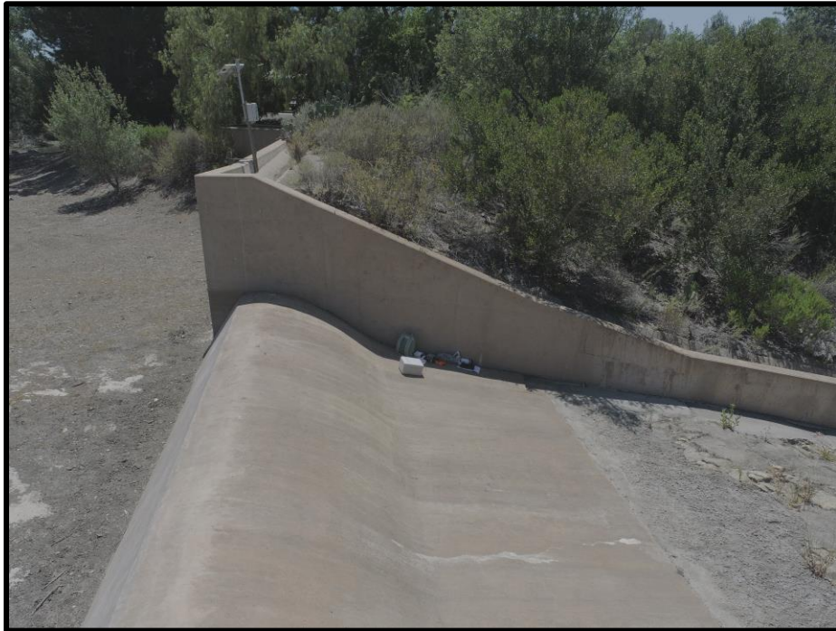
Photo 9) View of spillway wall panel L1.
