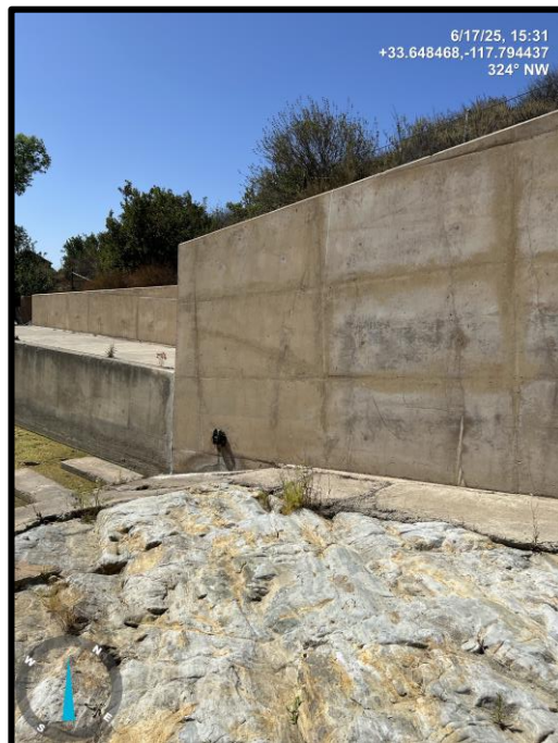
Photo 32) View of spillway wall panel R3 looking downstream. Note spillway drain.
