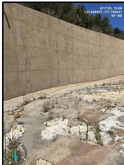
Photo 30) View of spillway wall panel R3 looking upstream.
