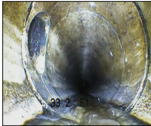
Photo 12 – STA 00+39: Lateral tap connection at 9 o'clock.
