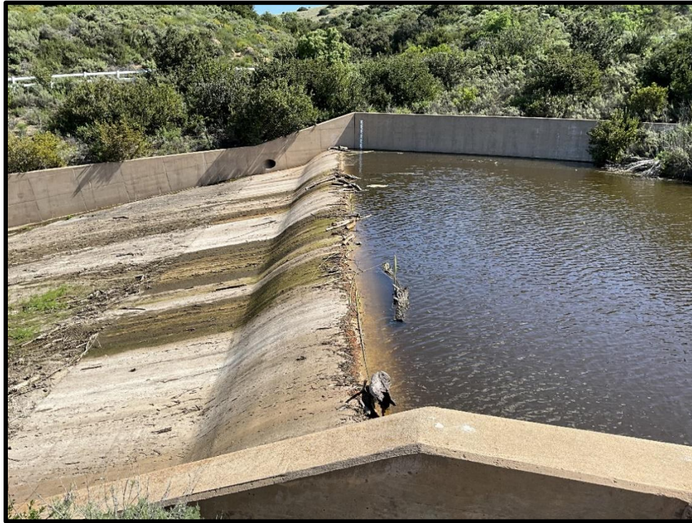
Photo 9) Spillway control ogee section and approach. Note debris and water level.
