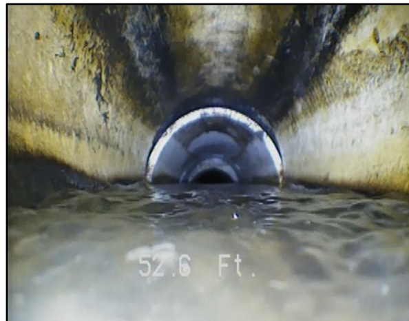
Photo 14 – STA 00+52: 50% water level and change in pipe diameter.
