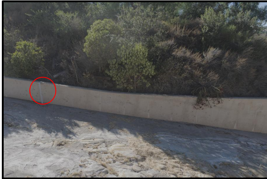
Photo 15) View of spillway wall panels L1 and L2. Note recently repaired wall joint.
