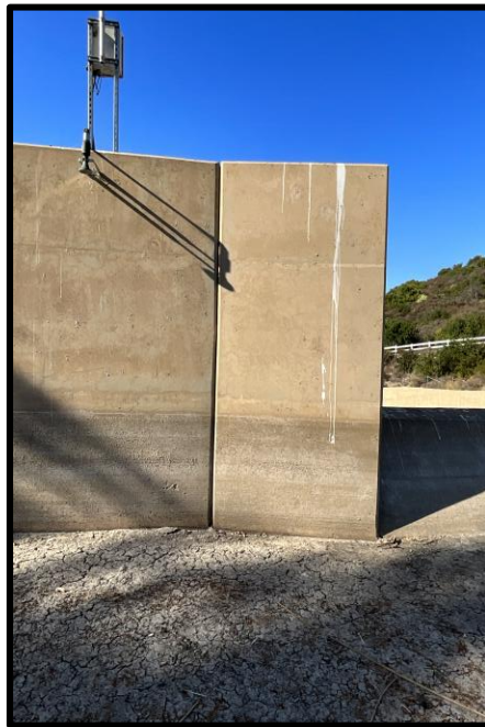
Photo 36) Vertical wall joint \frac{1}{2} " open max with 1 \frac{1}{2} " max wall joint offset.
