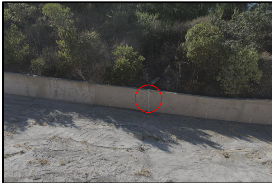
Photo 14) View of spillway wall panels L1 and L2. Note recently repaired wall joint.
