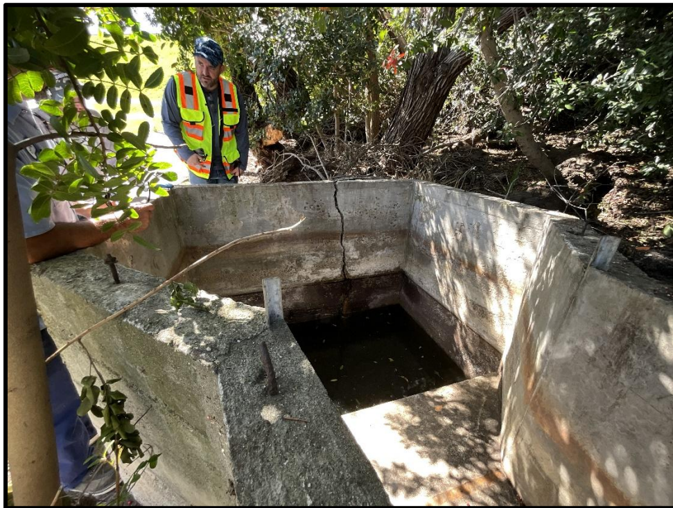
Photo 4) Abandoned irrigation weir box. Note pooled water.
