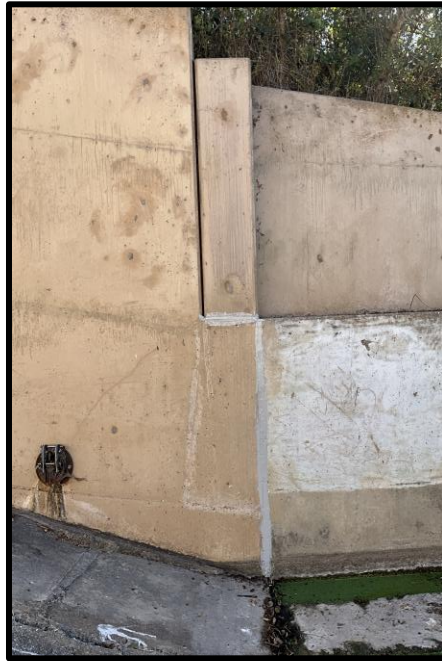
Photo 33) Recently repaired spillway vertical wall joint. Note spillway drain.
