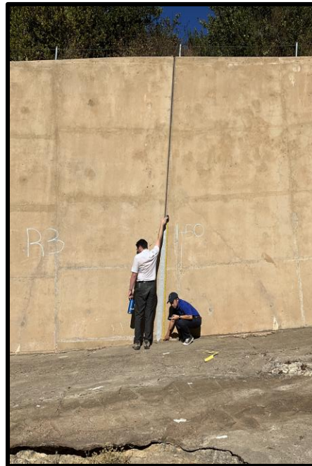
Photo 20) Vertical wall joint open \frac{1}{2} " max between wall panels R2 and R3. Note recent repair of bottom half of joint.
