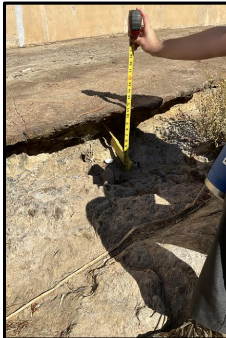
Photo 26) Spillway floor undermining. 11" max height, 12" max depth.
