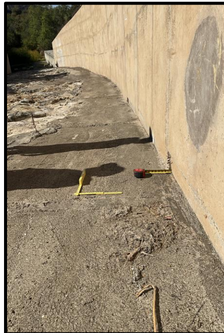
Photo 16) 1" offset at bottom of spillway wall panel R2.
