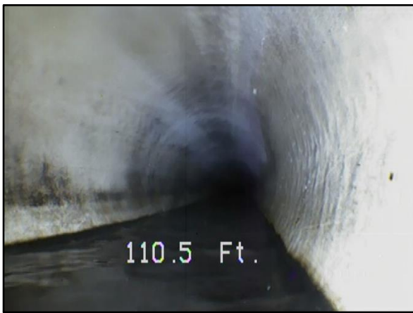
Photo 17 – STA 01+10: Pipe is in good condition.
