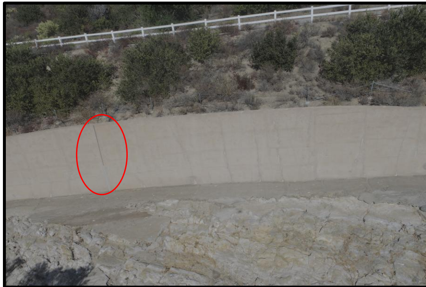
Photo 17) View of spillway wall panels R2 and R3. Note recently repaired wall joint.
