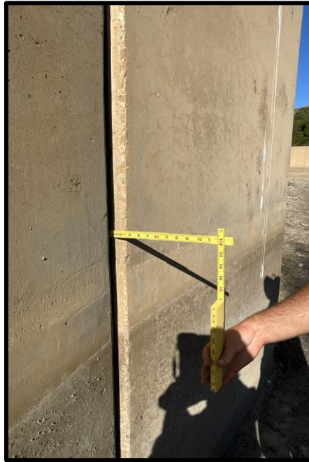
Photo 37) Vertical wall joint \frac{1}{2} " open max with 1\frac{1}{2} " max wall joint offset. 1" void in joint.
