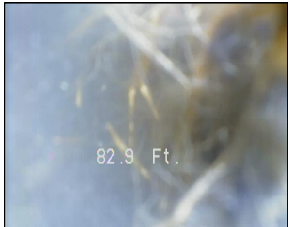
Photo 4 – STA 00+82: Root ball inside pipe.
