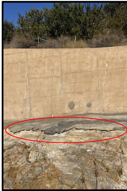
Photo 13) 5" height undermining of spillway floor.
