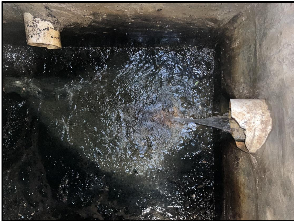
Photo 16) Seepage at left subdrain. Right subdrain was dry.
