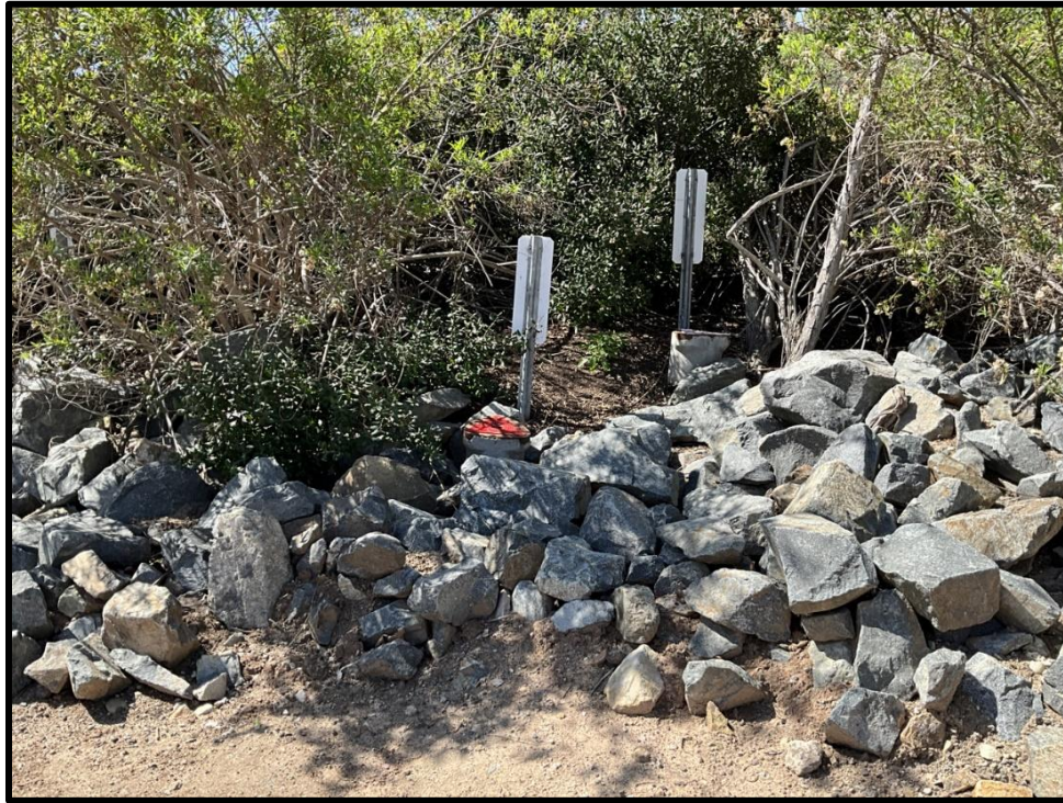
Photo 15) Close up of large diameter angular rocks and vegetation limiting access to emergency valves #23 and #24.
