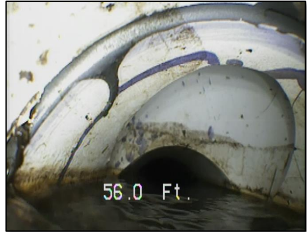
Photo 16 – STA 00+56: Change in the pipe diameter.
