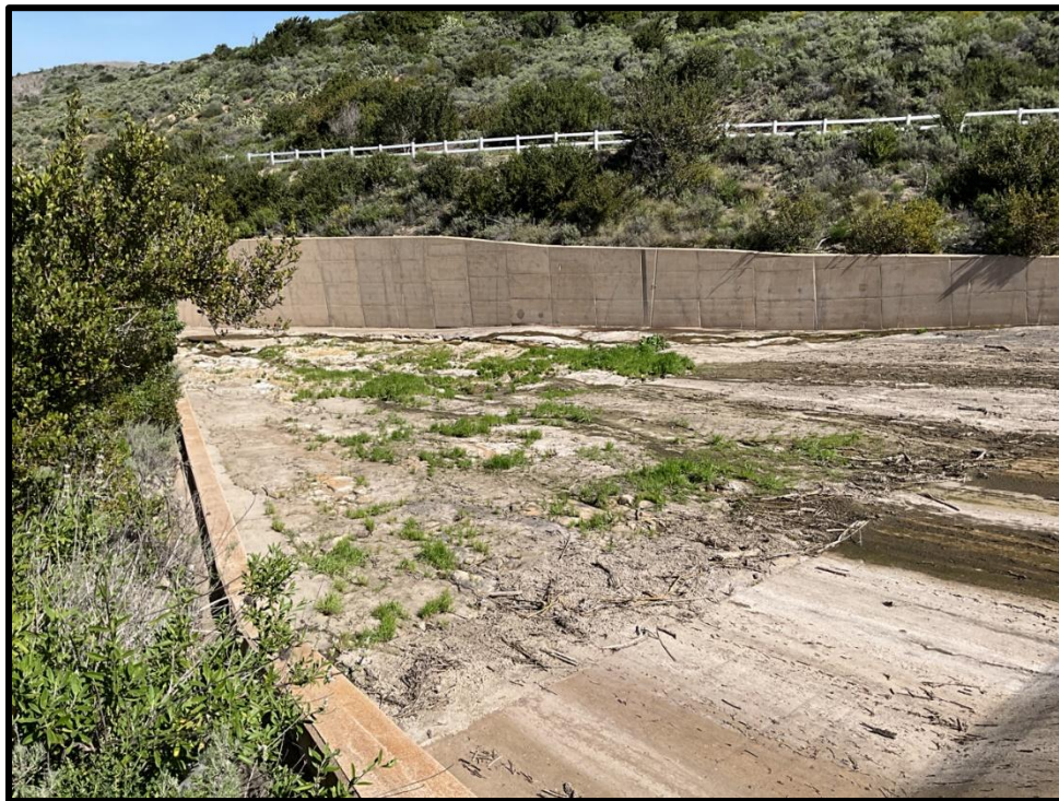
Photo 10) Spillway channel looking downstream. Note vegetation and debris.
