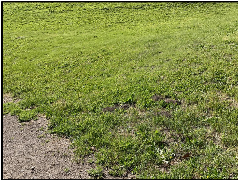
Photo 8) Minor rodent activity on the downstream toe near the left abutment.
