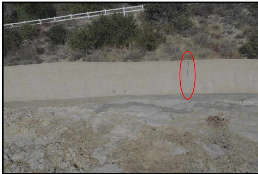
Photo 10) View of spillway wall panel R1 and R2. Note recent vertical joint repair.
