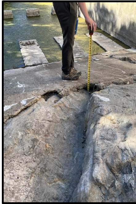
Photo 29) 4.6" downstream slab joint offset at unlined spillway channel and stilling basin transition.
