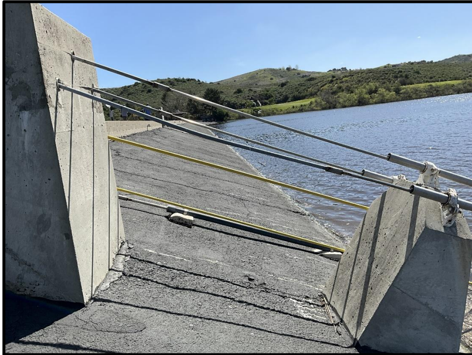
Photo 13) Close up view of the buckled gate valve #2 stem.
