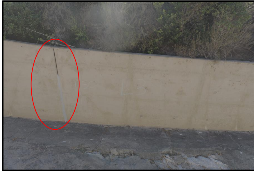
Photo 21) View of spillway wall panels L2 and L3. Note recently repaired wall joint.
