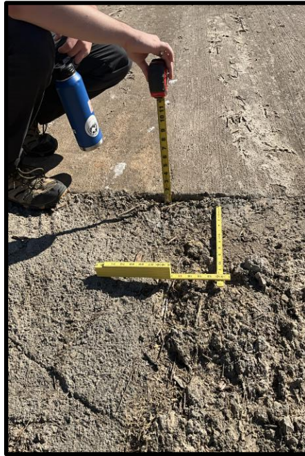
Photo 3) 1" slab joint offset at spillway ogee weir and unlined spillway channel transition.
