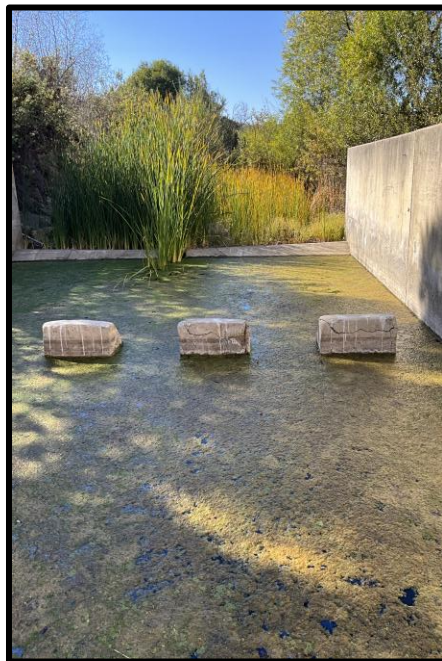
Photo 32) Spillway stilling basin. Note cracks on concrete baffles.
