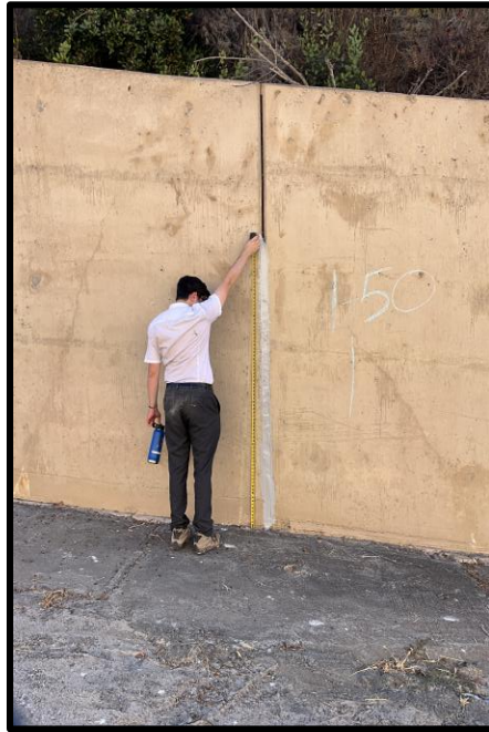
Photo 35) Vertical wall joint open \frac{1}{2} " max between wall panels L2 and L3. Note recent repair of bottom half of joint.
