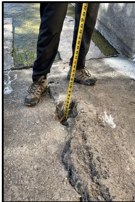
Photo 30) 11" Length (L) x 6" Width (W) x 5" Depth (D) concrete popout at unlined spillway channel and stilling basin transition.
