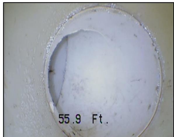
Photo 8 – STA 00+55: 90° bend in the pipe.
