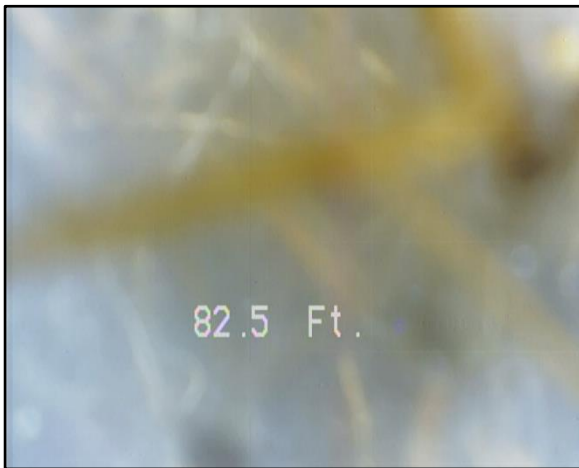
Photo 3 – STA 00+82: Root ball inside pipe.
