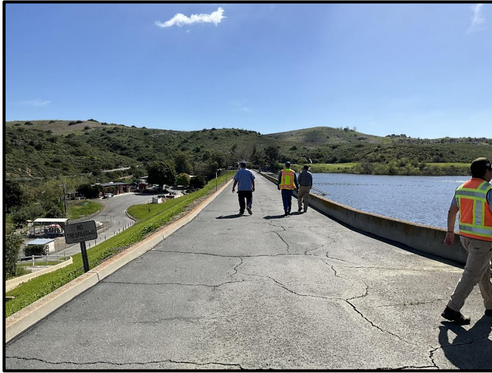
Photo 1) AC paved crest looking towards the right abutment, including 1-foot-high curb wall.
