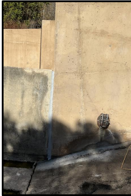
Photo 31) Recently repaired spillway vertical wall joint. Note spillway drain.
