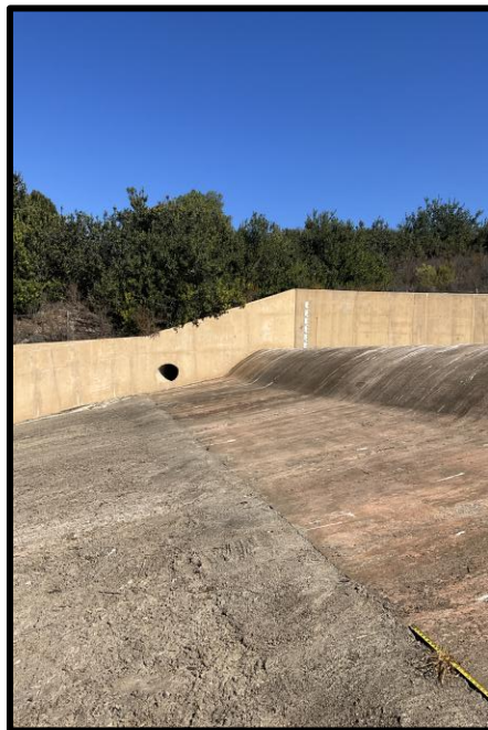
Photo 4) View of spillway ogee weir and unlined spillway channel transition looking northeast. Note 2' diameter corrugated metal pipe.
