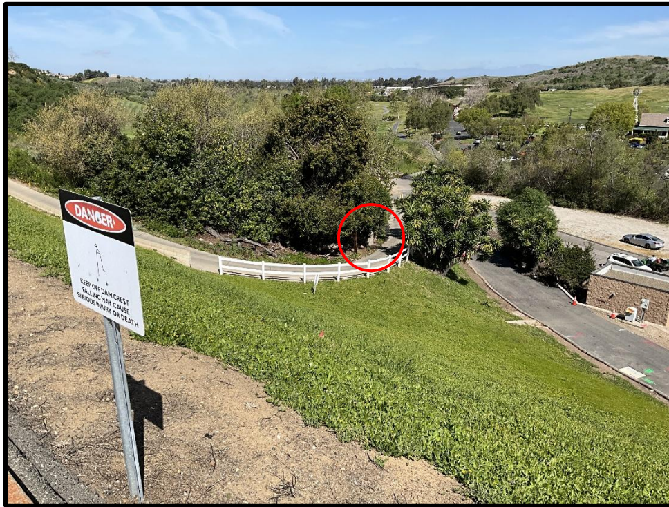
Photo 5) Downstream face of dam near left abutment. Note abandoned irrigation weir box.
