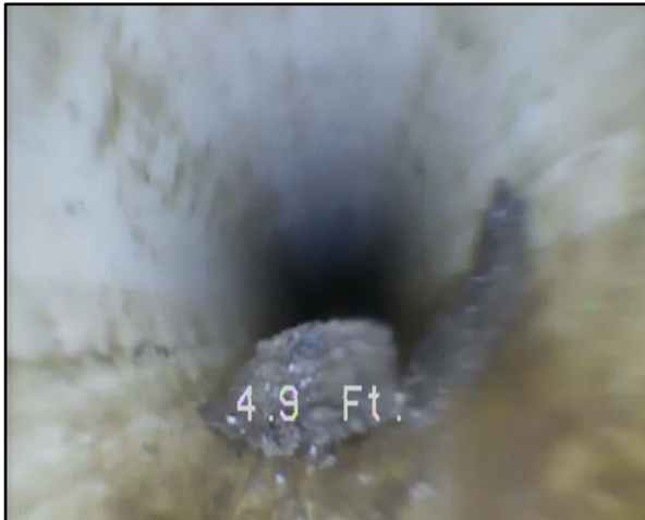
Photo 5 – STA 00+04: Debris in the pipe.
