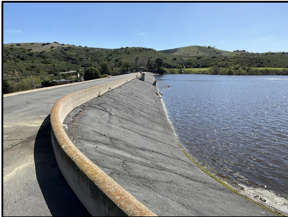
Photo 2) AC-lined upstream face looking towards right abutment. Note cracks along face.
