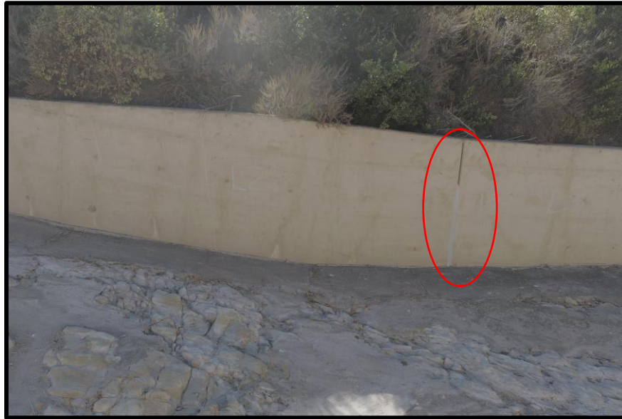
Photo 19) View of spillway wall panels L2 and L3. Note recently repaired wall joint.
