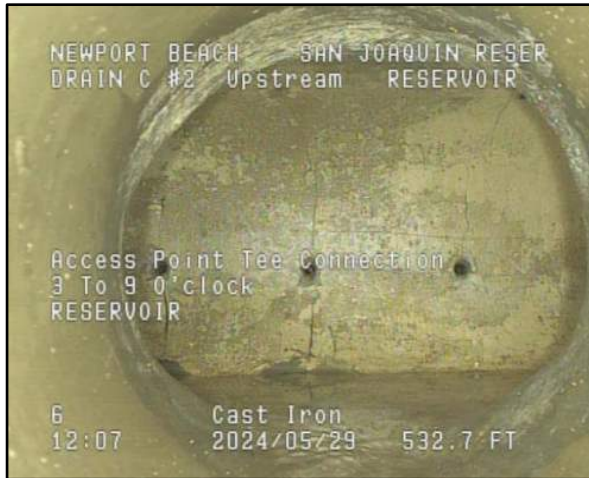
Photo 27 – STA 05+32: Tee connection and the end of the survey.
