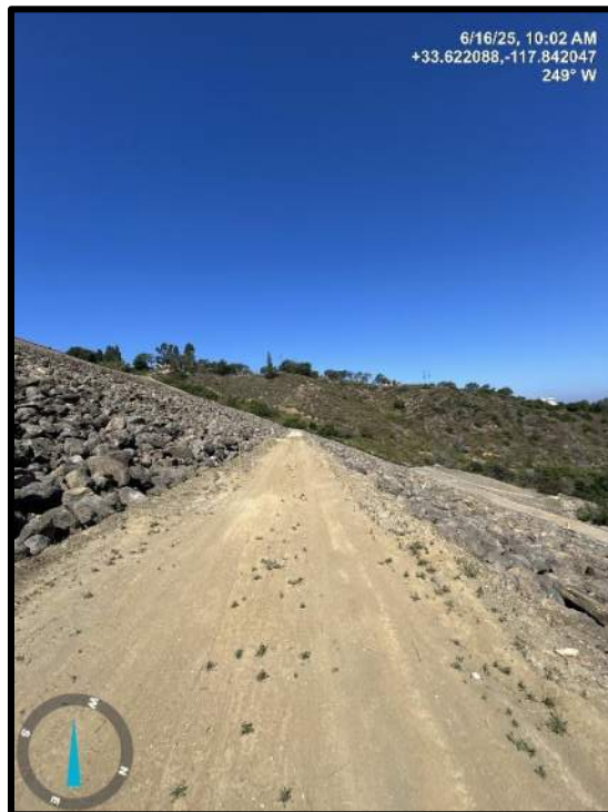
Photo 8) Downstream face looking towards left abutment from middle downstream bench.
