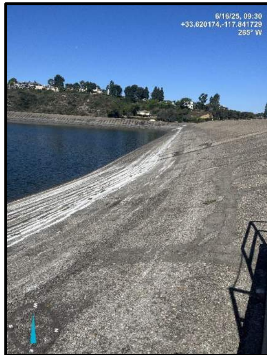
Photo 2) AC-lined upstream face looking towards left abutment.
