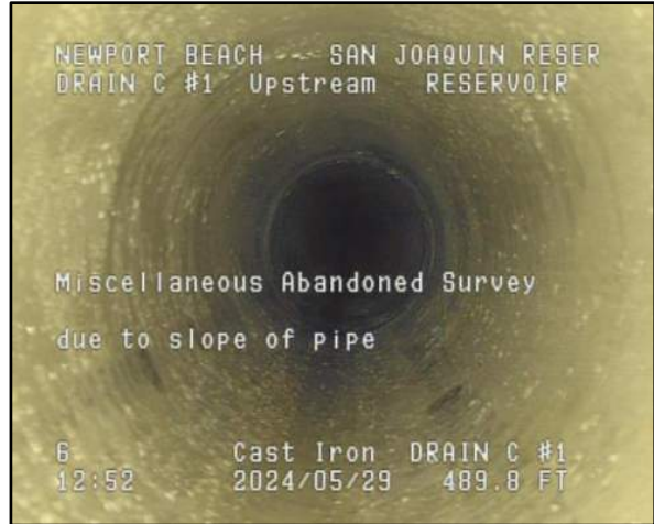
Photo 20 – STA 04+89: End of survey.
