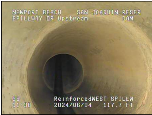
Photo 34 – STA 01+17: Pipe is in good condition (typical).
