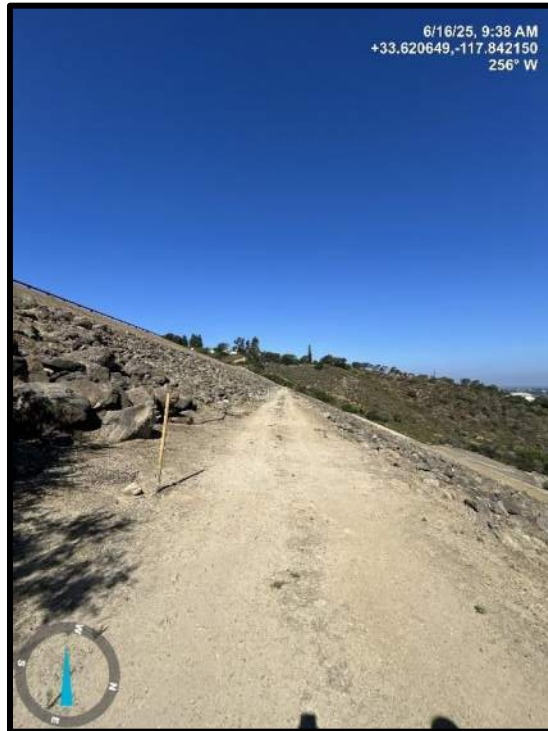
Photo 7) Downstream face looking towards left abutment from the top downstream bench.
