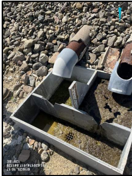
Photo 25) U/S Collector Drain #1 (left) and #2 (right). Note leakage underneath v-notch weirs.
