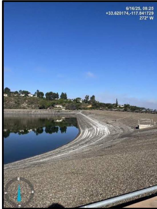
Photo 1) AC-lined upstream face looking towards left abutment.
