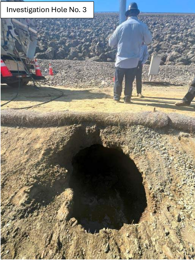
Inside of Investigation Hole No. 3
