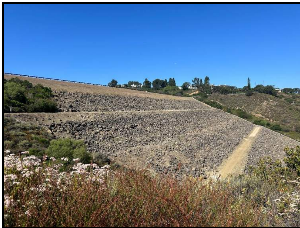
Photo 6) Downstream face looking towards left abutment.
