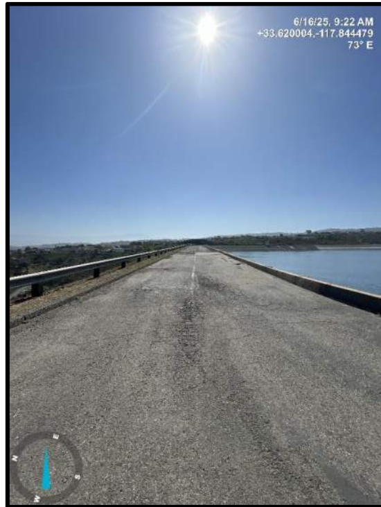
Photo 3) AC pavement on crest looking towards the right abutment.
