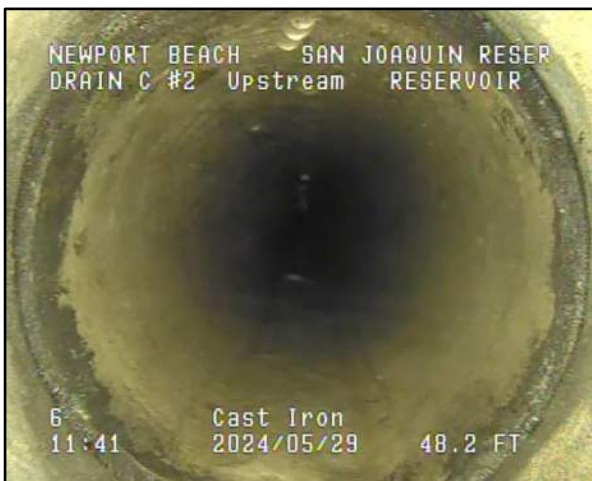
Photo 21 – STA 00+49: Pipe is in good condition (typical).
