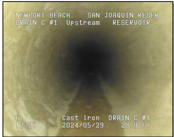
Photo 16 – STA 00+28: Pipe is in good condition
