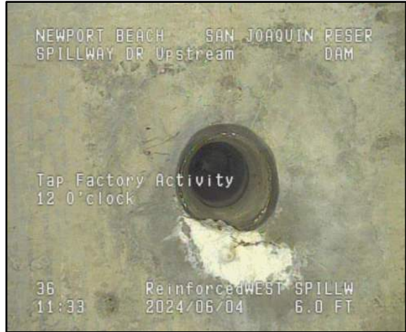
Photo 33 – STA 00+06: Tap into the pipe at 12 o'clock.
