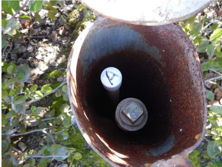
Photograph 5: View of Piezometers CP-3A & CP-3B.
