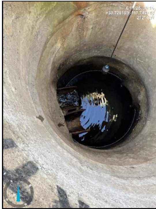
Photo 19) Seepage drain-pipe outfalls at the bottom of MH #1 downstream of dam.
