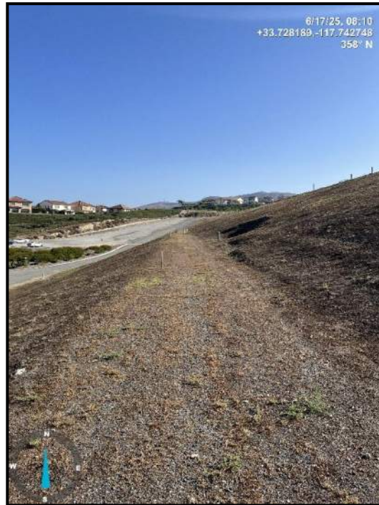
Photo 1) Downstream face looking towards right abutment from the middle bench.
