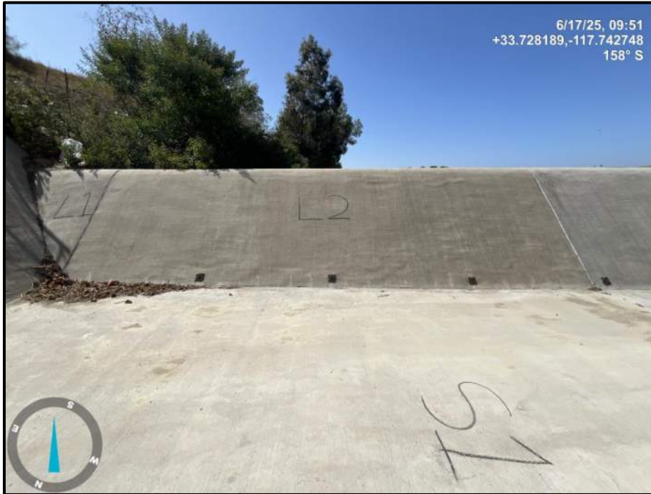
Photo 3) Wall panel L2. Note weep holes.
