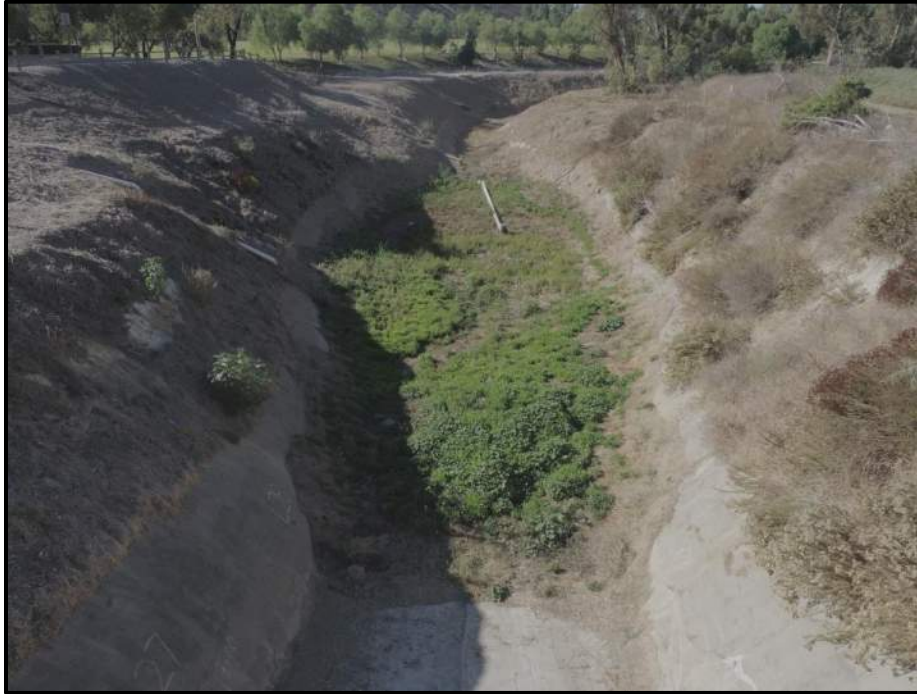
Photo 47) View of spillway stilling basing looking downstream. Note vegetation and sediment.
