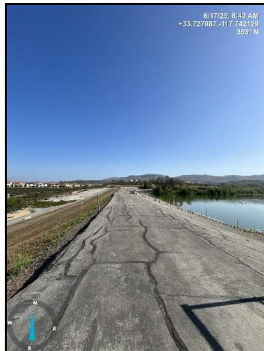
Photo 2) Dam crest, downstream face, and upstream face looking towards right abutment.
