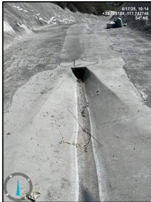
Photo 22) Existing 8” diameter spillway subdrain. Looking upstream.
