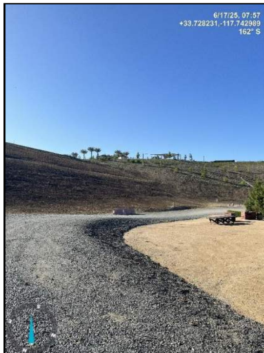
Photo 6) Downstream face as viewed from right abutment access road.
