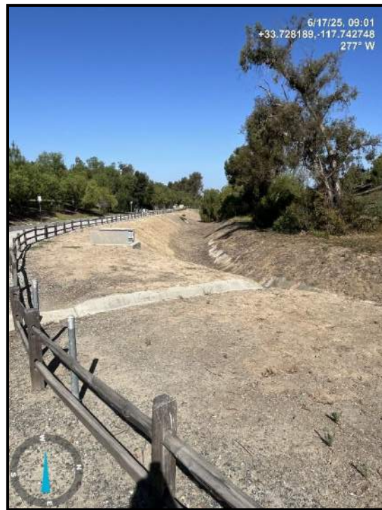
Photo 16) Downstream channel and seepage vault, looking downstream.
