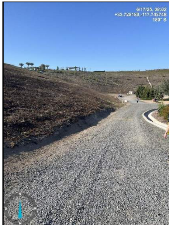
Photo 8) Downstream face and toe as viewed from right abutment access road.
