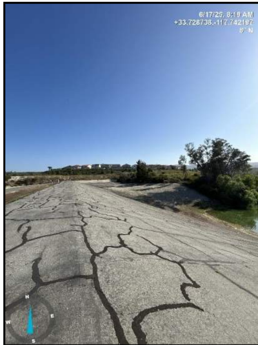
Photo 5) View of crest and upstream face of dam from the center of the dam.
