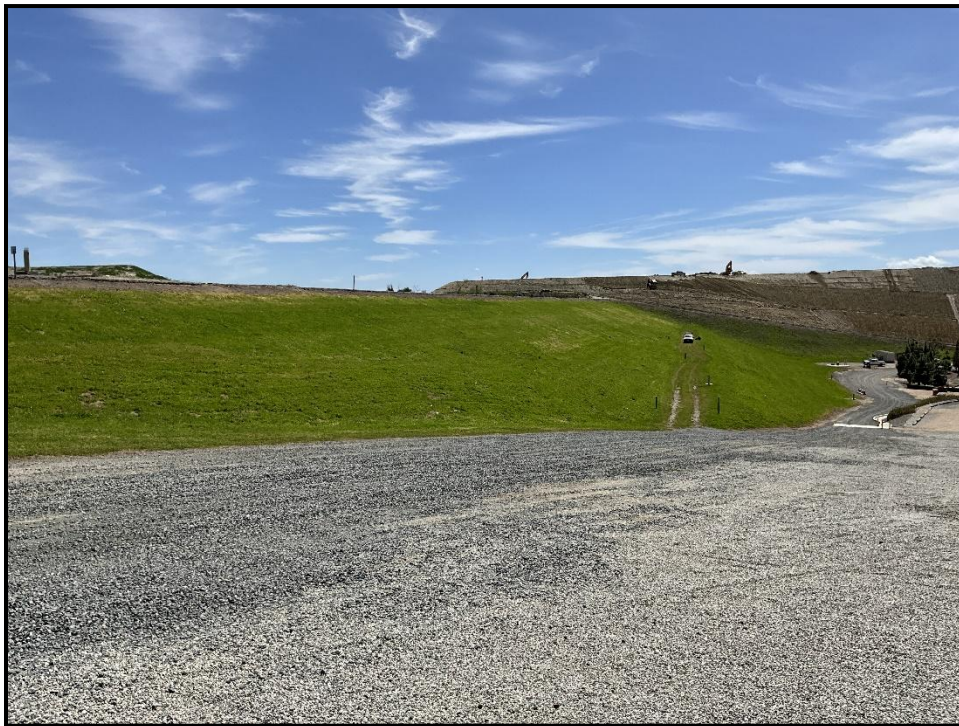
Photo 4) Downstream face and bench as viewed from right abutment access road.
