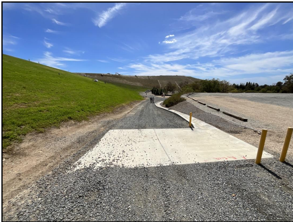
Photo 6) Downstream face and toe as viewed from right abutment access road.
