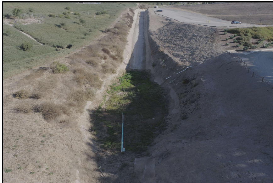
Photo 46) View of spillway stilling basin looking U/S. Note vegetation and sediment.
