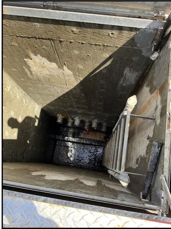
Photo 15) Seepage drain-pipe outfalls at the bottom of the seepage vault downstream of dam.
