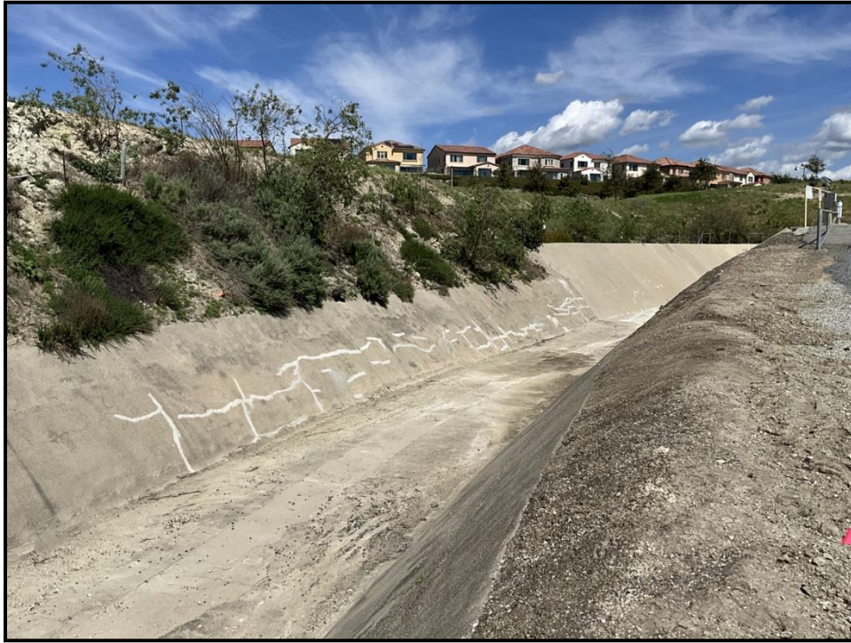
Photo 9) Spillway channel looking upstream. Note recent sealant repair on the right spillway wall.
