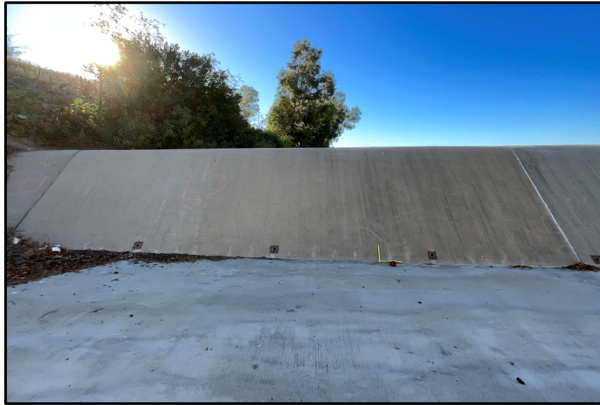
Photo 3) Wall panel L2. Note weep holes.
