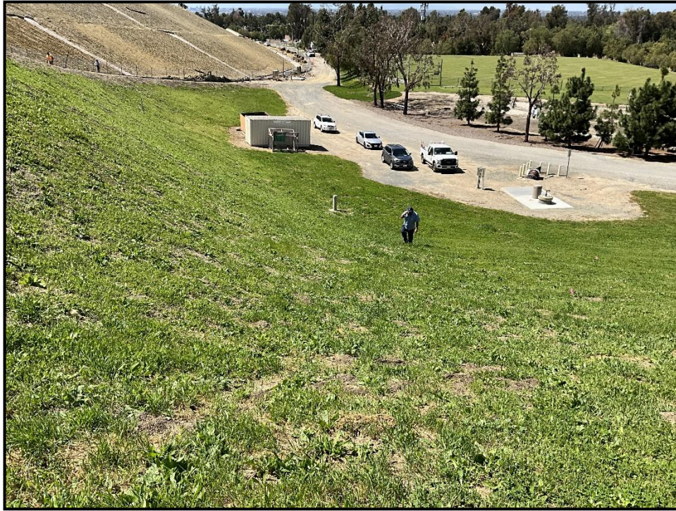
Photo 5) View along the left downstream face.
