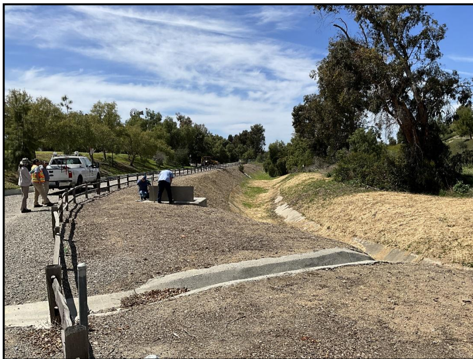
Photo 13) Spillway stilling basin looking downstream. Note trees and vegetation.
