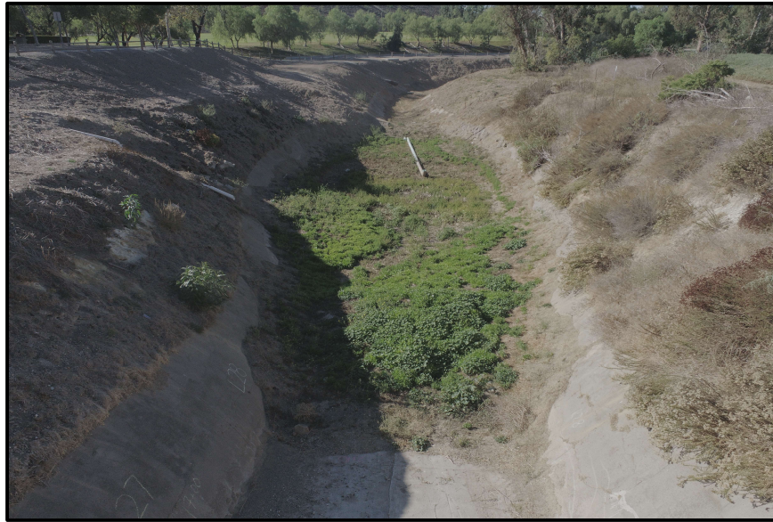
Photo 45) View of spillway stilling basing looking D/S. Note vegetation and sediment.
