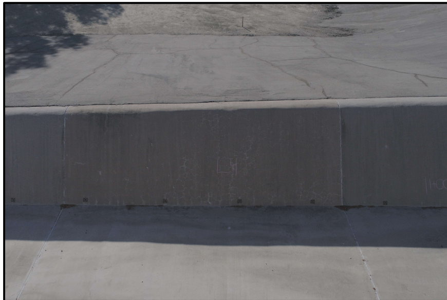
Photo 6) Wall panel L4.
