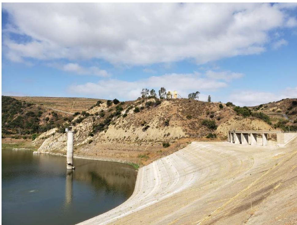
View of the outlet tower and spillway approach.
