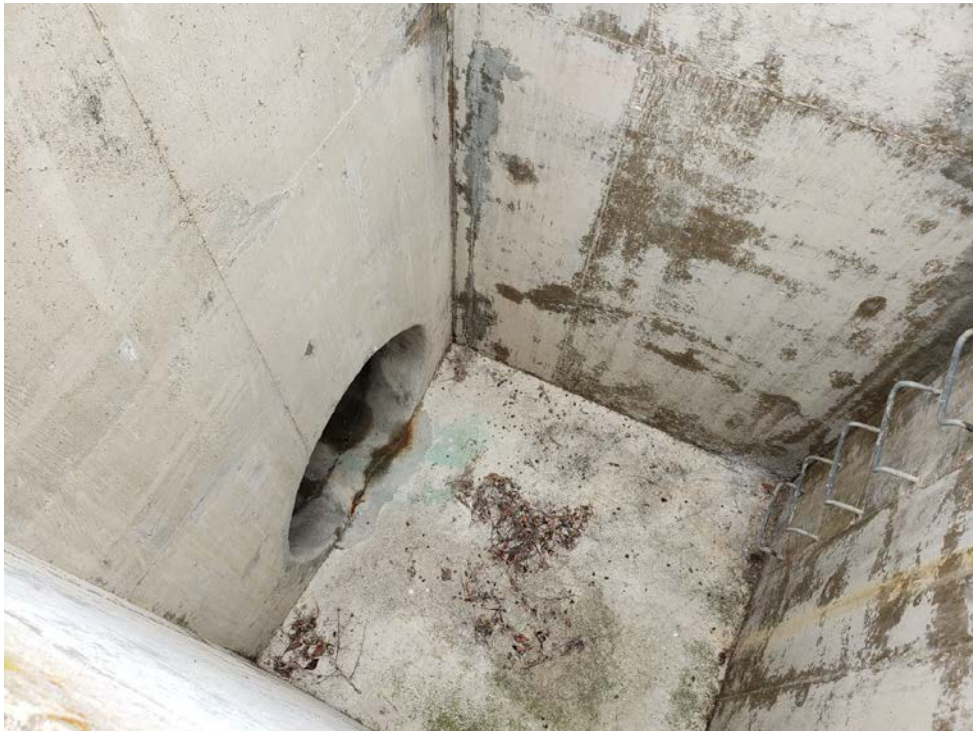
View looking in one of the drop inlet spillways.
