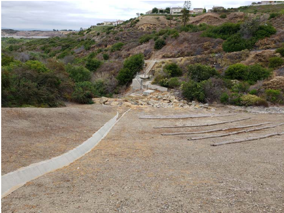
The lower downstream slope area.
