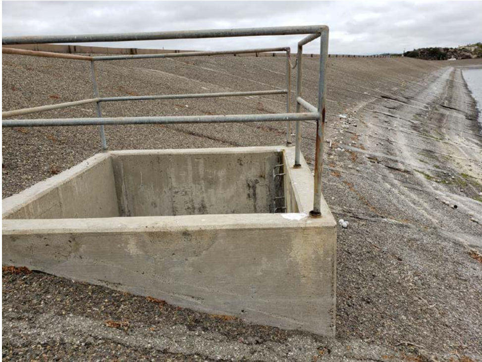
The approach to the two spillways were open and clear.
