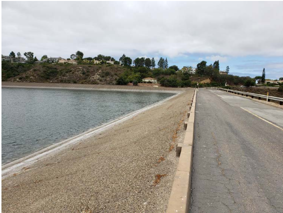
View of the crest and upstream slope.
