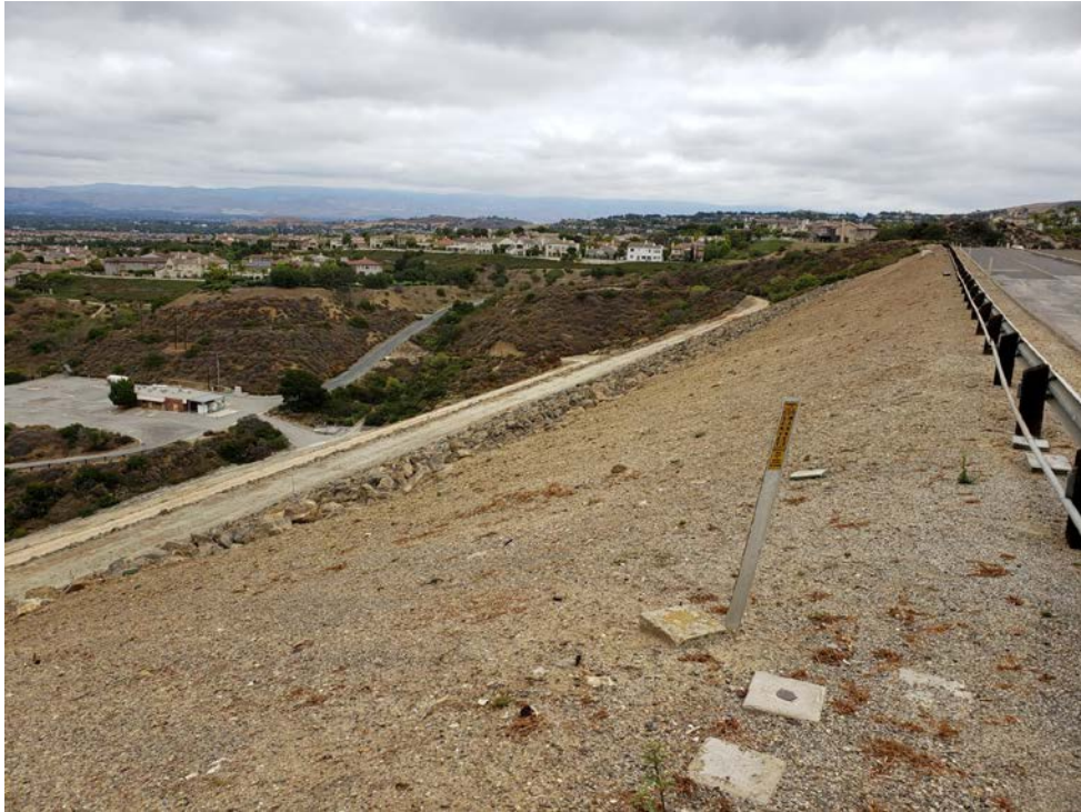
The upper downstream slope.
