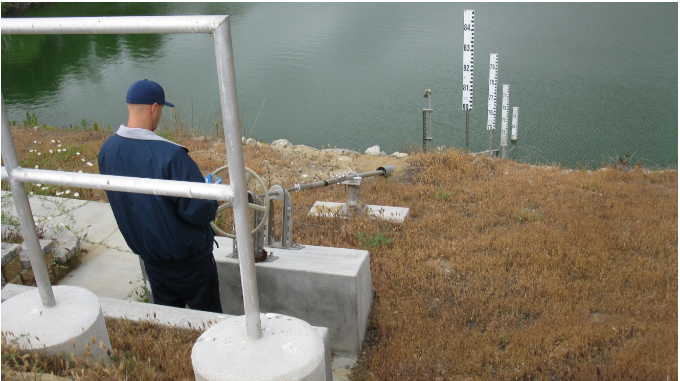
Outlet Valve Operation
