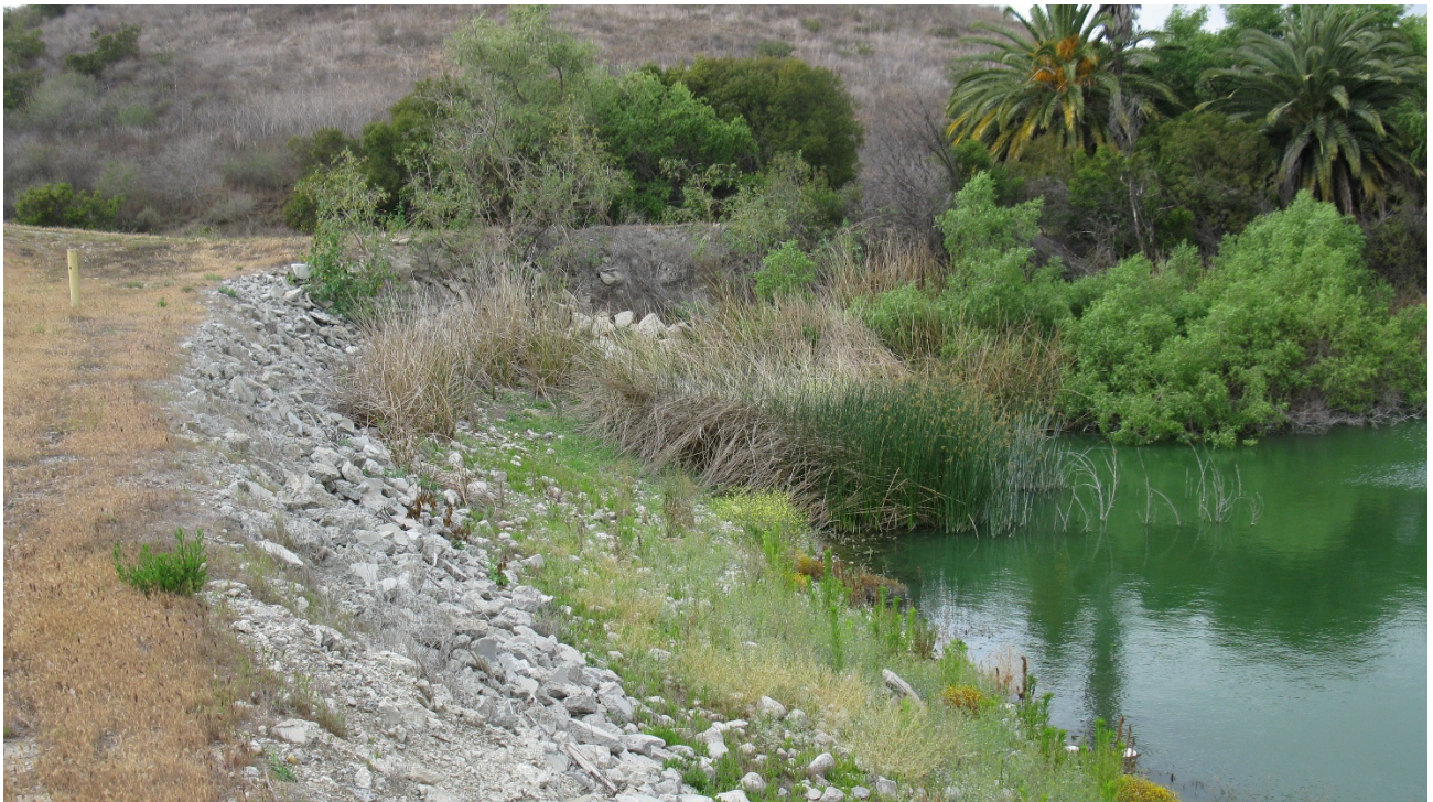
Vegetation on Right Upstream Groin must be cleared to permit inspection
