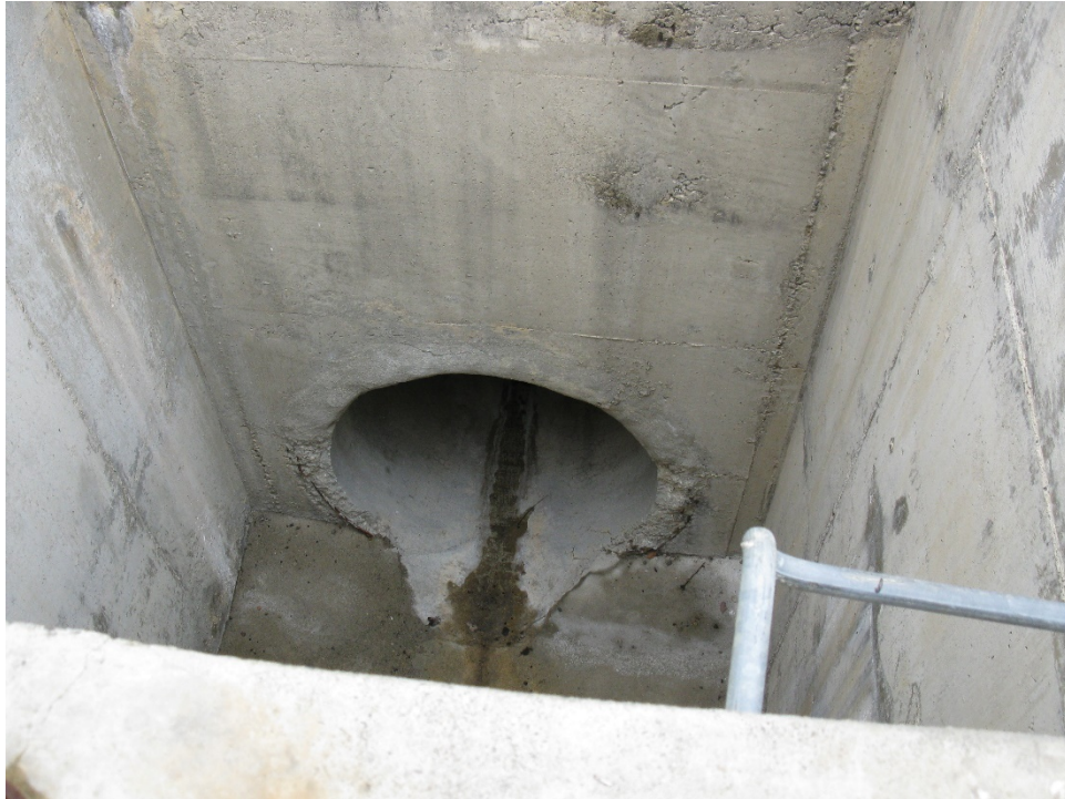
Entrance to 48" RCP at Bottom of Right Drop Box Inlet Spillway
