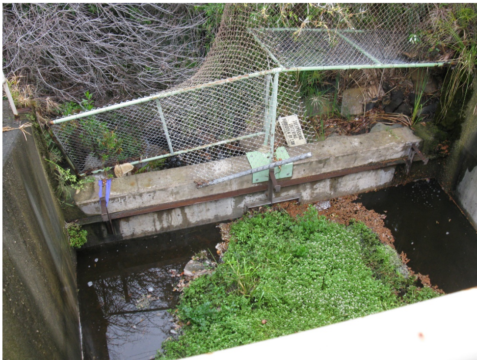
Spillway Impact Dissipater (Exit) Structure
