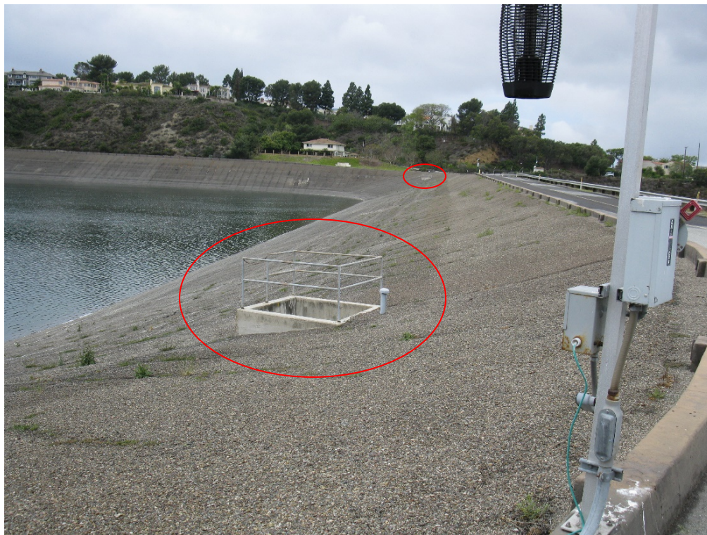
(2) – Drop Box Inlet Spillways
