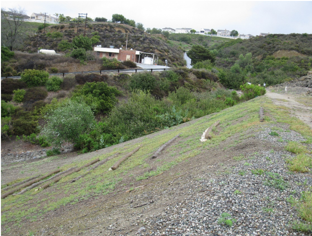
Grove of woody vegetation near the downstream toe near the Right Abutment (should be cleared)
