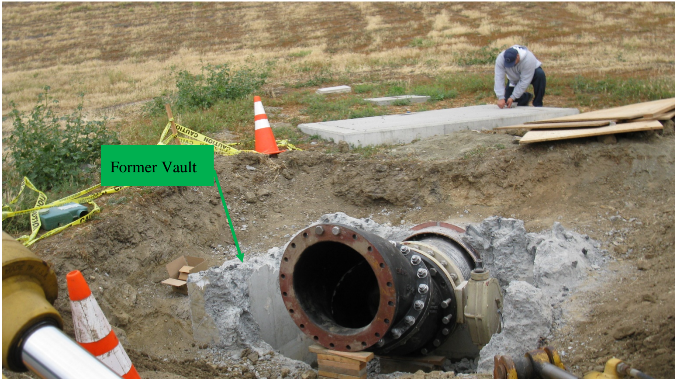
New Outlet Works in progress at downstream vault
