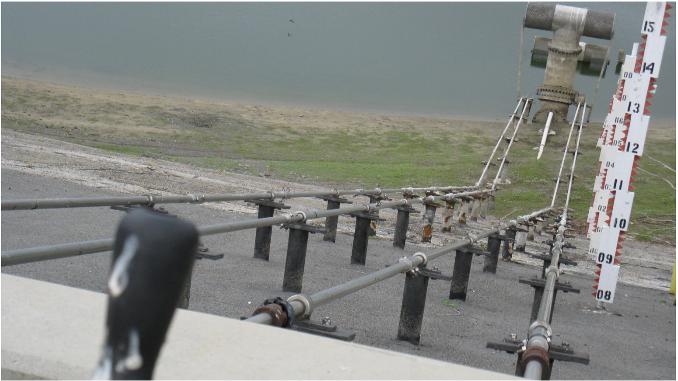
Upstream Valve Controls – High inherent friction made operating the valves very difficult
