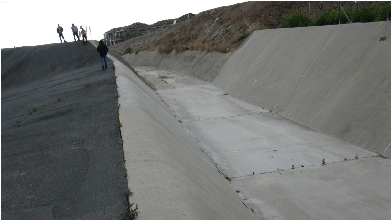
Spillway Approach and Side Channel Drop Inlet
