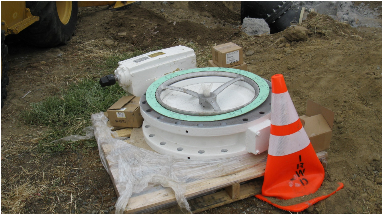
New Valve and Actuator
