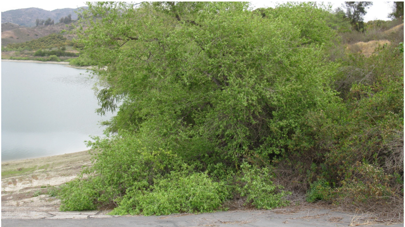
Trees and Woody Vegetation on Left Upstream Groin must be removed.
