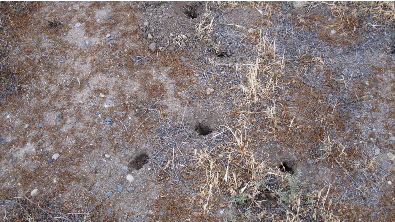
Rodent Activity on left side of Spillway Channel
