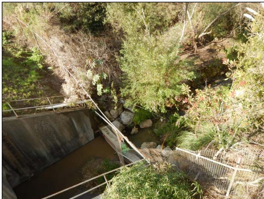
**Photo 3. View of heavy vegetation growth immediately downstream of the energy dissipator.**
