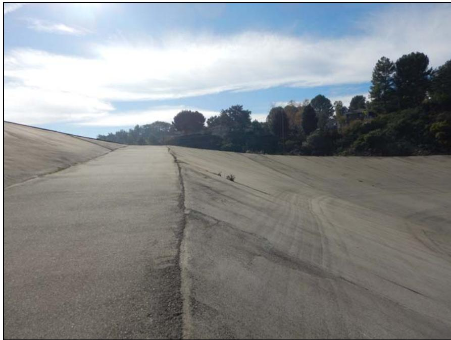
**Photo 4. View of vegetation growth along joints near the reservoir access ramp.**
