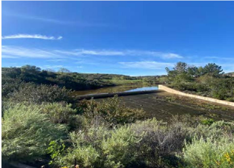
Figure 37. Overview of Ridge Valley C in November, 2024.
