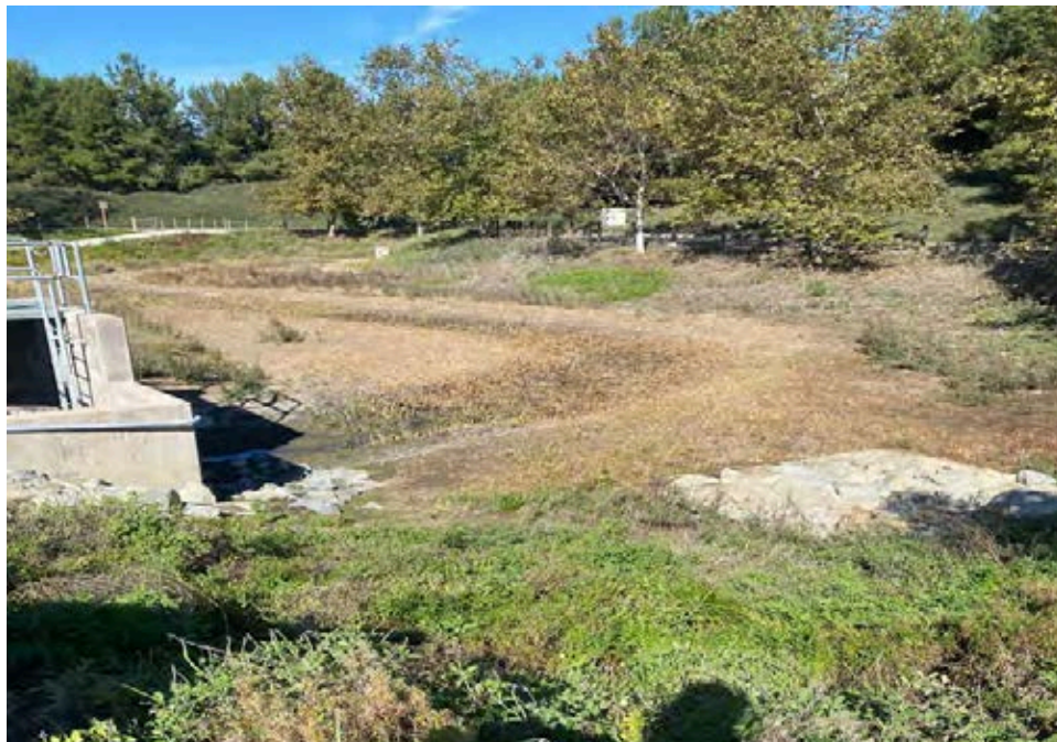
Figure 26. Laguna Altura South as of November 2024.
