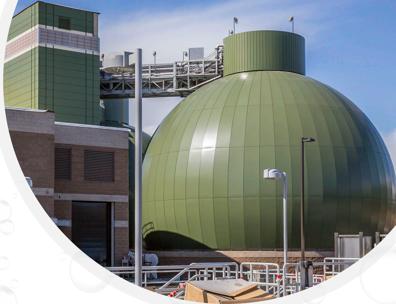
MWRP Biosolids Facility
