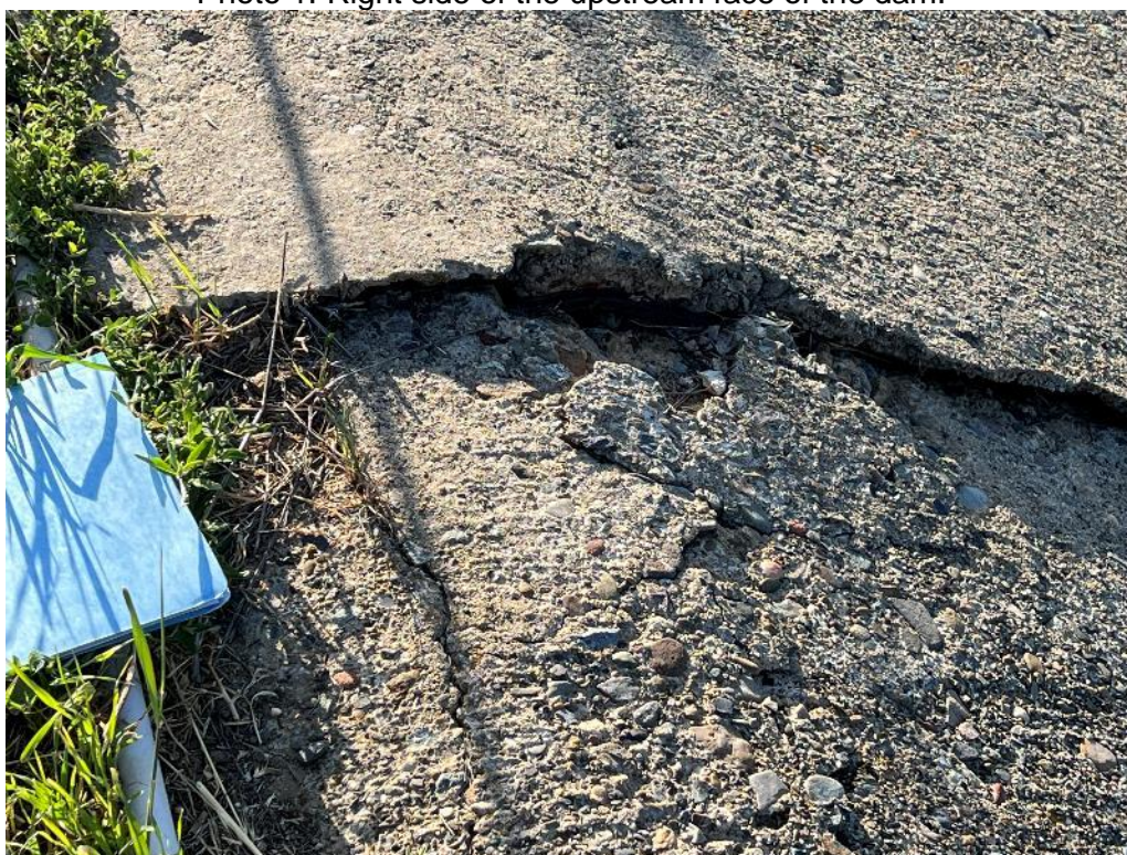
Photo 2. Crack in the upstream concrete liner.
