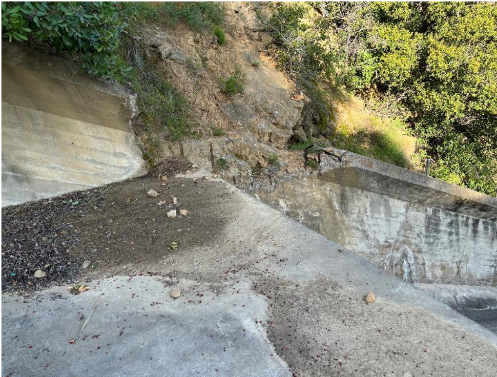
Photo 9. Missing section of concrete at the downstream end of the spillway chute and flip bucket.
