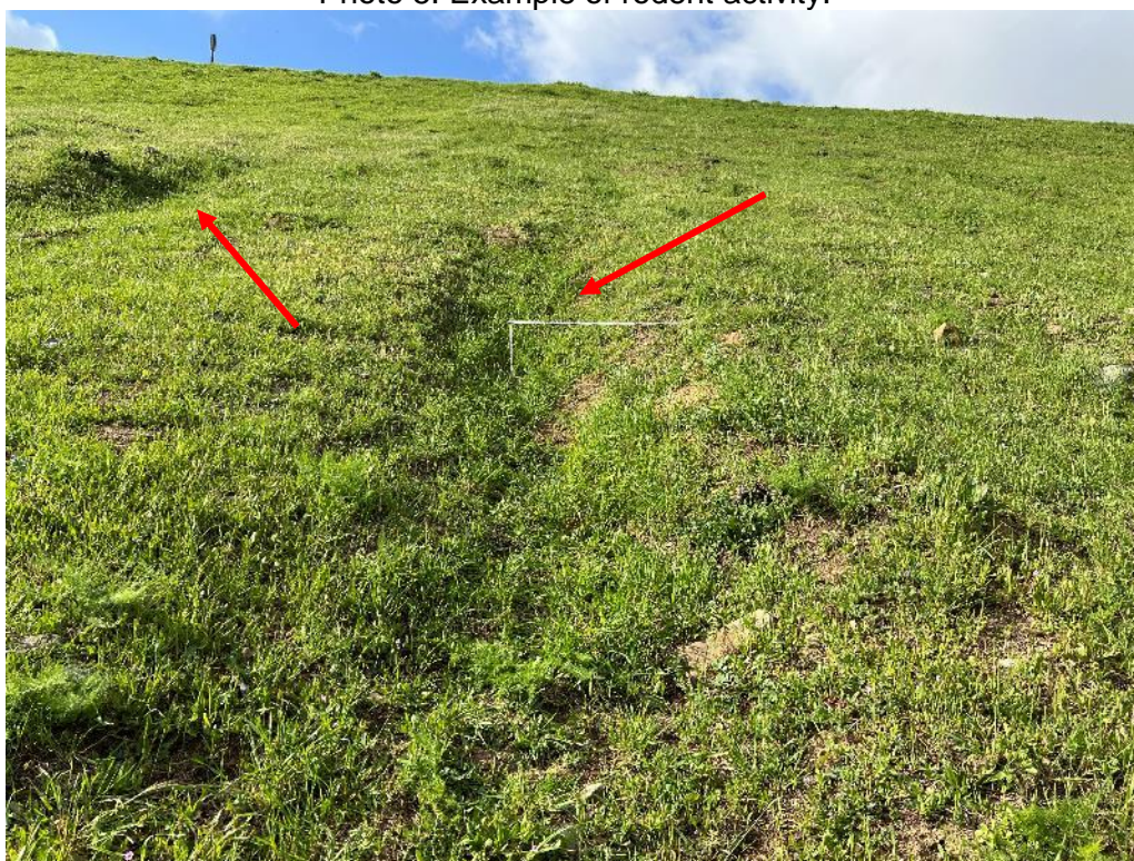
Photo 6. Example of erosion rills on the downstream face of the dam.
