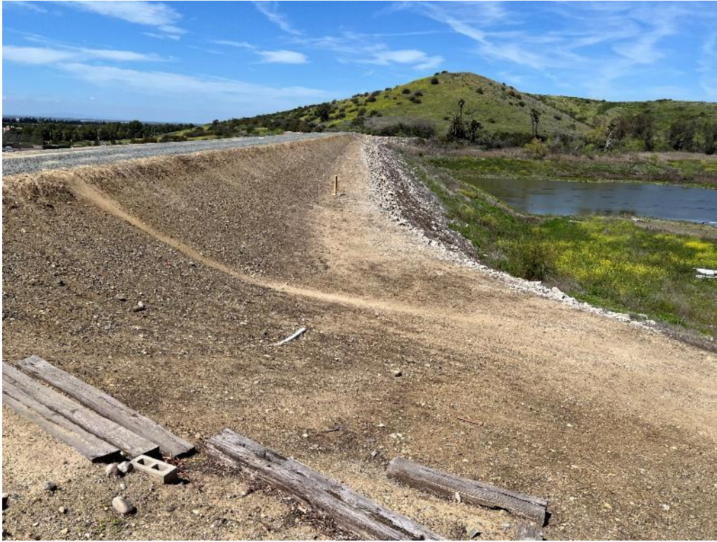
Photo 2. Upstream face of the dam.
