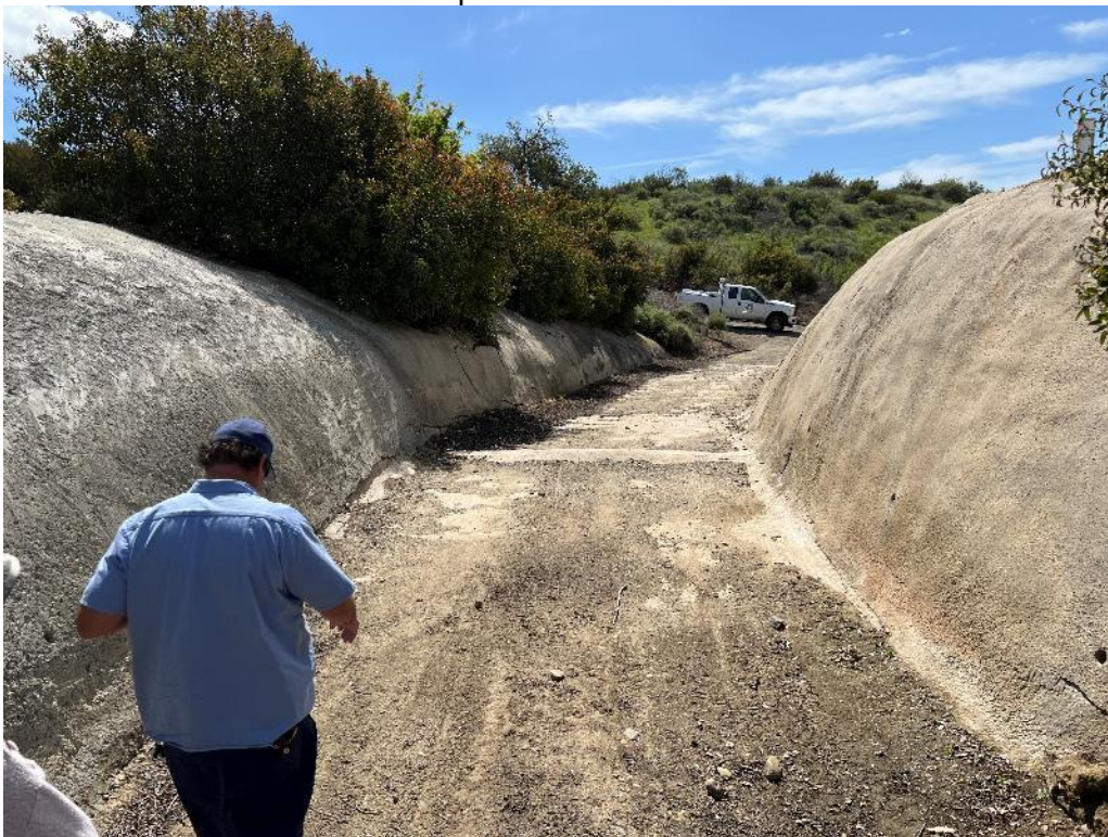
Photo 3. Spillway control section and downstream channel.
