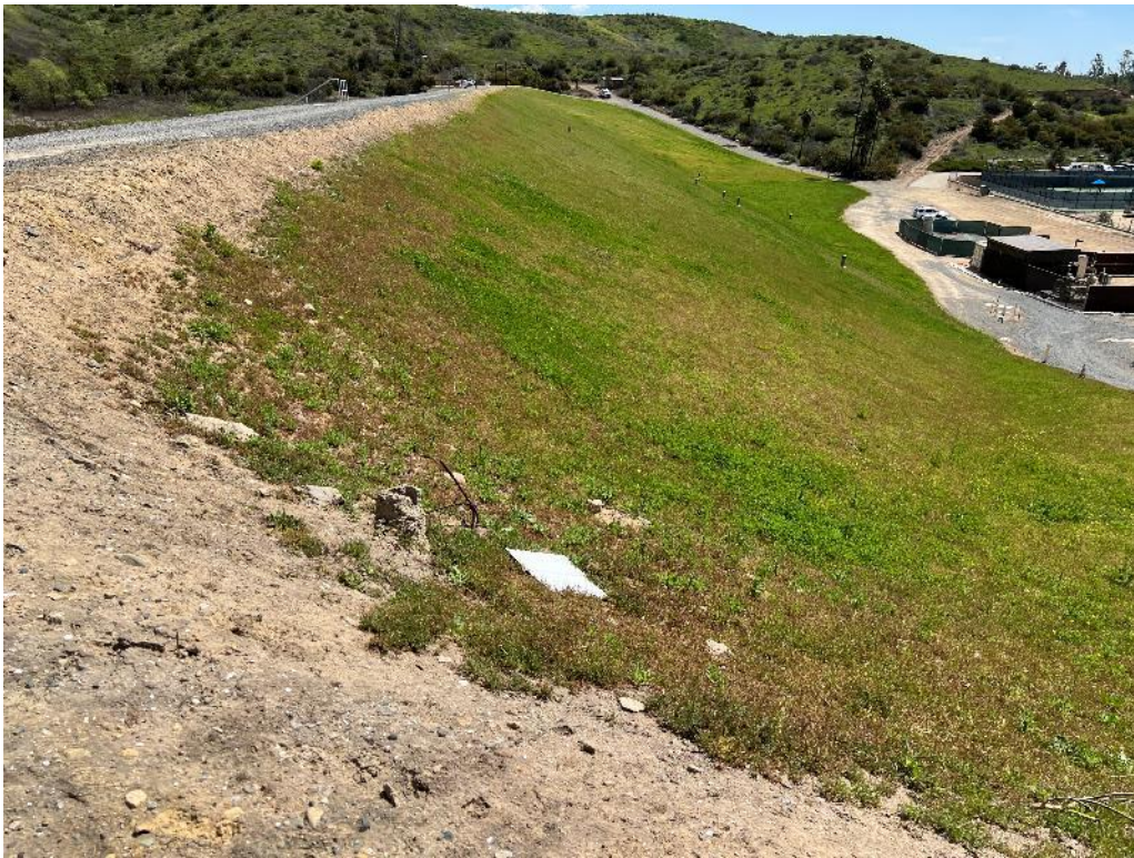
Photo 1. Downstream face of the dam.
