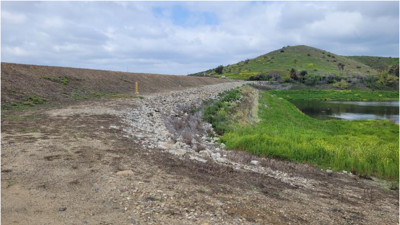
Photo 3: View of the upstream slope from the left abutment.
