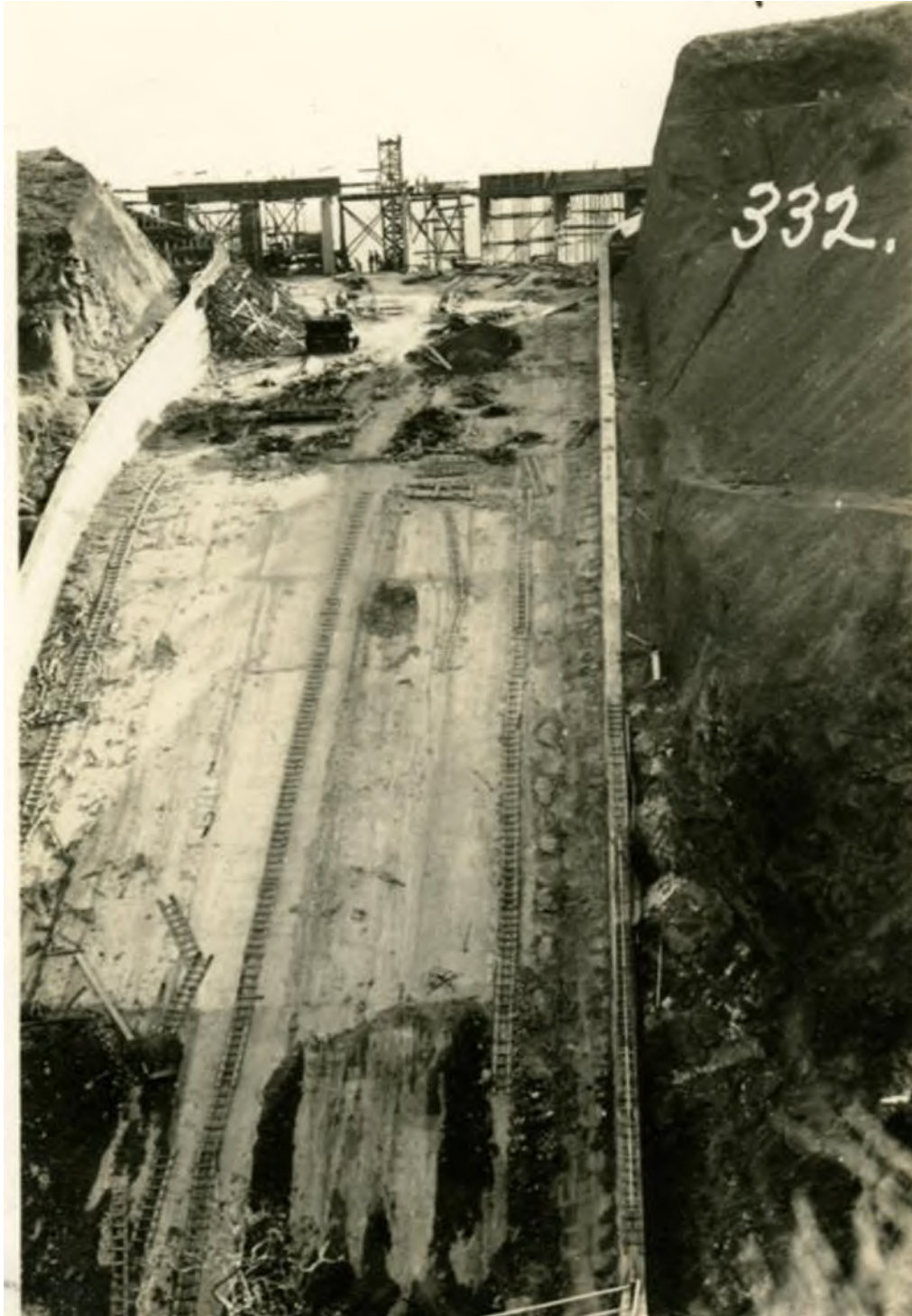
Exhibit 16: Spillway crest and chute under construction circa 1931 (Courtesy of IRWD)
