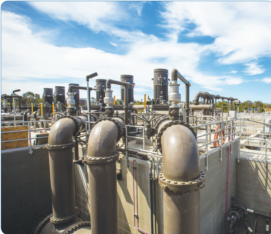
Pumps and pipes for the membrane bioreactor at the expanded Michelson Water Recycling Plant.
