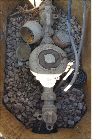
New Residential Meter
