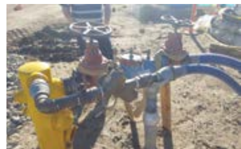
Another meter with backflow assembly
