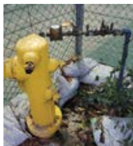
Meter with backflow assembly
