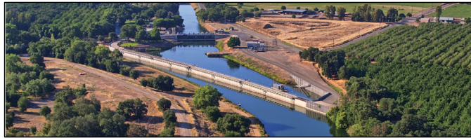
GCID Main Canal Pumping Plant use to divert Sites water
