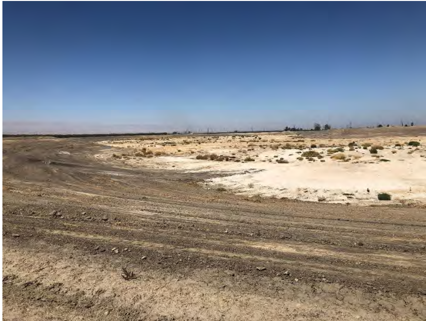
Photo 6: View of Buena Vista Water Storage District Daly Ranch recharge facility showing deepened basins to expose sandy material (lighter colored sediments in the center right of the picture).
