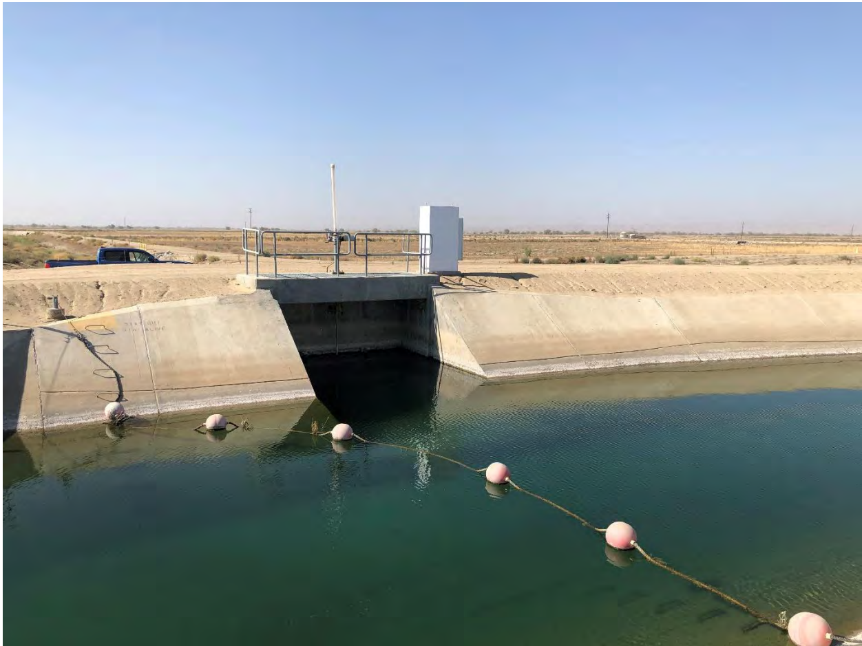
Photo 1: Cross Valley Canal outlet to South Strand feeder canal.
