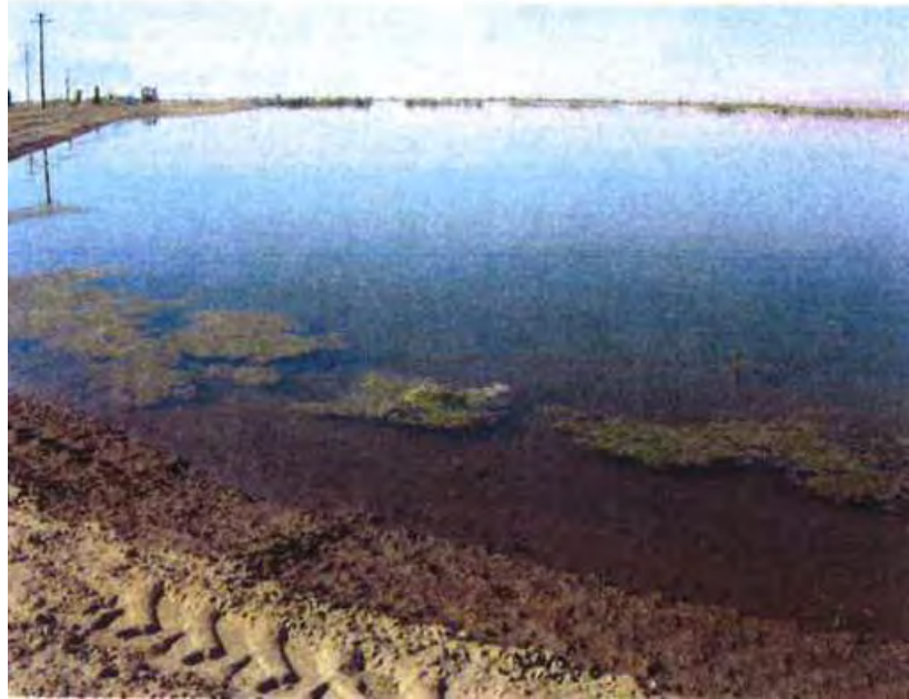
Photo 5: Strand Ranch basin during full condition showing algae buildup in surface water. (Photo from HDR, 2009).
