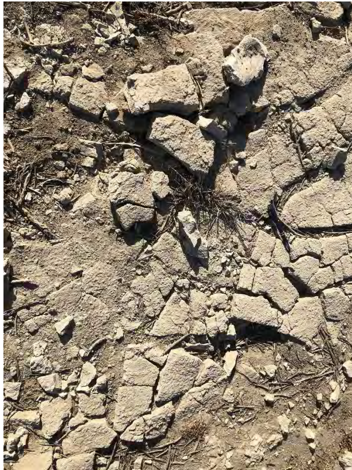
Photo 2: Fine-grained buildup on the bottom of the South Strand feeder canal. The fines become cracked and breakup during dry periods but likely go into solution when water is released from the CVC.
