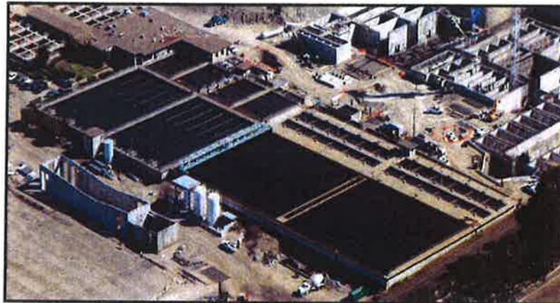
Figure 5-1: Typical Flocculation-Sedimentation Basins
