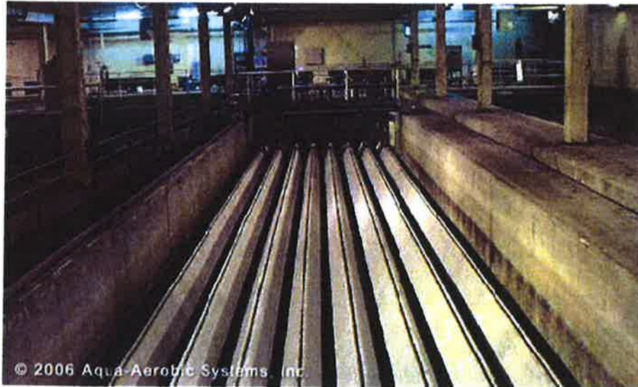
Figure 5-6: AquaDiamond Cloth Filter Installation
