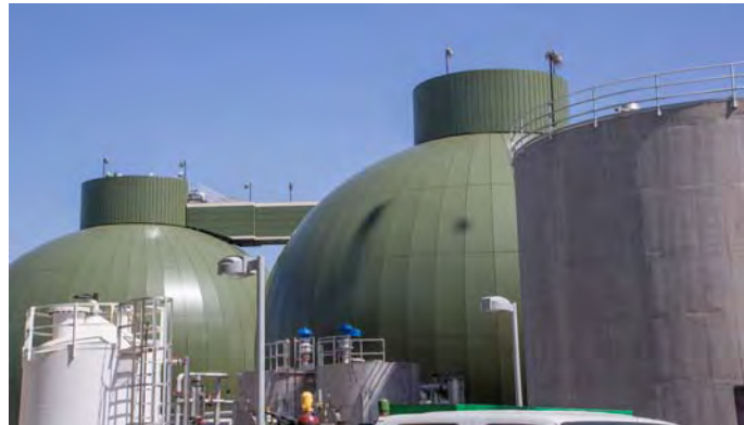
Biosolids and Energy Recovery Facilities Project
