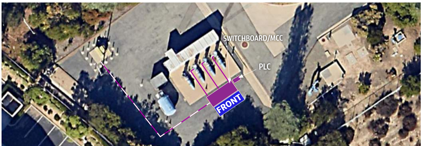
Figure 2.3 - location of pad mounted temporary power equipment and above grade pump feeders
