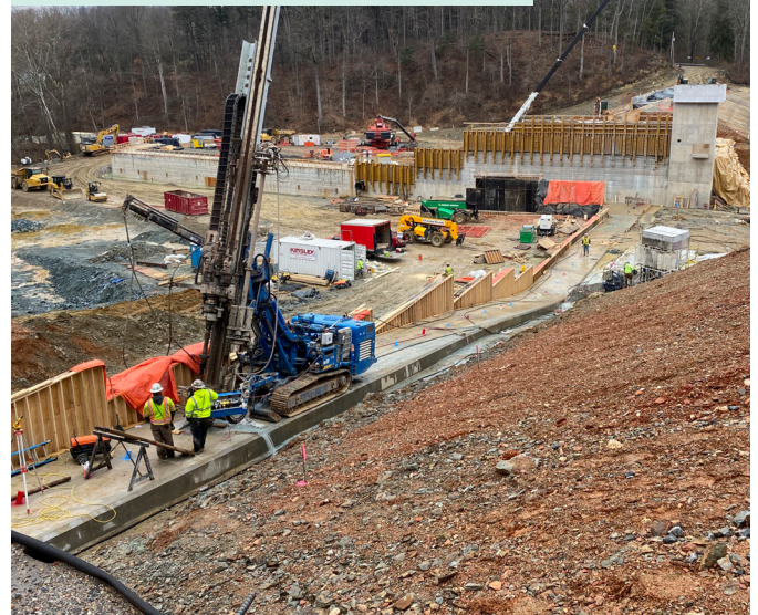
Lake Williams Dam Rehabilitation
