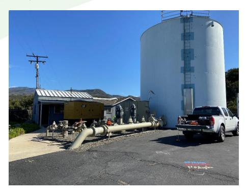
IRWD provides potable water supply service to the Santiago Area located in an unincorporated region of Orange County. This service area includes four distinct sub-areas containing a system of reservoirs and pump stations that solely rely on the existing 150,000-gallon steel Zone 8 Fleming storage reservoir and the existing Zone 8 to 9 booster pump station as the main source of water supply.
