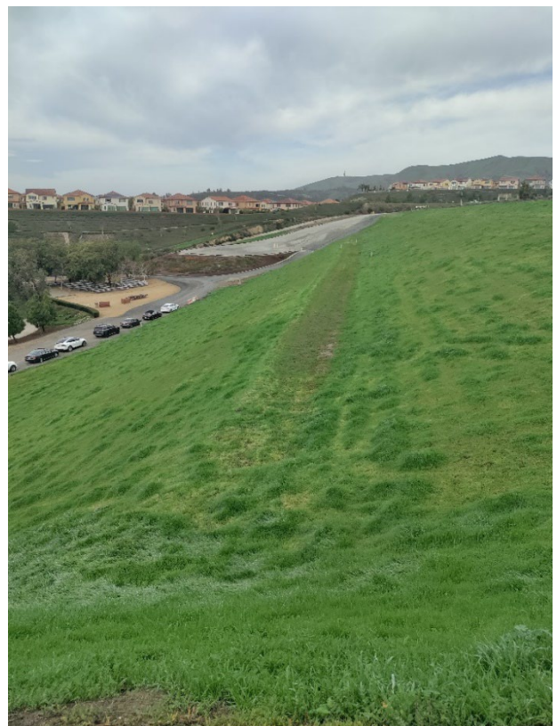
Downstream slope of Rattlesnake Dam showing the intermediate bench where the two sonic borings will be drilled from.
