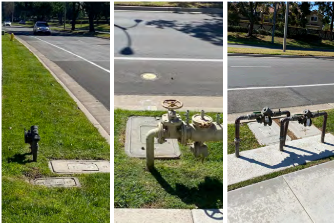
Irrigation Water Meters
